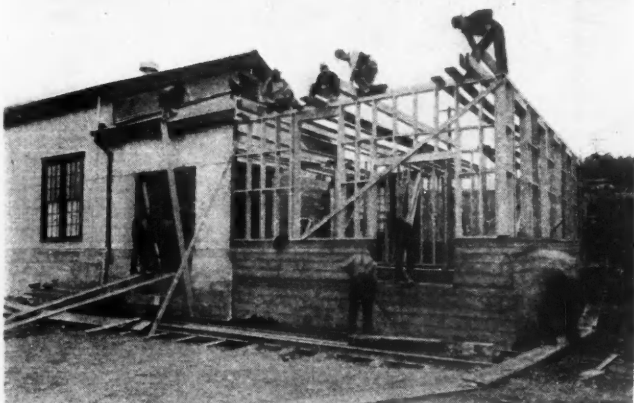
Carpenters at work on a building job at Puget Sound, part of the Federal $3,300,000,000 Public Works program
