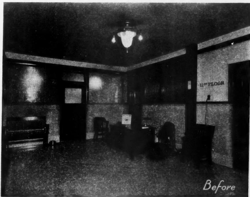
To left: Typical of hundreds of thousands of old style offices, this Minneapolis reception room invited complete rebuilding in which flat bands of hardboard took the place of marble and glass, and acoustical tile covered the hard plaster ceiling
