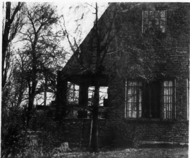
VIEW OF SHAFFER HOUSE as new addition nears completion. Cost of work was 60 per cent less than a 1931 estimate
