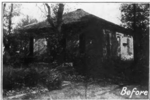
HERE IS THE PHOTOGRAPHER'S PICTURE OF THE HOUSE AT 105 N. CASS AVENUE AS IT APPEARED BEFORE CONTRACTOR HUGHES STARTED MODERNIZATION WORK.
