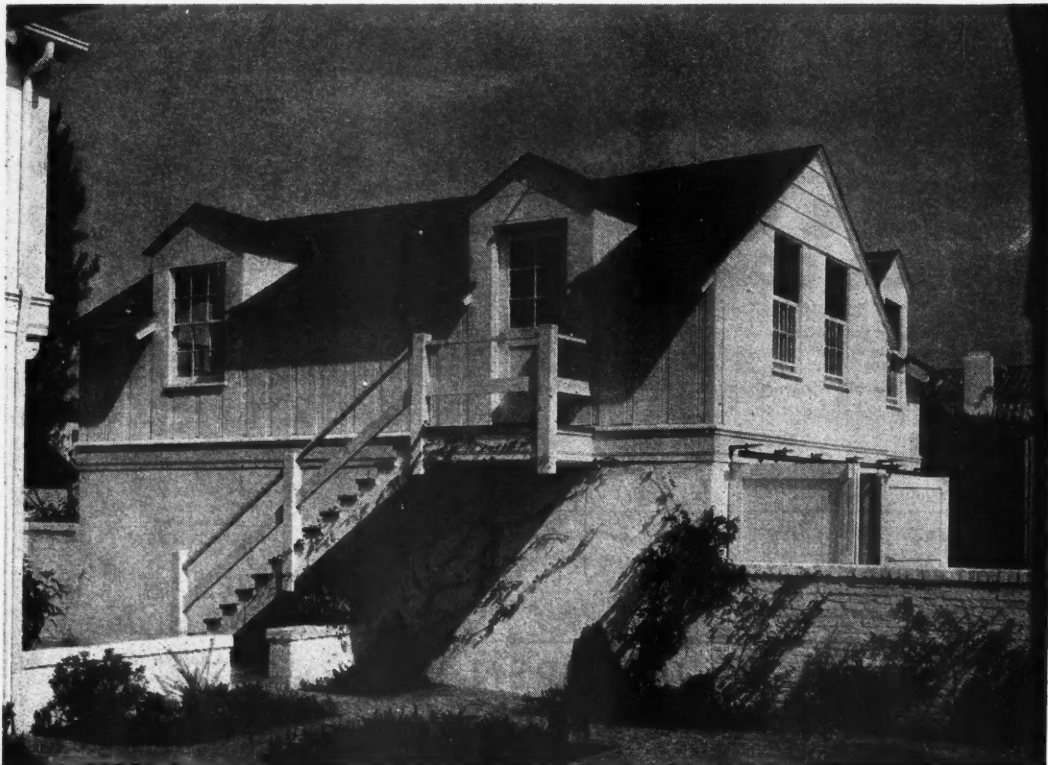
This attractive Los Angeles garage designed by Architect Paul R. Williams illustrates how quality can be carried out in garage construction in a simple, effective way. The brick wall at right blends well with the white stucco first floor exterior. Vertical boards of unusual width are used above the first floor.
