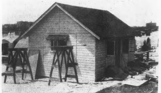
On the smaller houses, the panel construction is left visible as a feature on the outside design. On the larger models no panel lines are seen, being cleverly covered by the construction. Photos show process of setting up 2-room Pullman at Fair.
