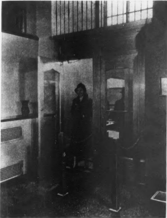
MAGIC DOOR which opens on approach of a person. A photo-electric control, door operator, and an air compressor make up the mechanism. Interception of a ray of light shining on a photo-electric cell opens the door, and it closes automatically—The Stanley Works.
