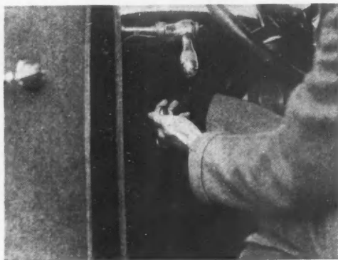
RADIO CONTROL at left automatically opens the garage doors. Code signal is sent from transmitter in car when approaching garage. A pull on lever by driver opens doors—Barber-Colman Co.
