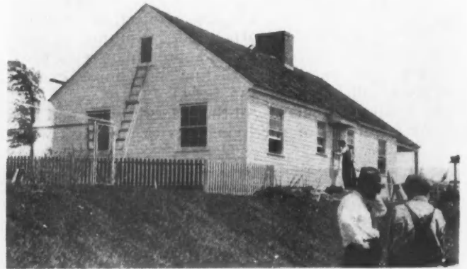
Progress views showing assembly of Crossett 5-room (Cape Cod model) home at Century of Progress. Factory-built panels for walls, partitions, floor and roof interlock and are bolted or nailed together.
