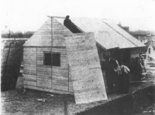
On the smaller houses, the panel construction is left visible as a feature on the outside design. On the larger models no panel lines are seen, being cleverly covered by the construction. Photos show process of setting up 2-room Pullman at Fair.
