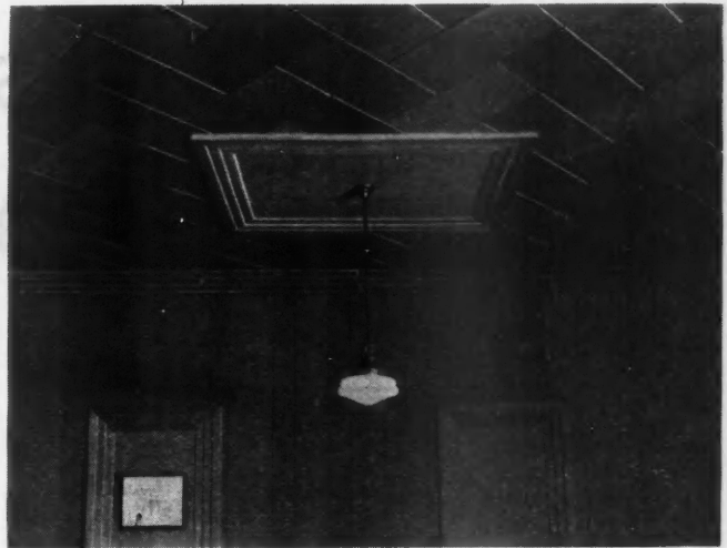
Attractive installation of new wood tile, which insulates and gives acoustical correction.
