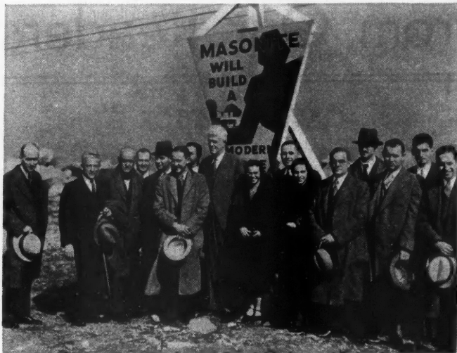
Dedicating the prize winning Masonite house as construction started on the World's Fair grounds at Chicago was quite an event, as the picture shows. Present above were Eugene Klaber, W. H. Mason, R. G. Wallace, Col. Robert Isham Randolph, H. B. Watkins.
