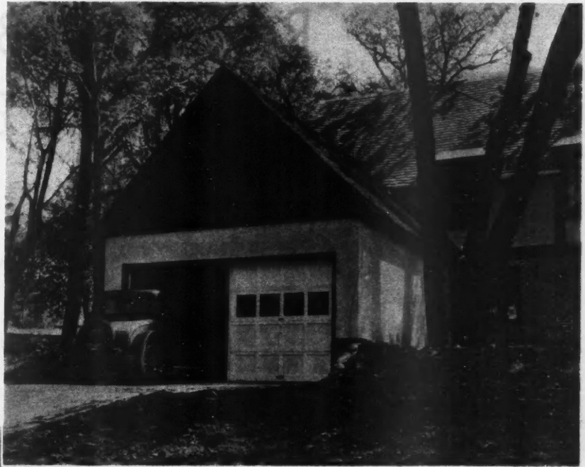
Stucco and stained siding are used to good advantage in the garage above. Below is another attractive design equipped with automatic door control.
