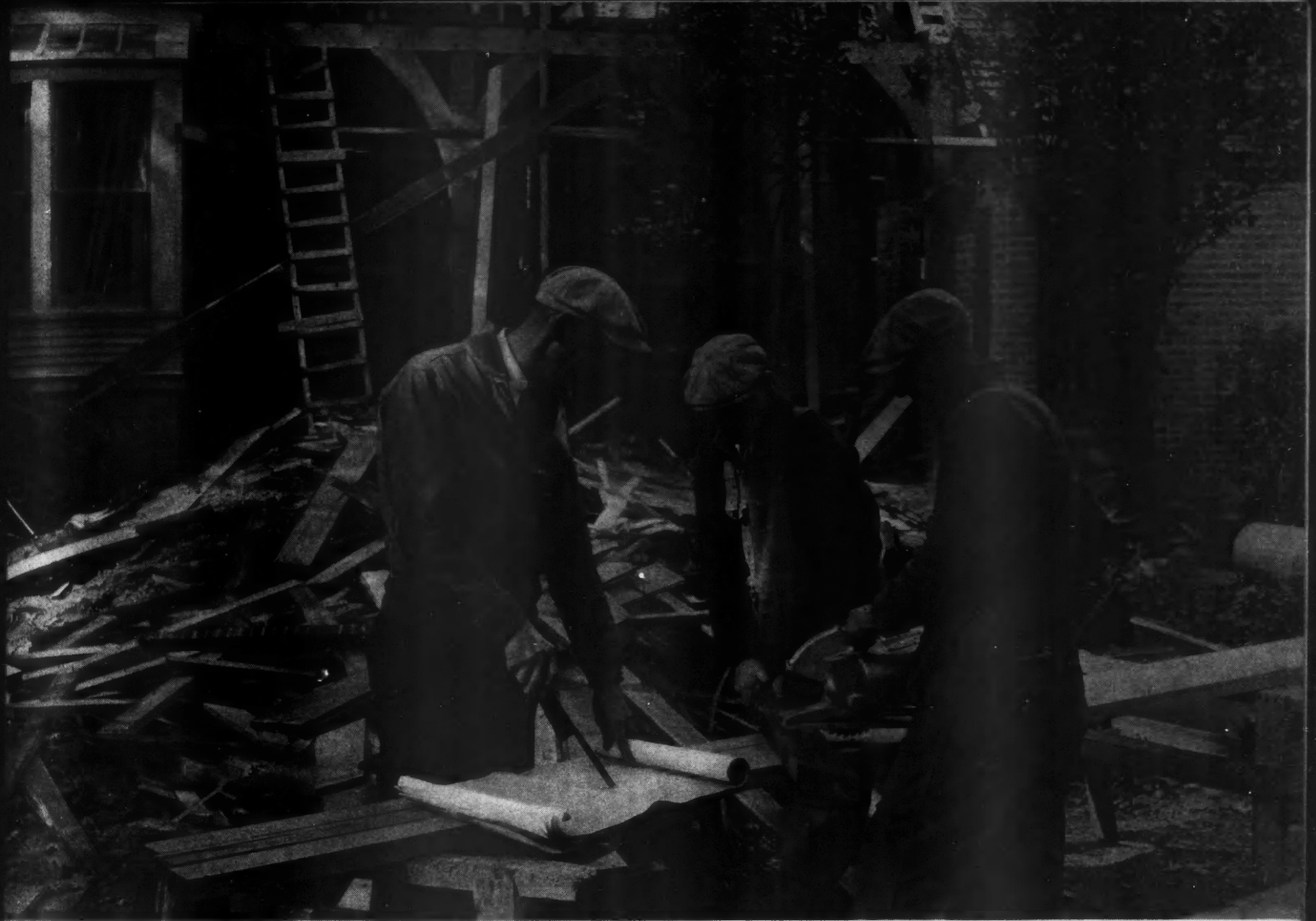
On this Highland Park, Ill., modernizing job thousands of feet of lumber were reclaimed through use of the power saw. W. J. Brown, the contractor is shown at left giving instructions to operator.
