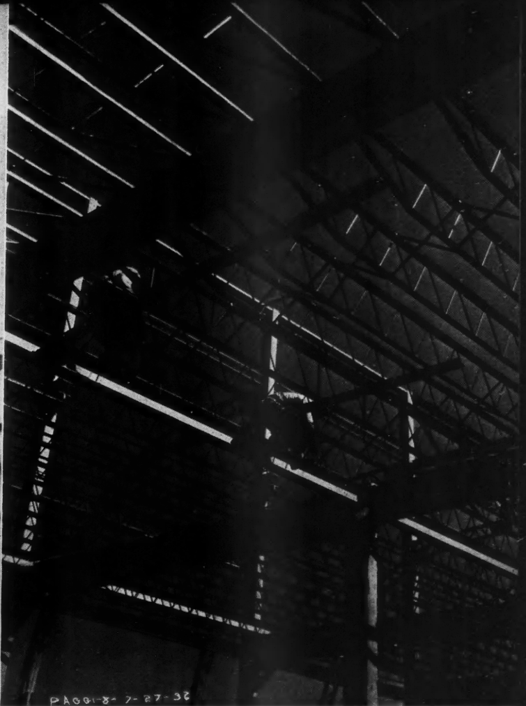
4—Agricultural Building, showing typical steel framing used on various exposition buildings.
