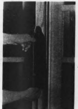
Exterior and details of new double hung window which has improved weight and frame permitting inside casing as narrow as 2 1/4 inches.
