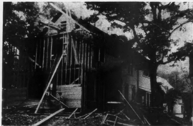
Front view showing addition of big living room. The old lumber in foreground was all to be reclaimed through use of power saw. New two car garage can be seen at rear.
