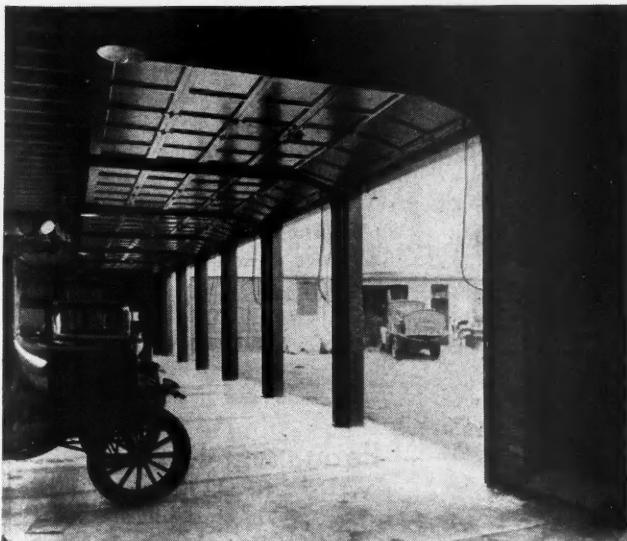
Here Is a Spring Balanced, Upward Acting Door Which Has Been Designed for Private Garages and Service Stations.
