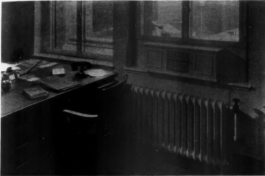
A Neat Metal Box, Placed on the Window Sill Furnishes an Ample Supply of Filtered, Fresh Air and Excludes Outside Noises.
