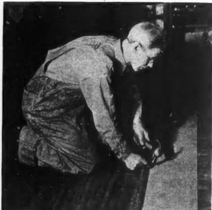
Factory Finished Flooring, Bored for Nails and Designed to Produce a Perfectly Even Surface.
