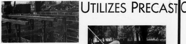
Temporary Wood Shores on Which the Gypsum Floor Units Are Supported While the Reinforced Concrete Beams Are Being Cast in the Troughs of the Gypsum Floor Form Units.
