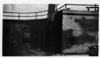
A Railroad Retaining Wall Before and After Being Repaired, with Pulverized Iron Used as a Bonding and Waterproofing Material, Shows the Perfect Results Obtained.
