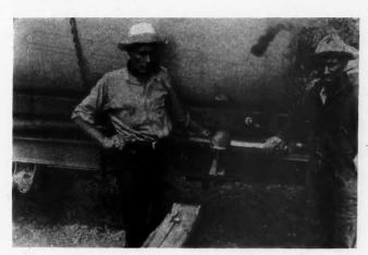
A Frame Attached to the Truck Chassis for Hauling Heavy Pipe.
