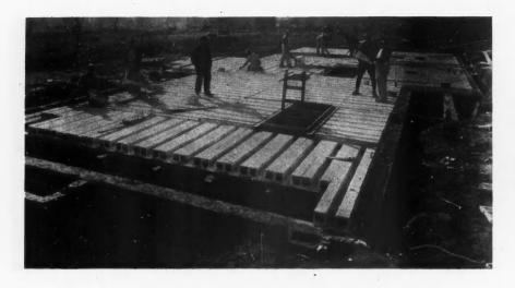
When the Gypsum Floor Units Are Laid the Thin Web Over the Center Hollow of Each Floor Unit Is Sawed Away, Thus Making a Series of Parallel Troughs Which Serve as Forms for Reinforced Concrete Floor Beams Running from Wall to Wall. The concrete is poured over the entire floor surface, thus making a concrete floor slab of any desired thickness with finished plaster ceiling underneath.
