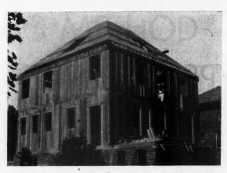
After the Gypsum Supported Concrete Slab Floor Is in Place, Vertical Units Form the Exterior Walls; Openings Are Left for Doors and Windows and Walls Are Complete Ready for the Exterior Veneering.
