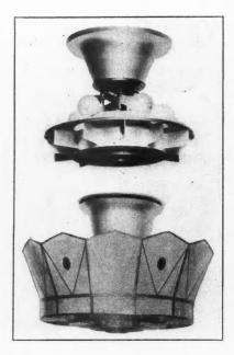
Two Purpose Lighting Fixture with Its Construction Shown Above.
