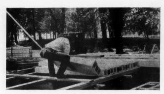
Placing the Gypsum Floor Units on the Temporary Wood Shores.
