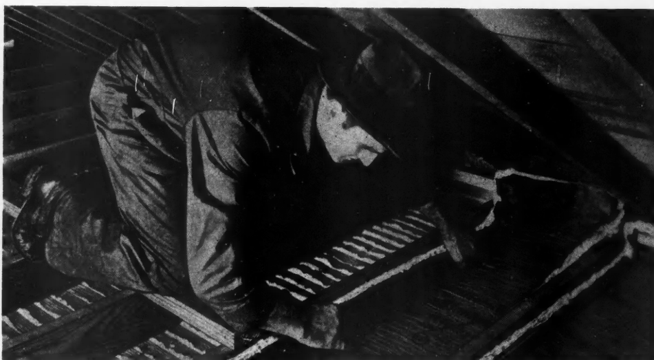
Flexible Blanket Insulating Materials Are Most Effective When Applied Between Studs, Joists, or Rafters, Dividing the Enclosed Air Space.
