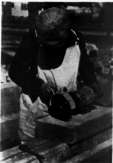
Scoring Stone Slabs with Power Saw for Breaking to Length.
