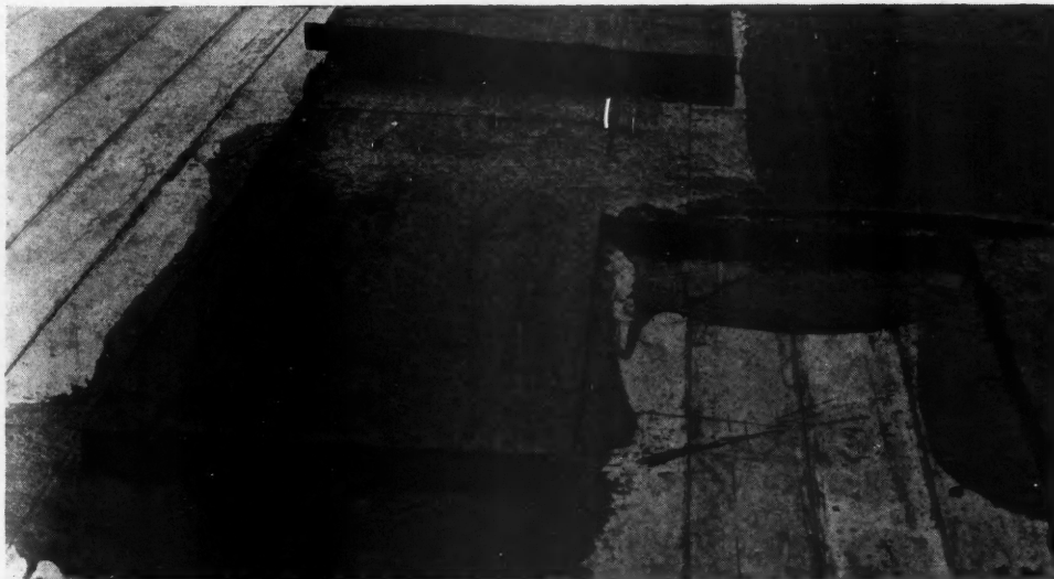
Insulating Boards Are Applied to Concrete or Steel Deck Roofs with Asphalt and Covered with Built-up Roofing of Various Types.
