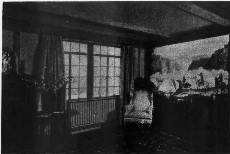
New Type Concealed Radiation Under the Window.
