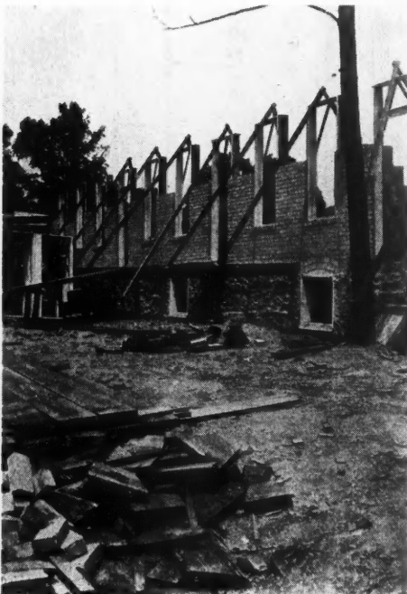
Supports Keep Frames in Position for Bricklayers on City Co. Job, Baltimore. At Right Above: Canopy Braces
