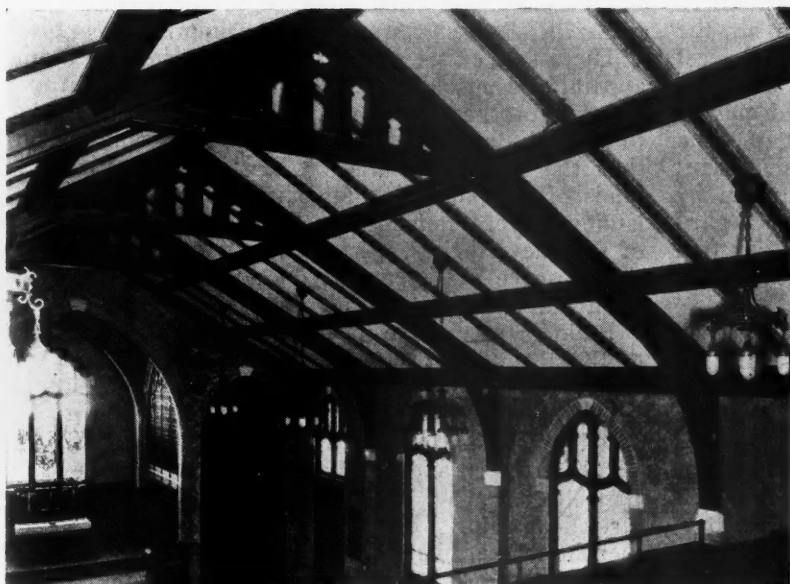
An Example of the Use of Fiber Insulating Board as an Interior Finish and Acoustical Material with Satisfactory Decorative Effect
