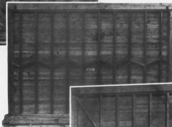
Fig. 2 (Above) — Herringbone Braces Add Little Stiff- ness.
