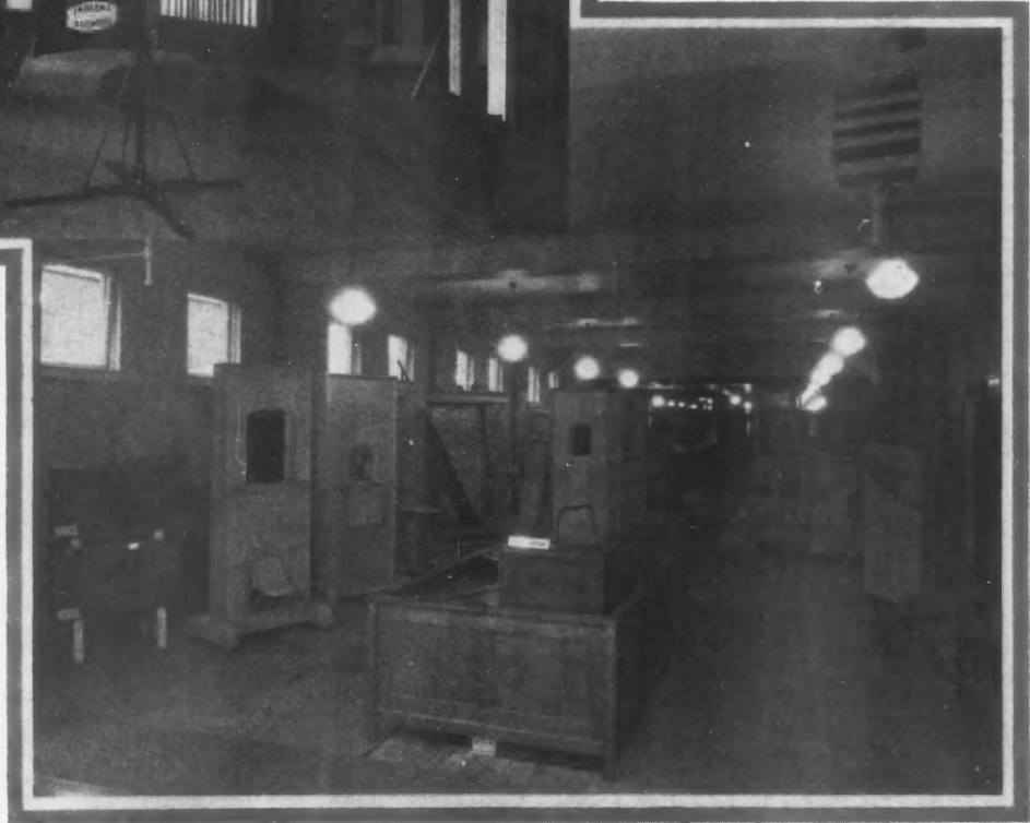
Sample and Display Rooms in the Offices of the In- diana Lumber & Mfg. Co., South Bend, Ind.
