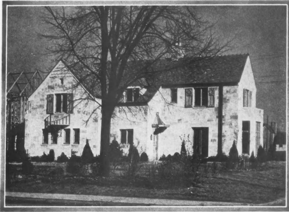
First Indianapolis Steel Frame House, Pennsylvania Avenue and East 57th Street; Limestone Exterior.
