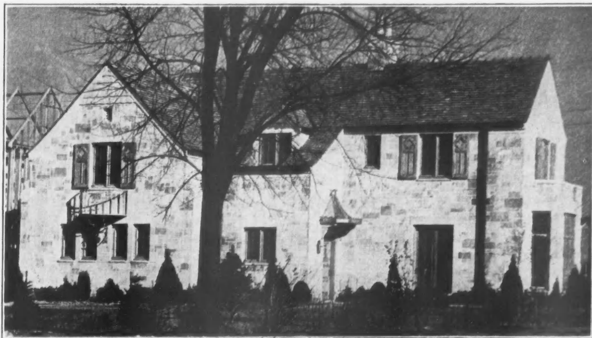
Residence in Indianapolis built by the Steel Framing method, and developed in blue-gray Indiana Limestone. Frederick Wallick, Architect.
