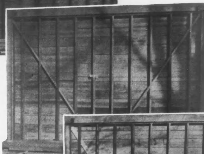
Fig. 3 (Above) — Diagonal 2 by 4 Cut-In Braces Im- prove Stiffness 60%.
