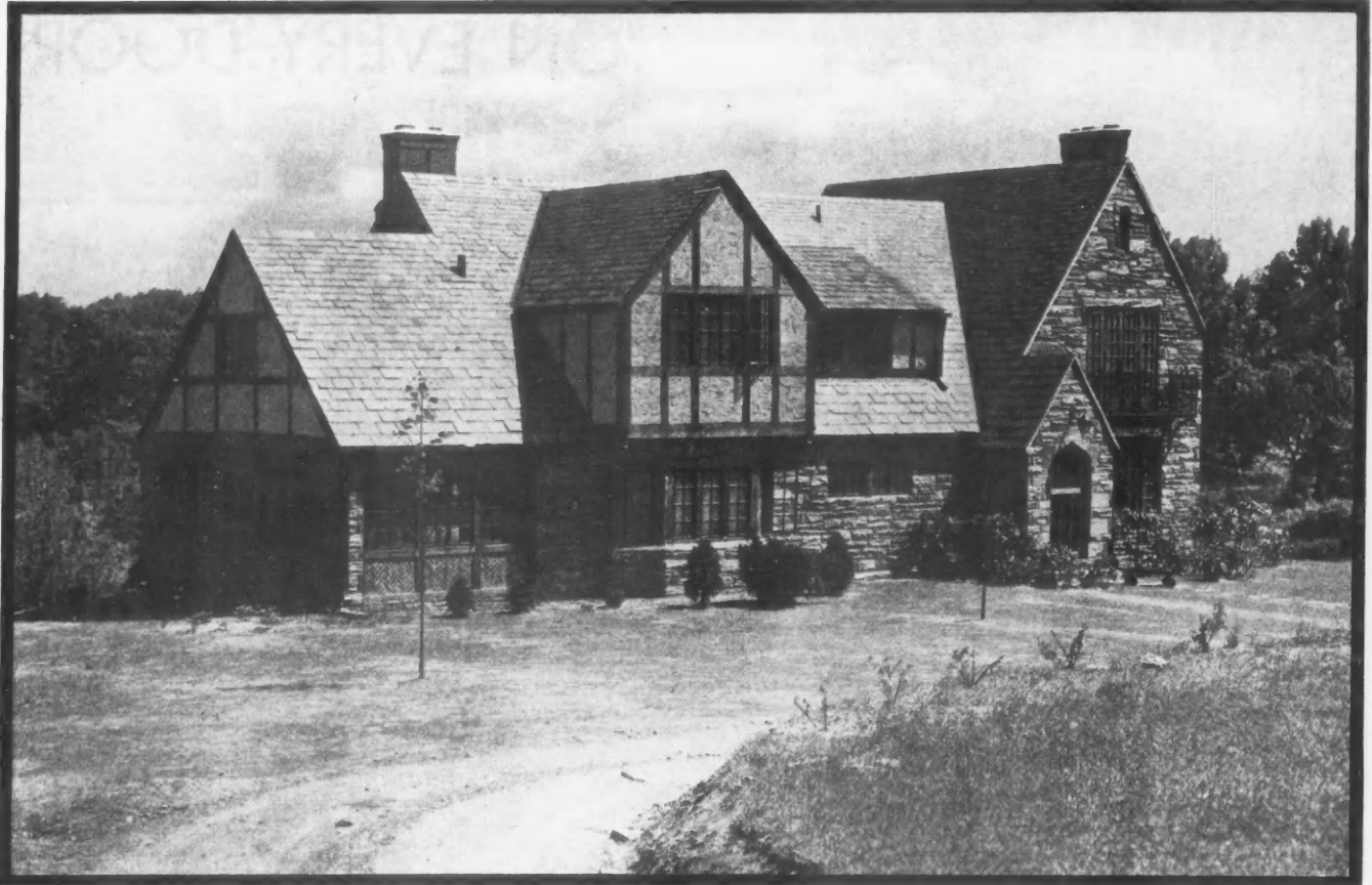
Lupton Casements enhance the charm of the James P. Henry residence, Wallingford, Pa. Flounders Bros., Builders, E. Kenney Crothers, Architect.
