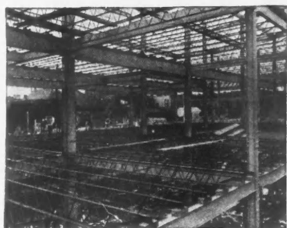
TRUSCON STEEL JOISTS for permanent floor construction, quickly erected at low cost
