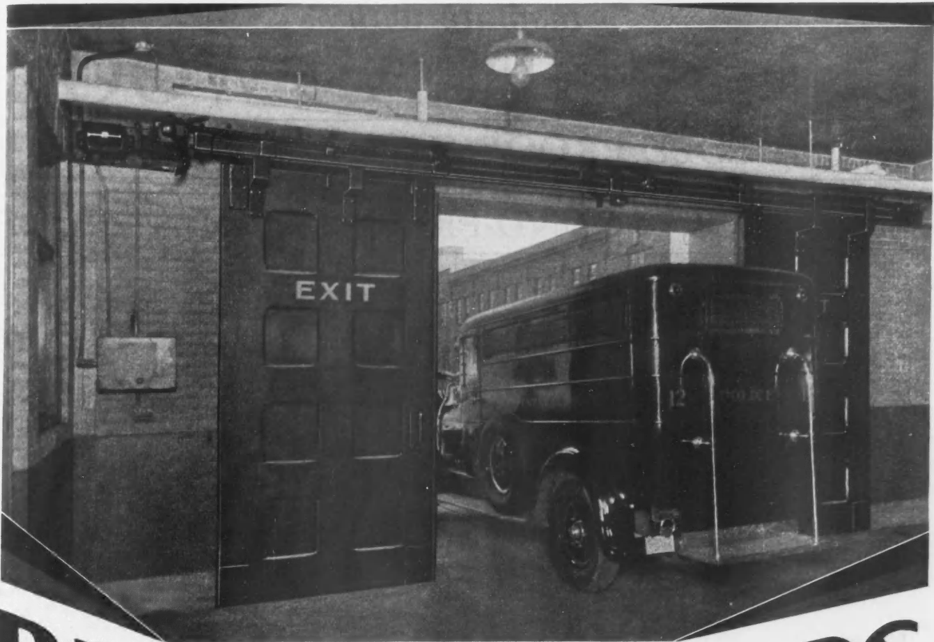
Police Headquarters Garage, St. Louis, Mo. . . . R-W equipped
