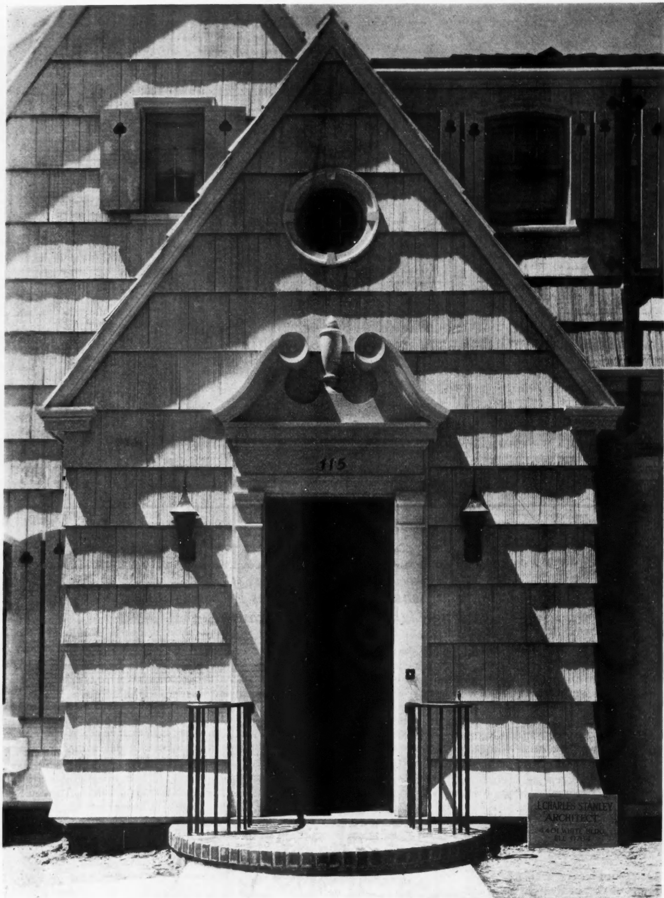
Cedar Shakes on the Outside Walls Play a Large Part in the Effectiveness of This "American Builder" All-Feature Home Design as Developed by J. Charles Stanley, Architect.
