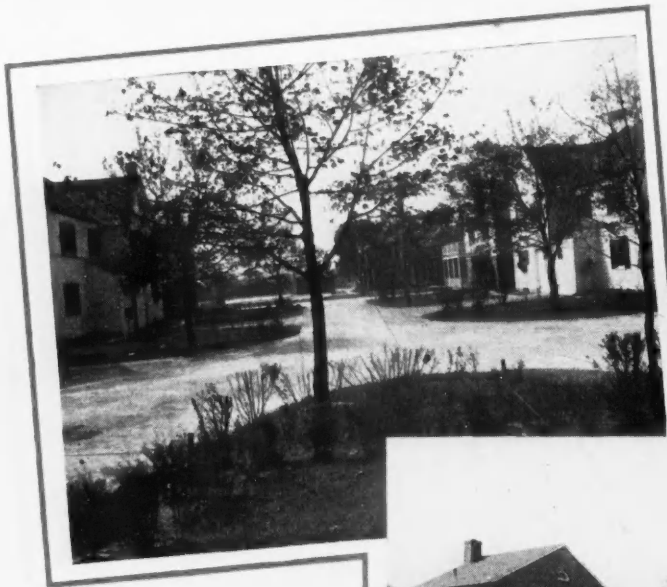
At Radburn the Short, Closed-end Street (Above) Provides Access to Rear Garages, Leaving the Beauty of the Garden Side (Upper Right)—Unmarred.
