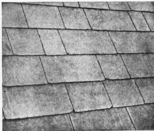
Permanent Colors and Rough Uneven Butts Makes Possible Artistic Roofing.
