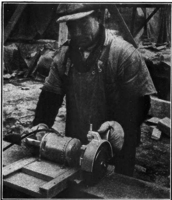
Cutting groove in stone with portable electric saw preliminary to breaking. A tap with a mallet on the opposite side breaks the strip clean on a line with the groove. One man keeps six stonemasons or bricklayers busy laying up stone!
