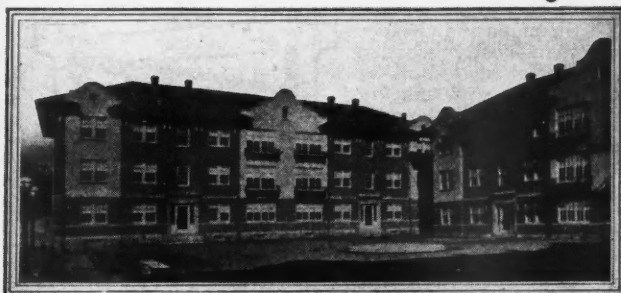
Terrace Court Apartments, Pittsburgh, Pa. equipped with du Pont Tontine.
