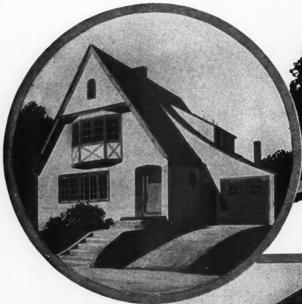
Garage Addition Provides the English Style with Another Sweeping Roof Line
