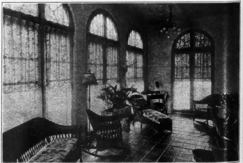
The Concrete Slab Itself May Be Marked Off Into Square or Irregular Patterns to Resemble Tiling Before the Concrete Has Received Its Initial Set.
