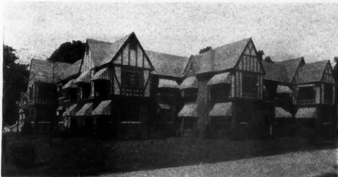
Another apartment house job of the Webb-Clark organization, the Elizabeth Apartments, Louisville. Note size of Fenestra Casements.
