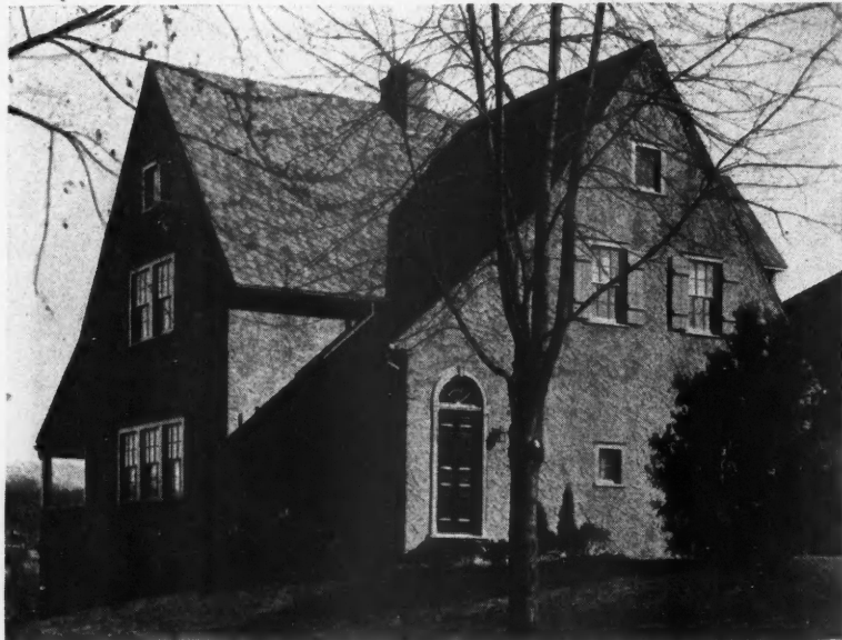
Variegated Colors Add to the Attractiveness of the Asphalt Shingle Roof on This Comfortable Looking Home.
