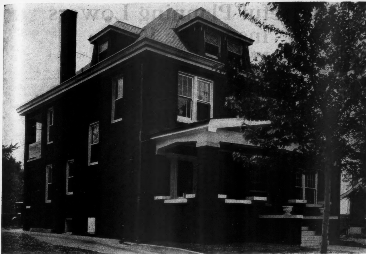
With the New Porch Completed and the Brick Veneer All Laid the House Would Hardly Be Recognized as the Same as That Shown Below on This Page. It is a fine example of the kind of permanent remodeling that is possible with an overcoating of brick veneer.
