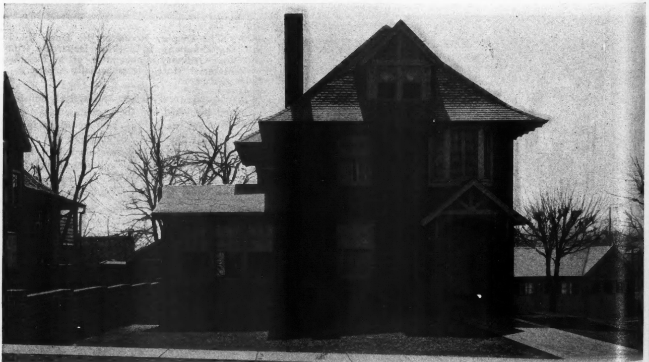
The Old Boyer Residence as It Appeared After Being Brought Up-to-Date. A sun room and garage, brick walks and brick wall were added and the house was completed overcoated with a handsome face brick. It is now considered one of the really fine, modern homes of the town and a highly salable property.
