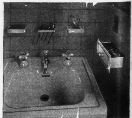
A Convenient Drawer, Built Into the Bathroom Wall Takes Care of Miscellaneous Articles and Keeps Them Free of Dust.
