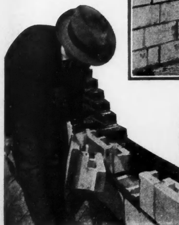
This picture shows how light weight and smooth surface of tile contribute to ease and speed of placing. Wide side walls contribute to ease of placing mortar and materially reduce mortar loss.
