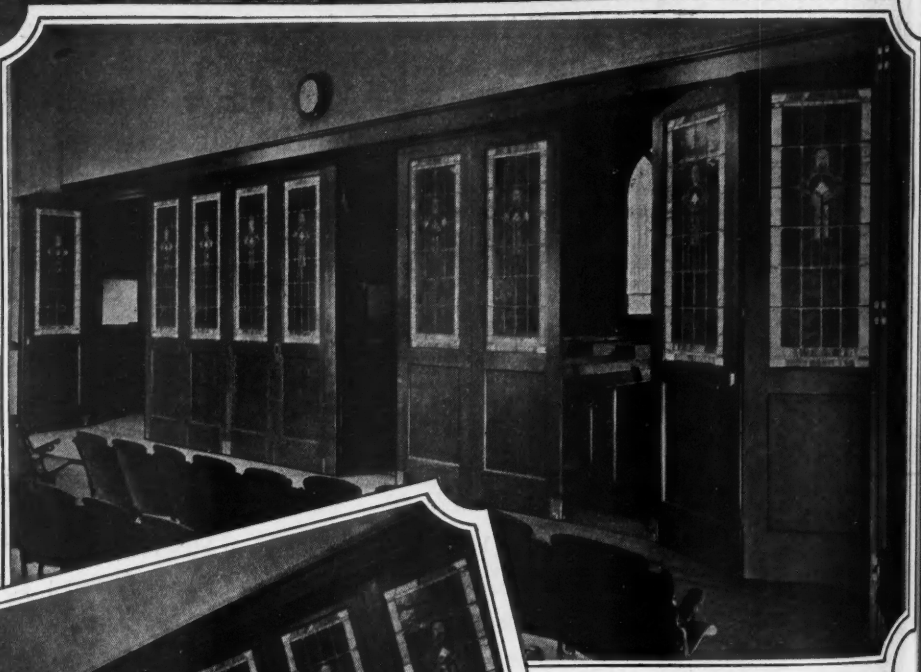
To right is shown how doors slide and fold in hinged pairs. Overhead hangers and track serve as a guide, with weight supported on floor track and ball bearing rollers.
