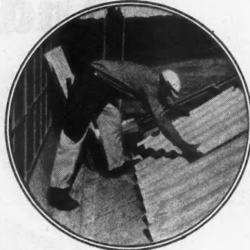
Eternit "Big-Seven" Corrugated Sheets have extraordinary strength—made possible by the 7" corrugation span.
