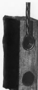
For two-hole sash, the coil spring is inserted in the upper hole, slipping the coil into end link and inserting in same manner as with single-hole sash.
