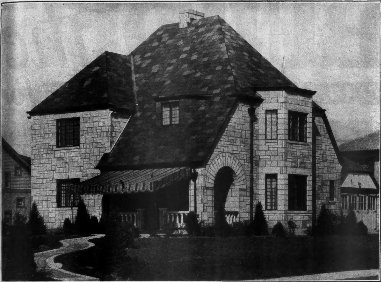
Chas. E. Carter residence, Indianapolis, Indiana. C. T. Myers, Architect. Built of Old Gothic Indiana Limestone Random Ashlar
