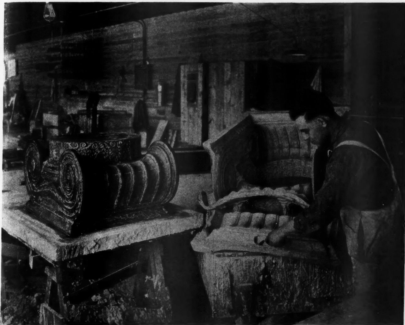
Making a Plaster Mold for a Column Capital. Into these molds the plastic concrete is cast and after it is thoroughly hardened the molds are cut away leaving the casting to be finished by skilled carvers.
