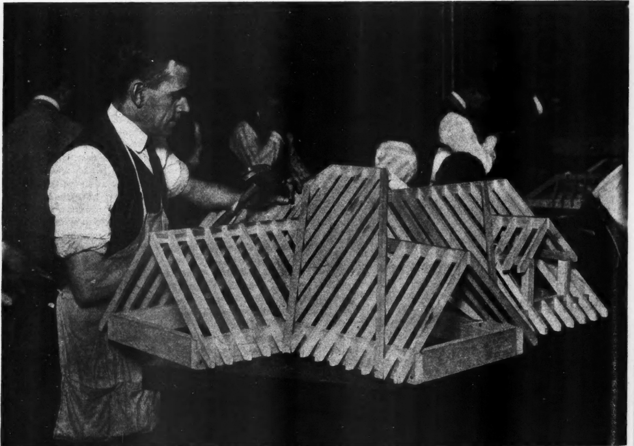
A Practical Exercise Problem in Roof Framing as Taught in the Evening School at Pratt Institute.
