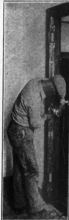
Hinge Butt Router and Templet on Jamb
