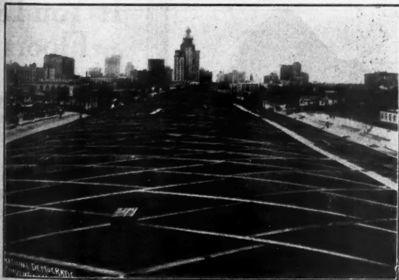
Top View of Roof Construction, National Democratic Convention Hall, Houston, Texas.
