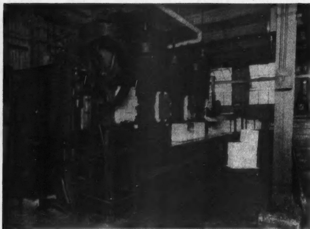
A New Type of Refrigerant Is Being Produced Here, Frozen Carbon Dioxide in Solid Form, Which Has a Temperature of 114.5° Below Zero and on Melting Leaves no Moisture.
