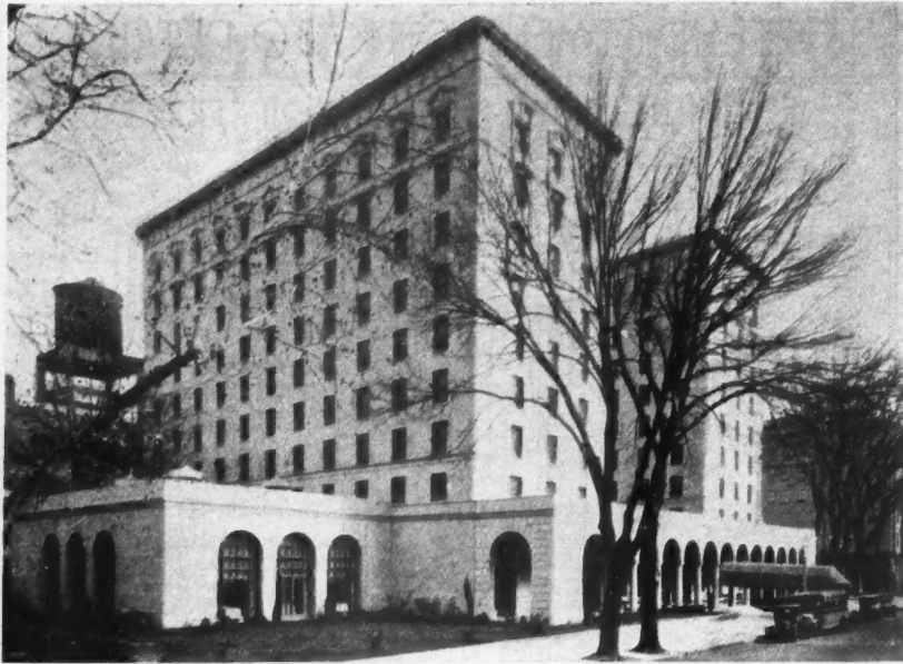
Stucco Exteriors Are as Suitable for Large Buildings as They Are for Small Bungalows. The Hotel Senator, Sacramento, California, is a notable example in support of this.
