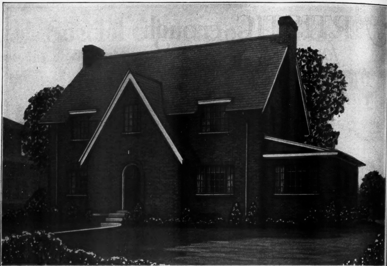
Masonite Insulating Lath was used as a plaster base in this attractive home located in South Bend, Indiana. Owner, Mrs. Caroline C. McNamara. Architect, Russell H. Stapp. Contractors and Builders, Whitcomb & Keller Real Estate Builders
