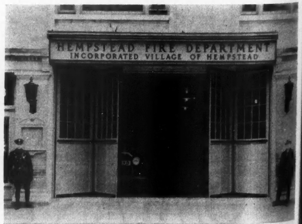
These Doors Are of a Quick Acting Type Which Has Been Found Particularly Suitable for Fire Stations.
