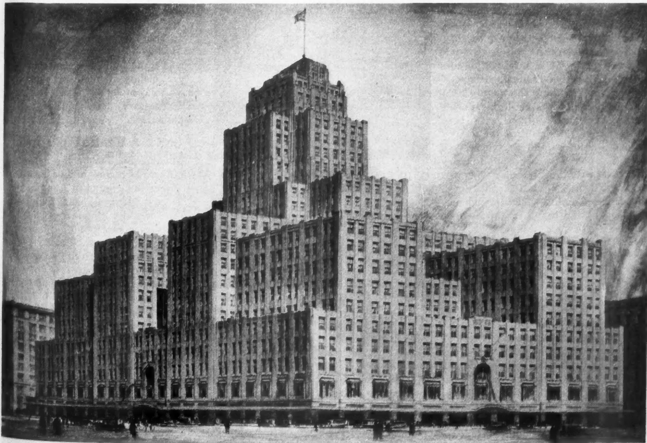
This Picture Shows How the World's Largest Building Will Look on Completion. It is now under construction in Boston and will cost $21,000,000. The ground area of the site contains 130,000 square feet and the building will be 25 stories in height and contain a permanent population of 20,000 people.
