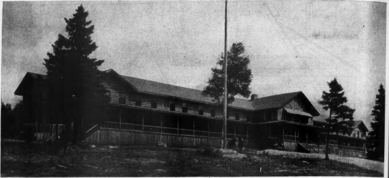
The Log Lodge at Lucerne-in-Maine Was Built from Materials Cut in the Immediate Vicinity and Its Rustic Construction Makes It Notable for Its Appropriateness as Well as for Being One of the Largest Log Structures Ever Built.
