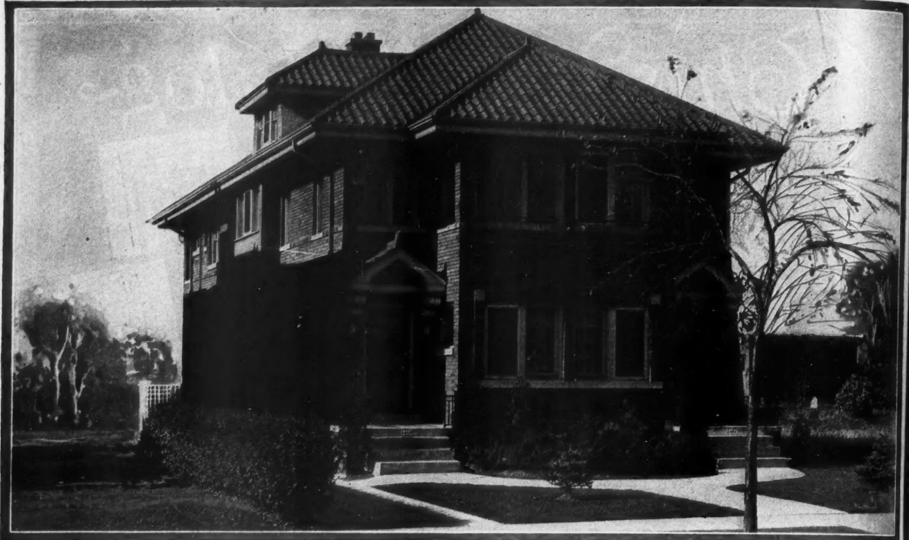
Sheet Steel Spanish Mission Tile Roofed Duplex House at 1489 Downer Avenue, Milwaukee, Wis.
