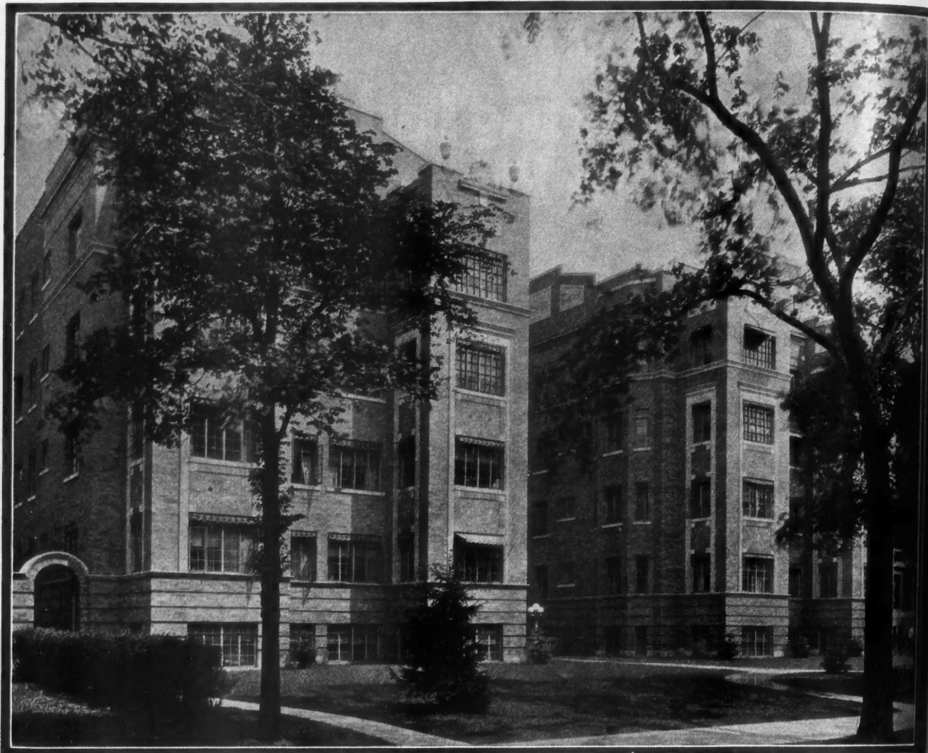
The Lerchen Apartments, Detroit. Ralph T. Lee, Architect. A. T. Lerchen, Owner and Builder.
