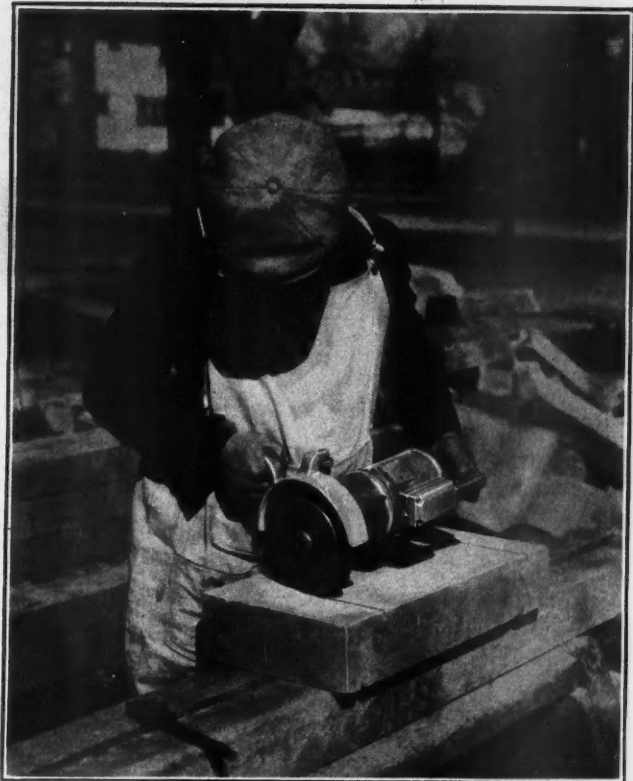
Electric saw replaces old-time mallet and chisel for breaking Indiana Limestone. One man now keeps six stone masons busy!
