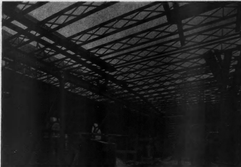
This Type of Truss-Joist, Made by Expanding Standard I-Beams, Is Exceptionally Strong, Light and Economical.
