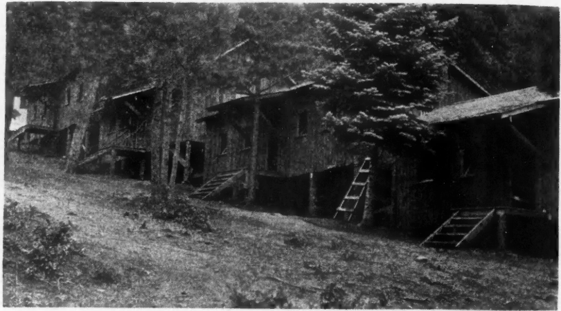
Scout Sleeping Cabins at Camp Burch, Pueblo, Colorado. Each is 16 by 30 feet and accommodates eight to ten boys with a window for each boy, assuring ample ventilation.
