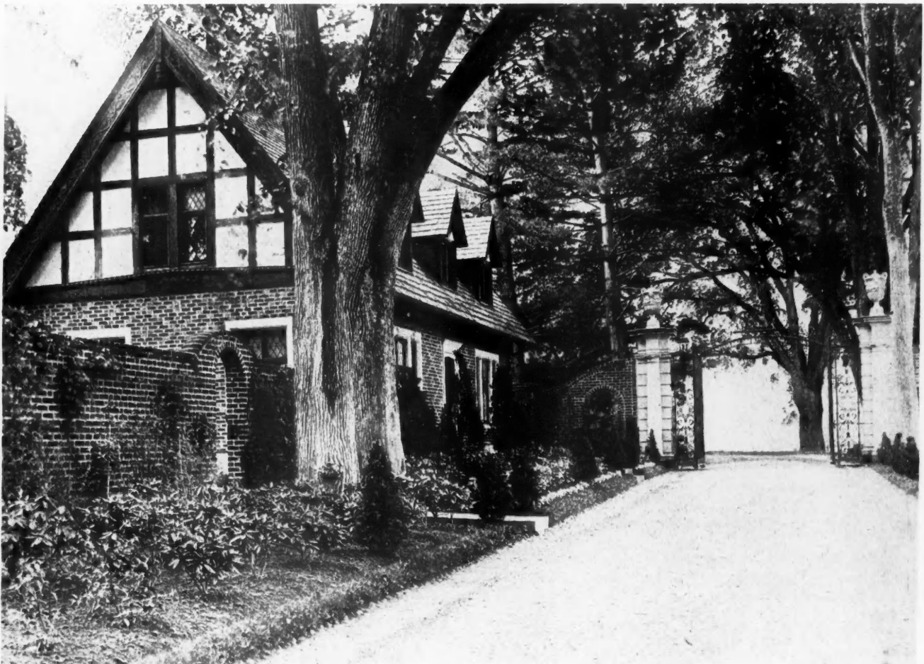
The Garden Wall Lends an Air of Privacy to the Outdoor Living Room Especially Necessary in This Day of Constantly Passing Traffic. Here the wall of brick, with well proportioned arch, is built in the style of the house making the house and garden seem one.
