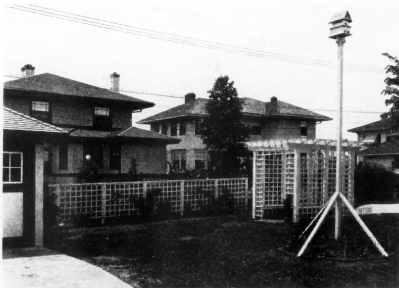
Dressing up the Backyard Is a Piece of Strategy on the Part of the Builder. Here is an arbor seat and lattice fence which add to the desirability of the home.
