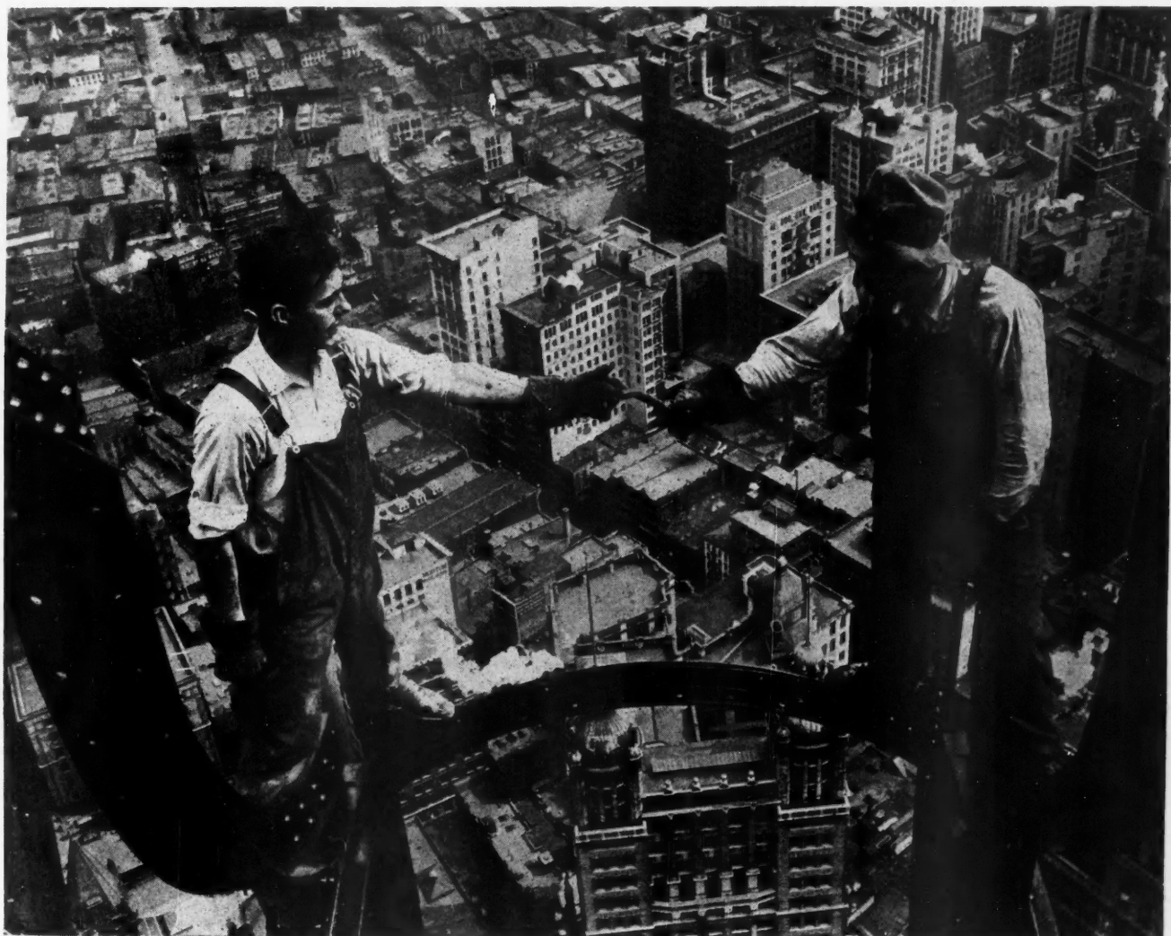
Where Daring as Well as Skill Is Required. This steel framework is 790 feet above the street level. The picture was taken when the Woolworth Building was under construction.
