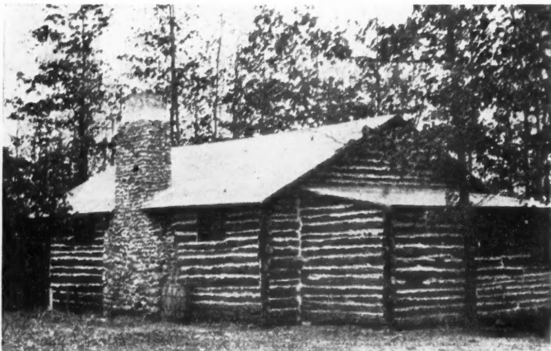
Toledo Council Boy Scouts Troop 23 Camp, an Attractive Example of the Rustic Log Home with Fireplace Chimney of Native Boulders.
