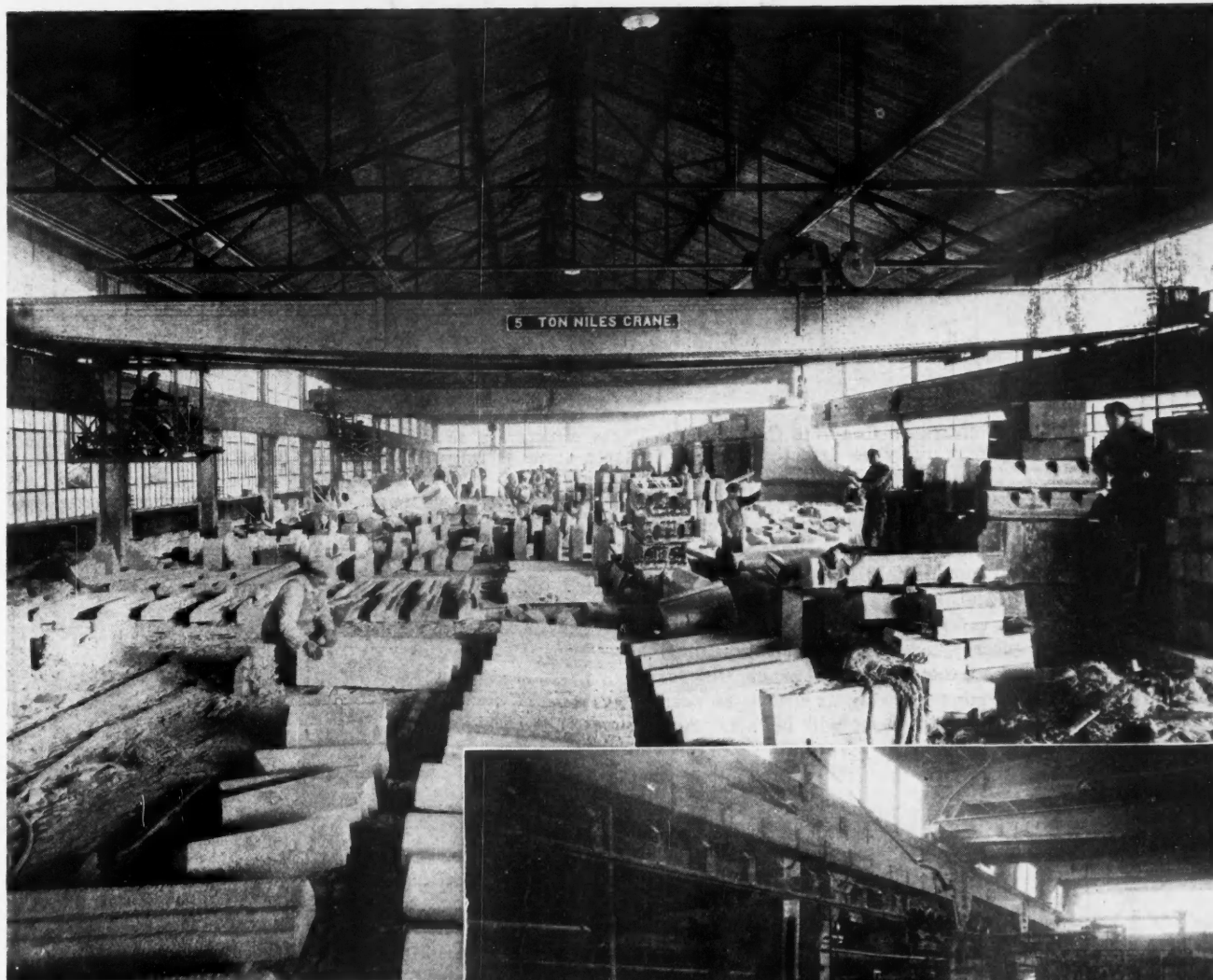
Casting Room of a Large Concrete Stone Company—the Simbroco Stone Company, Boston. Notice the two large capacity, overhead traveling cranes which handle these heavy pieces.
