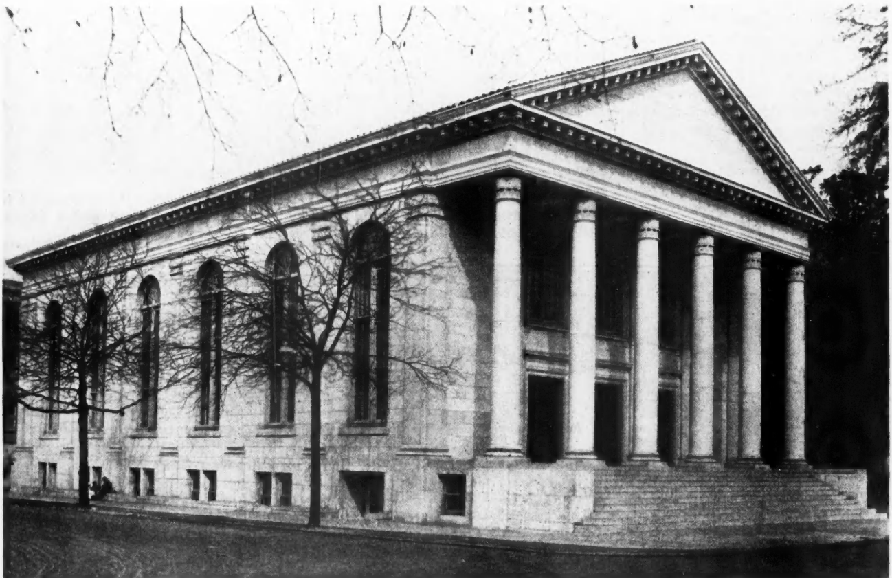
First Baptist Church, Savannah, Ga., Built of Concrete Stone Which Has Been Cut and Tooled After Casting. Stone work executed by Cut Art Stone Company, Savannah. F. McRae, builder, and Henrik Wallin, architect.
