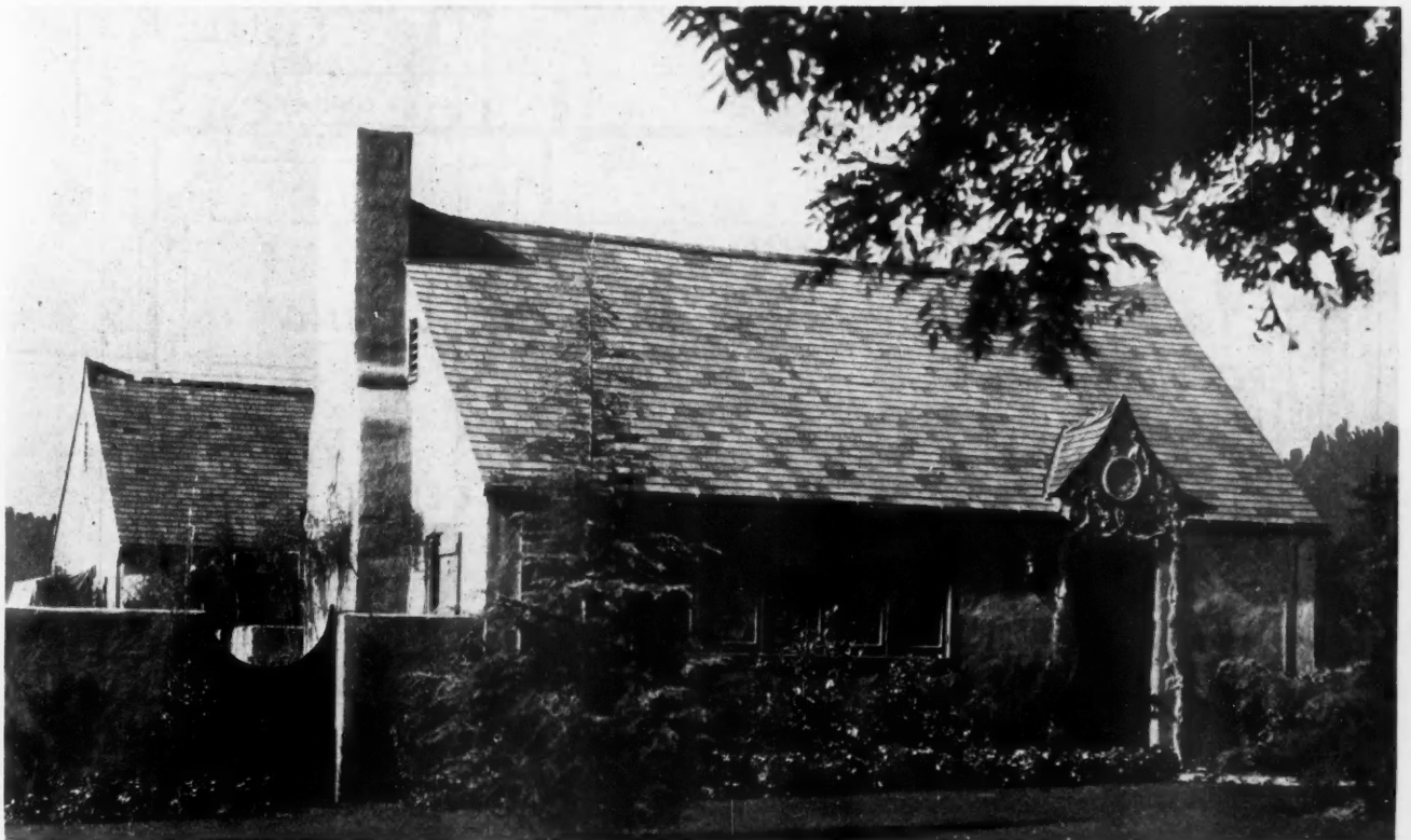
Delightful Six-Room Cottage of French Design as Illustrated on Our Front Cover This Month in Full Colors. Floor plans, elevations and details of construction are on the four pages following.
