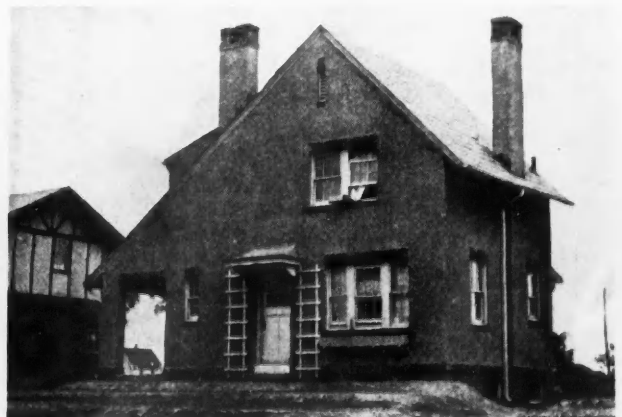
Fig. 4. A Good Base Course and Brick Shoulder Course Protect These Stucco Walls Where the Site Has Been Terraced.
