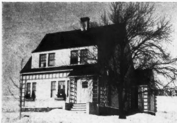
Fig. 2. Unless the Stucco Is Stopped Above the Grade Line as in This House, Soot Falling on the Snow Will Stain It.
