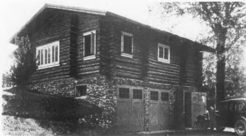
There Is a Three-Car Heated Garage Under the Smaller Cabin with the Entrance at the Rear on the Lower, Hillside Level.
