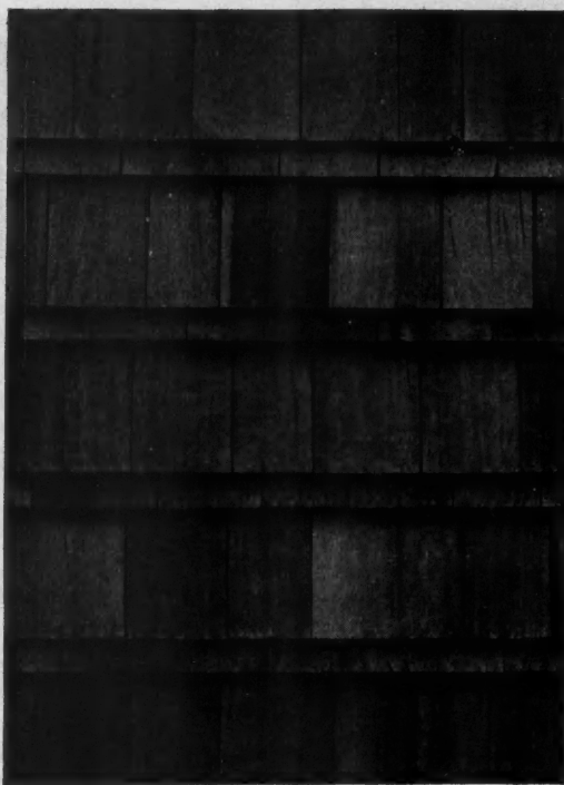
A Very Popular and Economical Sidewall Design of 12-Inch Shingles, Sometimes Called the "Ribbon Course." It is laid with 6-inch exposure for the wide course and 2-inch exposure for the narrow course.
