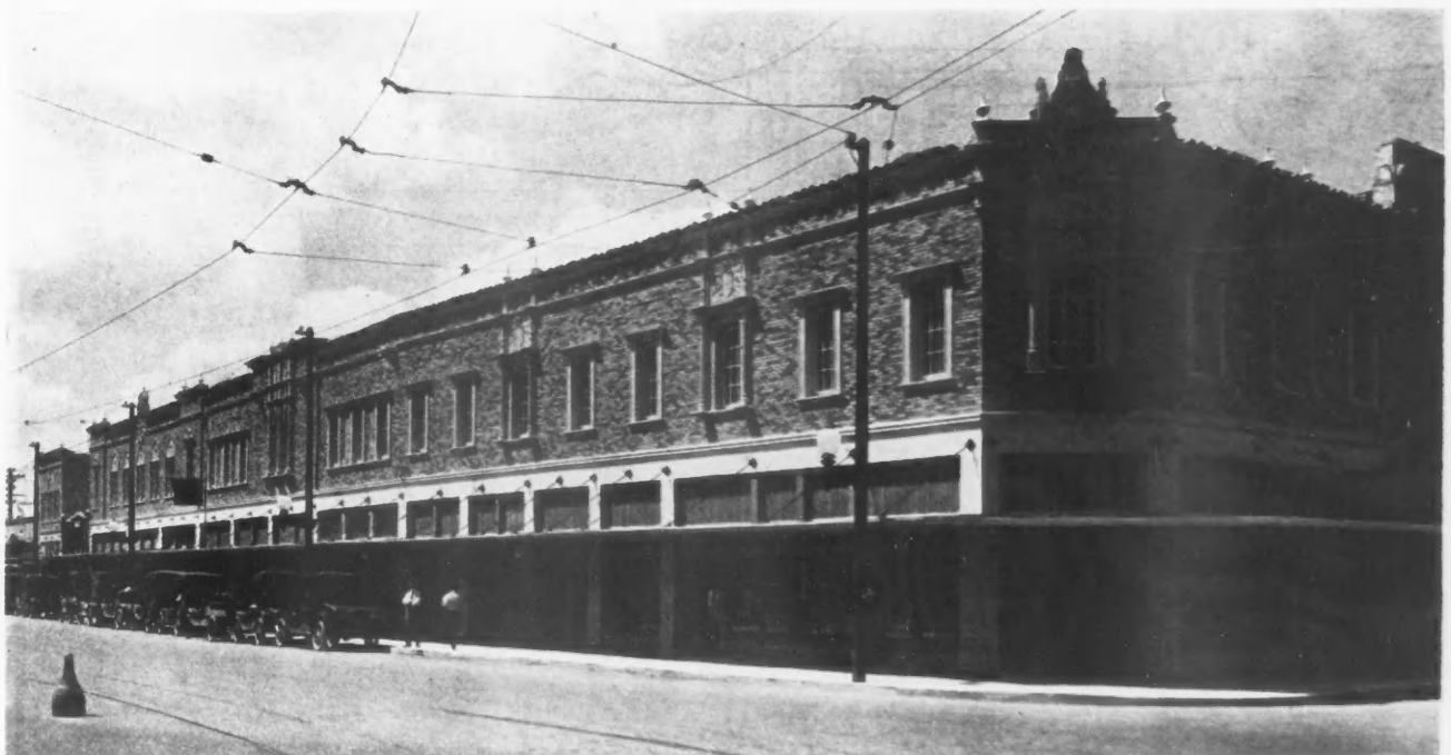
The Kallison Block in San Antonio, Texas, Is the First Commercial Building in that City of Spanish Origin to Display a Spanish Influence in Its Architecture. The result is an attractive as well as useful type of building.
