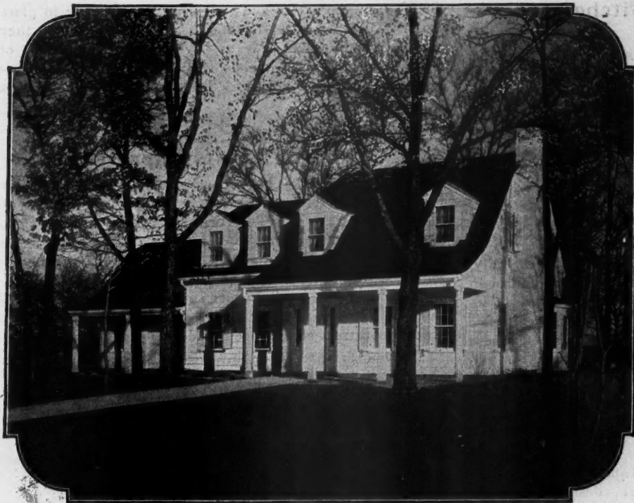
6500 square feet of Celotex Insulating Lumber was used as insulation with plaster applied directly to its surface in this residence of H. C. Wehmann, in Interlachen Park, Minneapolis. C. J. Bard was the architect, and the Holm-Johnson Company the builders.
