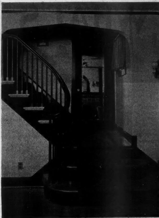
The Stairway May Be Made a Most Effective Feature of the Home by Attention to Perfection of Design.
