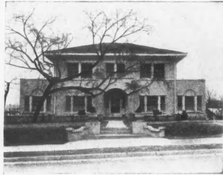
This is a Rocbond home in Hot Springs, Ark.—No. 531 of a series of 10,000 superfine Rocbond jobs.
