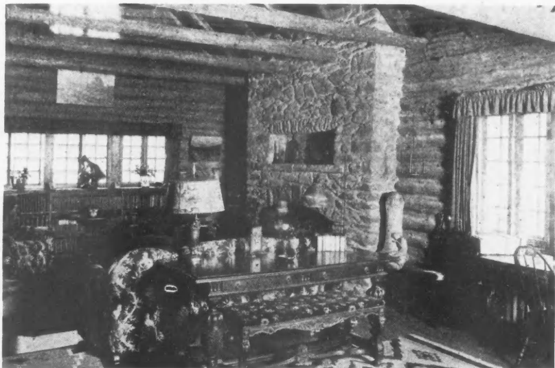
The 18 by 30 Foot Living Room Extends Up to the Roof with Exposed Log Beams, Rafters and Walls and with a Great Stone Fireplace at One Side.
