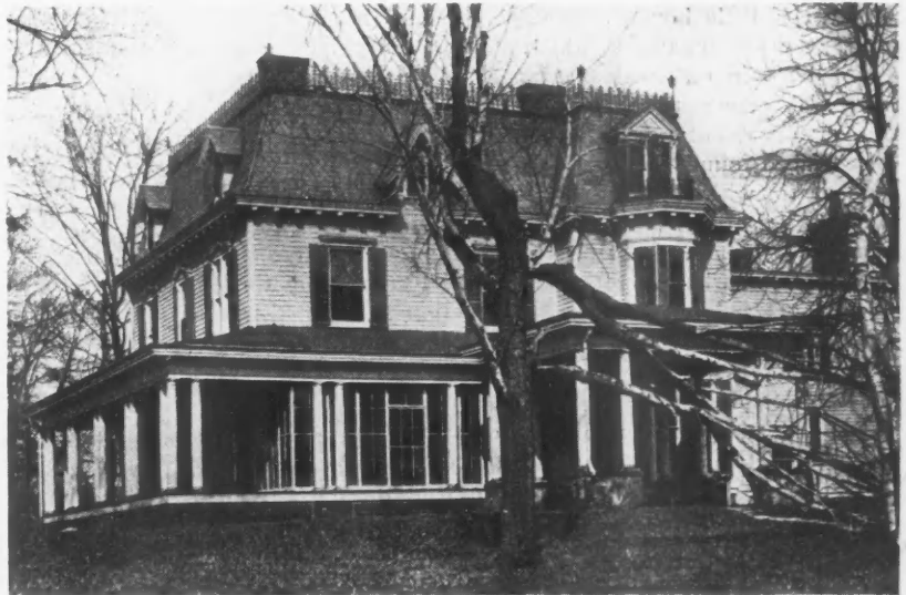
This Old Residence in Englewood, N. J., Had Apparently Lost Its Value Beyond that of the Ground on Which It Stood Until an Enterprising Local Builder Took Charge and Subjected it to a Remodelling Along Modern Lines.
