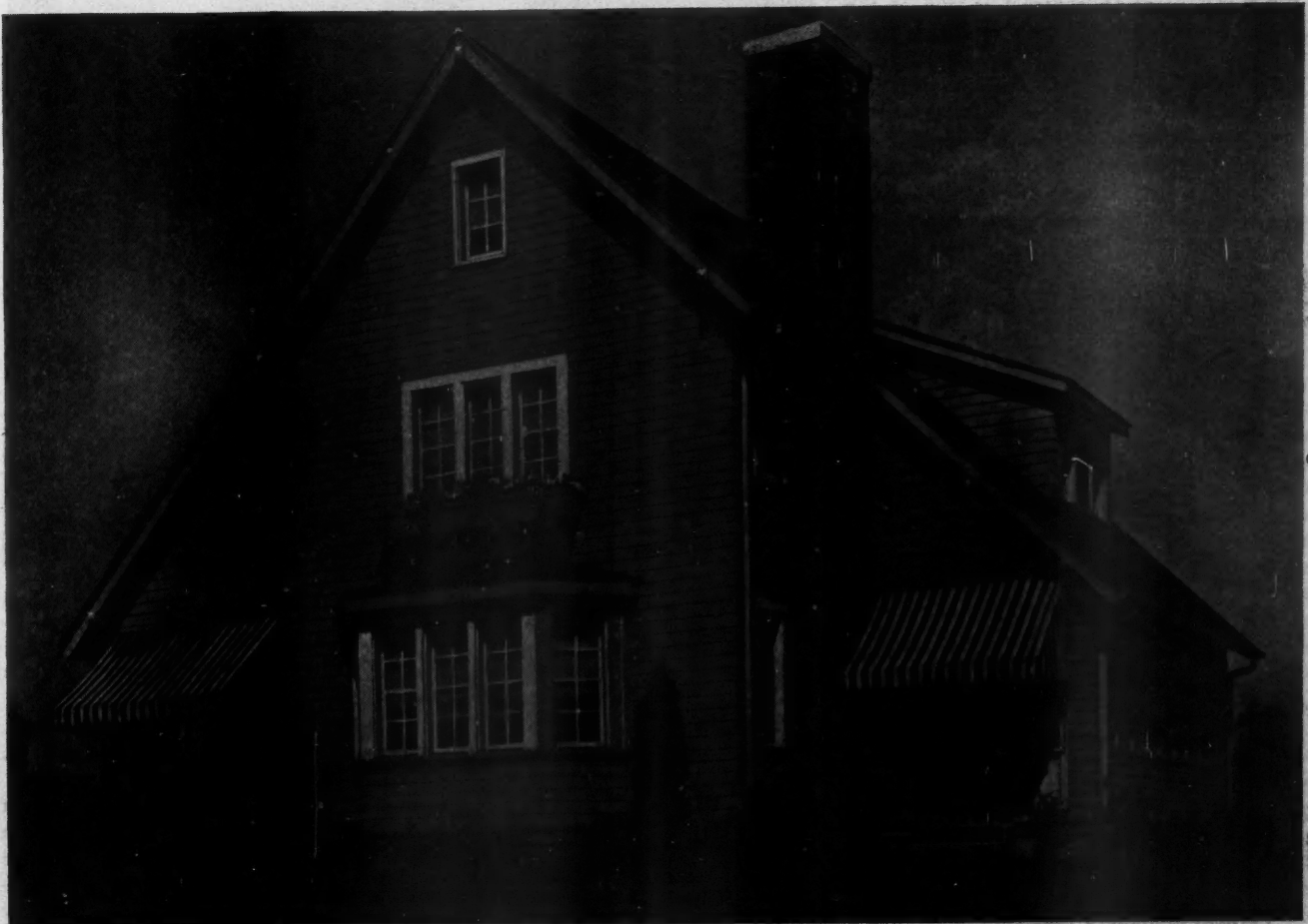
A Sturdy New House Represents the Honest Workmanship of the Builder Plus the Honest Service of the Dealer. A well built house is a monument to these two men.
