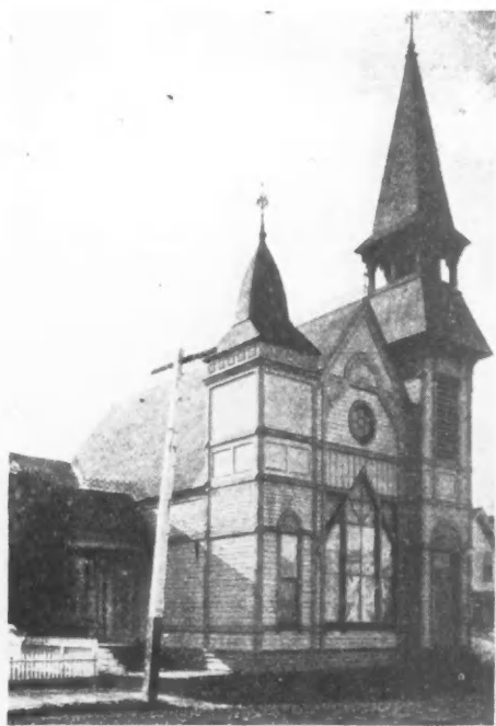
The Old First Presbyterian Church of Watsonville, California, Which Was Remodeled Into a More Attractive Building.
