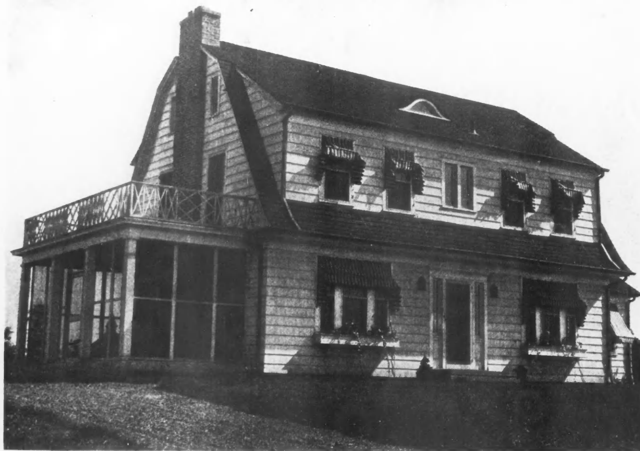
This Comfortable Residence, on Staten Island, N. Y., Presents an Inviting Appearance to the Passer Which Is Carried Out Throughout the Interior. Comfort is evident in the large living room with its fireplace, the screened porch and the general arrangement of rooms. The second floor plan shows seven separate closets in addition to one on the first floor. It is the work of Harry Lucht, Cliffside, N. J., architect.
