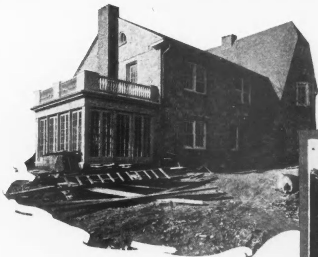
Residence of E. P. Williams, Easton, Pa. Built of Cinder Concrete Building Units. Photos show residence under construction and after completion. Architect, Paul Smith, Phillipsburg, N. J.; Contractor, E. P. Williams, Easton, Pa.
