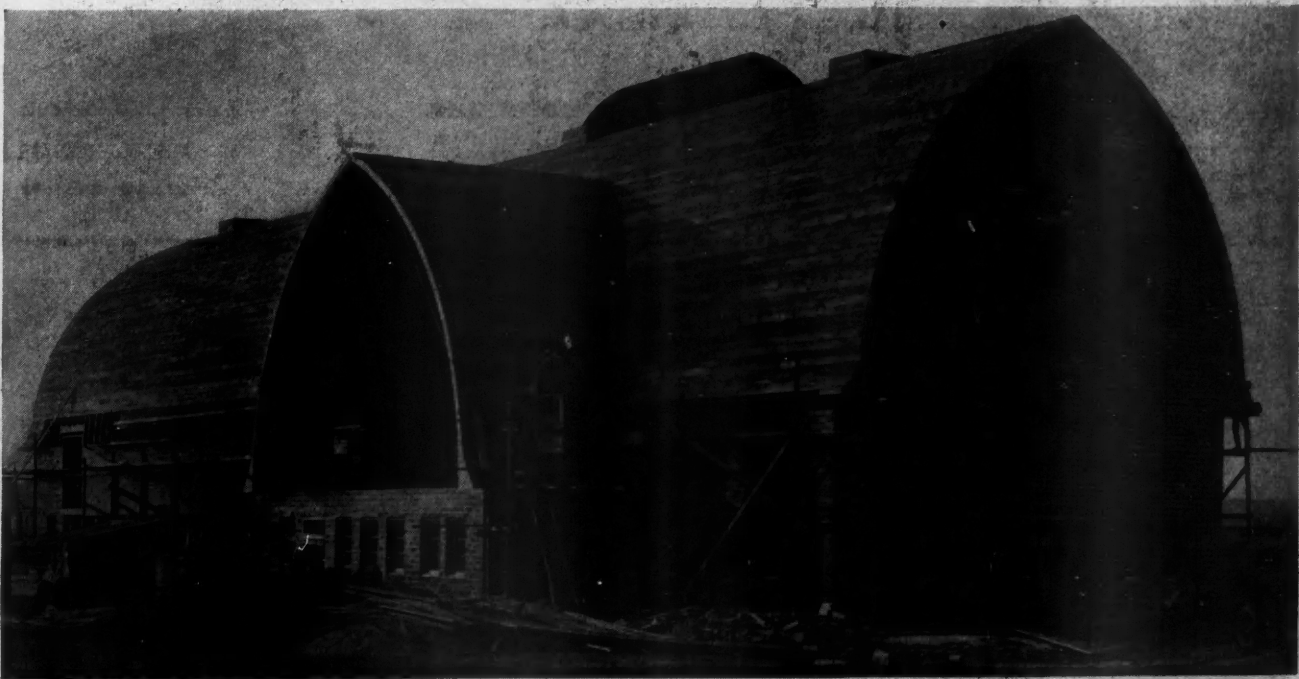
This, the Largest Dairy Barn in Minnesota, if Not in the Entire Country, Was Built to House a Famous Prize Herd of Holstein Cattle and Its Construction, of Hollow, Vitrified, Clay Tile, Makes It a Fine Appearing Building Providing for the Best Possible Care of Its Valued Occupants.
