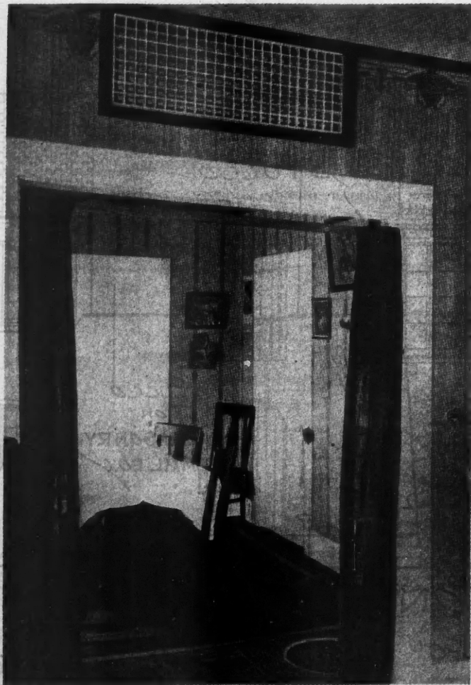
Fig. 1. A Wooden Grille Set in the Walls Over the Doorway Permits the Passage of Heat Between Rooms.
