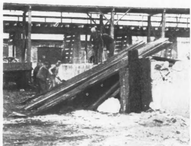
In the Absence of a Blasting Mat, Heavy Lumber, Railroad Ties, or Logs May Be Piled Against the Concrete to Prevent the Throwing of Material.
