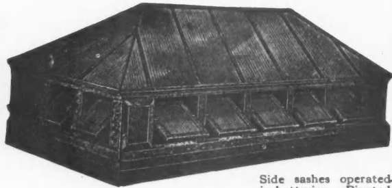
Side sashes operated in batteries. Pivoted to afford easy control.
