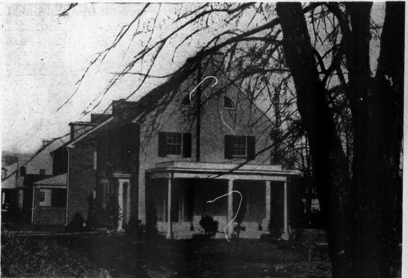
Alexander Sand, Jr., Son of Chief Engineer of the Pennsylvania Railroad, Has Built a Group of Straub Cinder Block Houses in the Aristocratic Narberth Section of the Philadelphia Suburbs. The house in the foreground was designed by the brilliant young architect, Walter K. Durham, inspired by a visit to Washington's Headquarters at Valley Forge. Those familiar with the old building will readily see the source of the inspiration. These houses are shown in this photograph. Mr. Sands' home is the house shown in the foreground.
