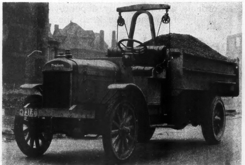
This Truck Is Powered by All of a Fordson Tractor Except the Wheels.
