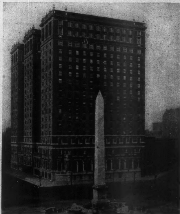
The New Hotel Statler at Buffalo, Opened Last May 19, With Its 1,100 Rooms and $9,000,000 Investment. This is one of the two costliest of 1923.
