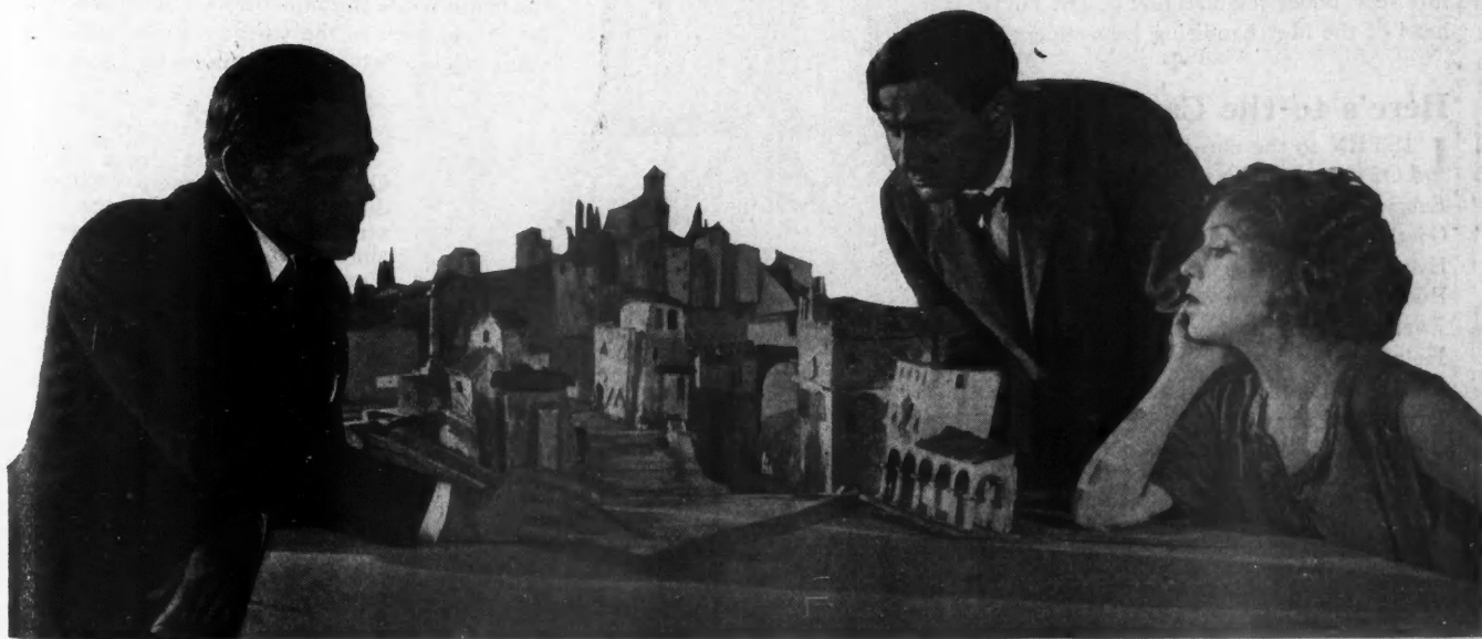
It is the Job of the Builder to Turn Dreams Into Realities and Often His Privilege, Too, to Help Shape and Fashion the Dream. Here we see Mary Pickford in conference with Svend Gade, Danish artist and architect, and Ernst Lubitsch, director. They are visualizing a stage setting of the city of Toledo, Spain, which, when completed, covered five acres.
