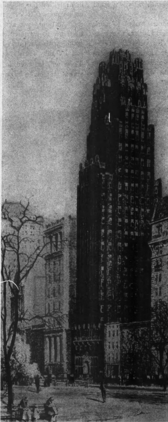
New American Radiator Co. Building in New York City; Black Brick and Yellow Stone Trim. Raymond M. Hood and John M. Howells, Architects.
