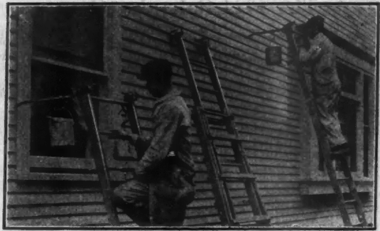
Center Ladder Shows Old Way and Outside Ladders Show New Way of Painting Patented
