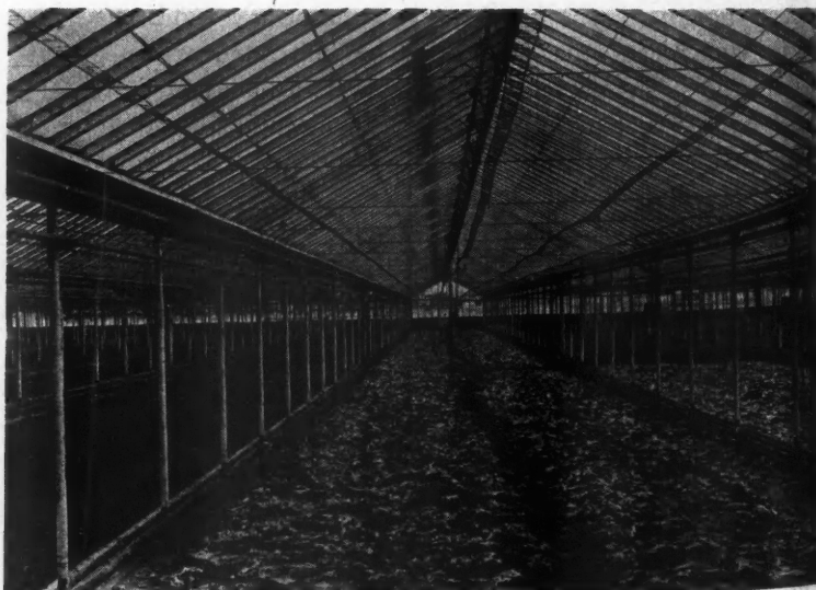
Wrought-Iron or Steel Pipe or Structural Steel in the Form of Bars, Channels or I-Beams Are Used to Support Side Walls and Roof, and Should Be Painted Frequently.
