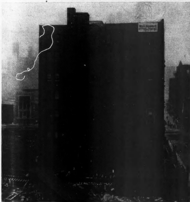
This Seven-Story Building Was Moved 84 Feet, with All Occupants Keeping on with Their Work, and Not Even a Pane of Glass Cracking.
