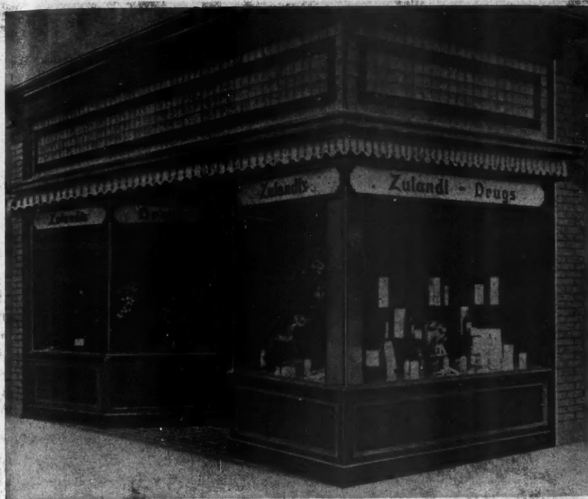
Drug Stores Were the Pioneers in Recognizing the Selling Power of the Properly Arranged Display Window. Prism glass reflectors overhead make the most of daylight.
