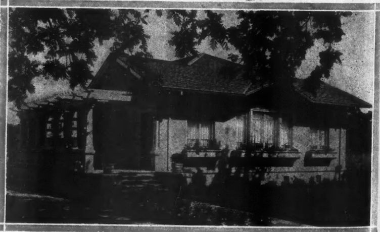
This Delightful 6-Room Electrified Home Is an Inspiration to Better Living.
