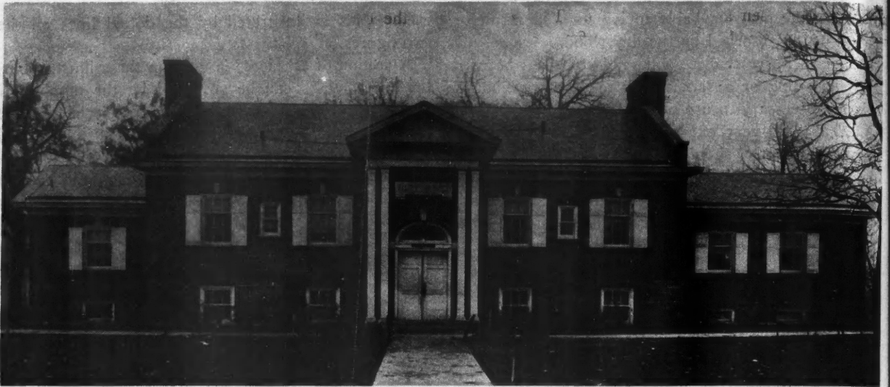
This Colonial Design Grade School Has Its White Trim Contrasting with Red Brick. Its plan has good features Applicable Anywhere.
