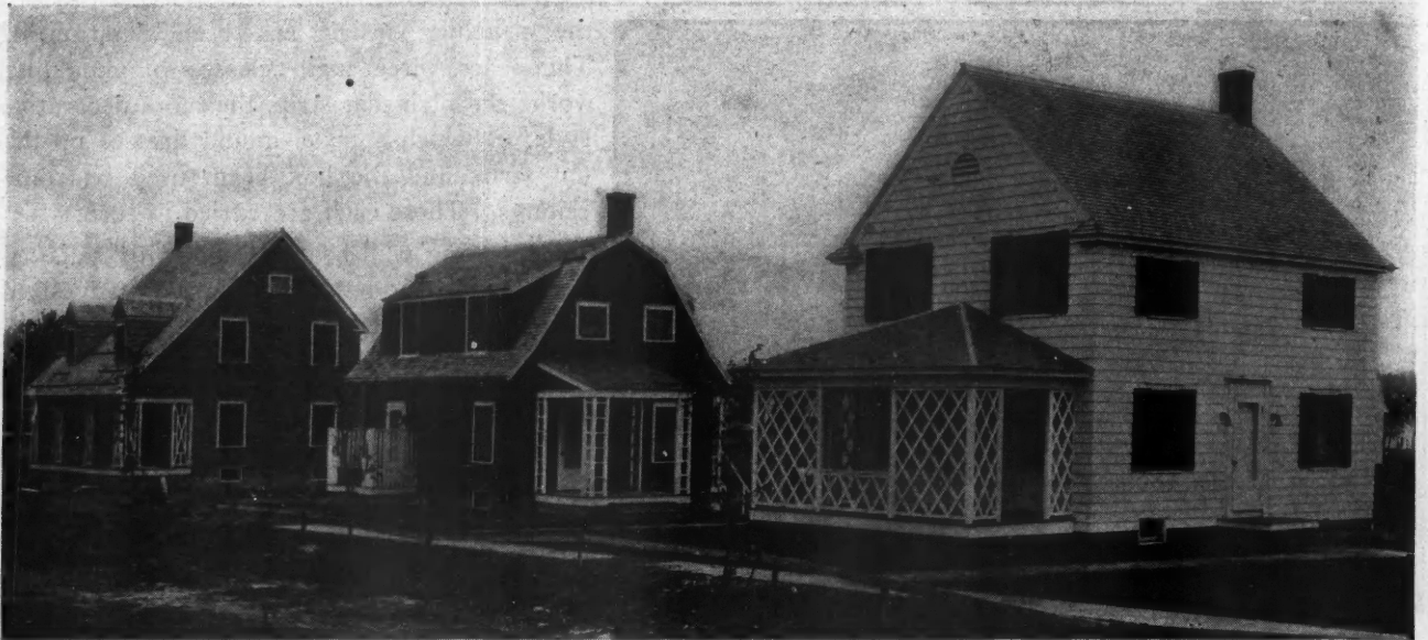
For the Colonial or Bungalow Types of Houses Shingles Lend a Touch of Quaint Beauty, and Are as Economical as They Are Attractive.
