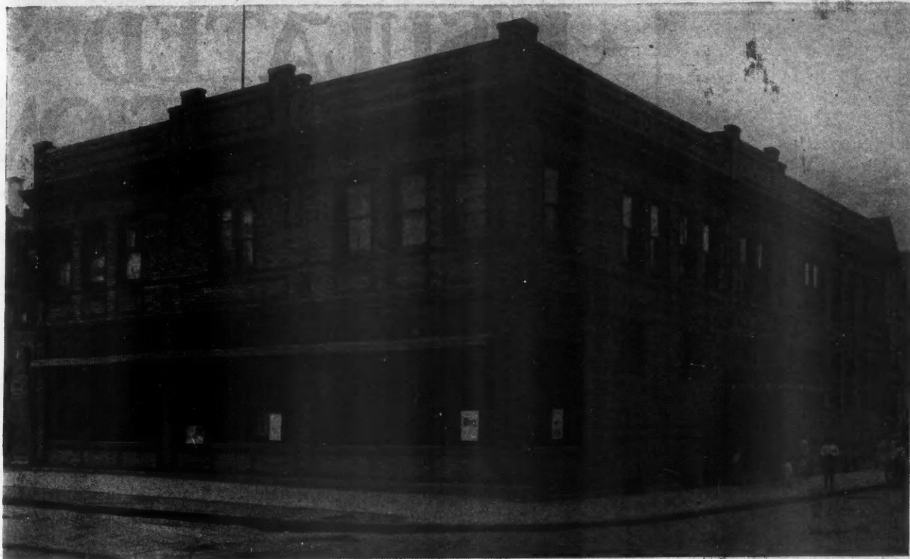
Lincoln Branch, Rochester Public Library. Entrance is in center of long side. The delivery desk is in the center, directly opposite the entrance. Shelving extends around the walls, with few floor cases. Adults' room is at the front; children's at the rear, divided by low shelving surmounted by a three-foot glass partition.
