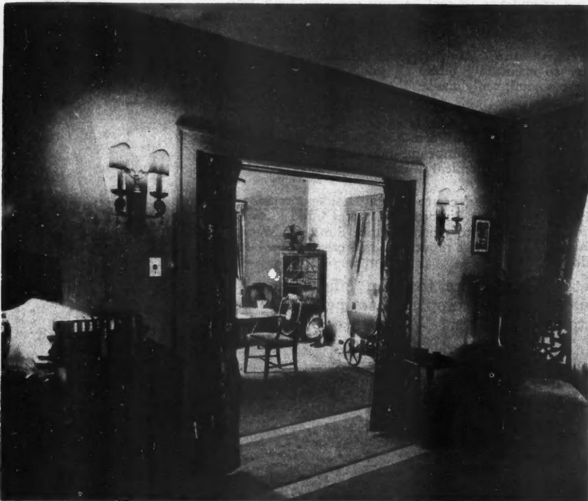
The Living Room Is Equipped with a Three-Way Switch for Controlling the Central Ceiling Fixture. The side-wall brackets are controlled from another switch alongside. There are two single and three duplex convenience outlets.
