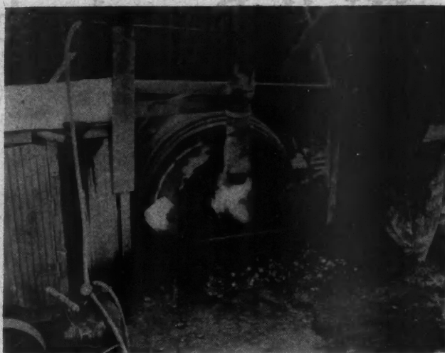
Heating the Concrete Aggregate with a Kerosene Torch Gives a Warmth Which Insures Perfect Set.
