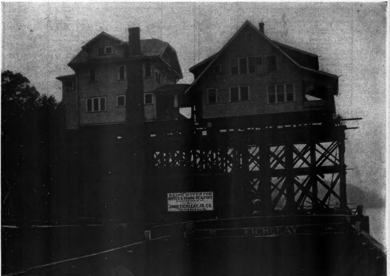
In Clearing the Site for the New State Capitol Building to Be Erected at Charleston, W. Va., It Became Necessary to Move Thirty Residences. Here is how they were ferried across the Kanawha River, furniture left in, and not even a crack in the plaster when placed on new sites.
