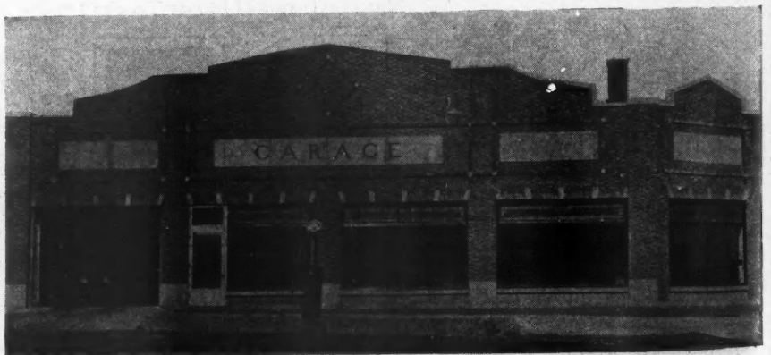
Since a Garage Must Cater to Passenger Cars and Trucks the Builder Must Make a Careful Analysis of Space Requirements Before Building.
