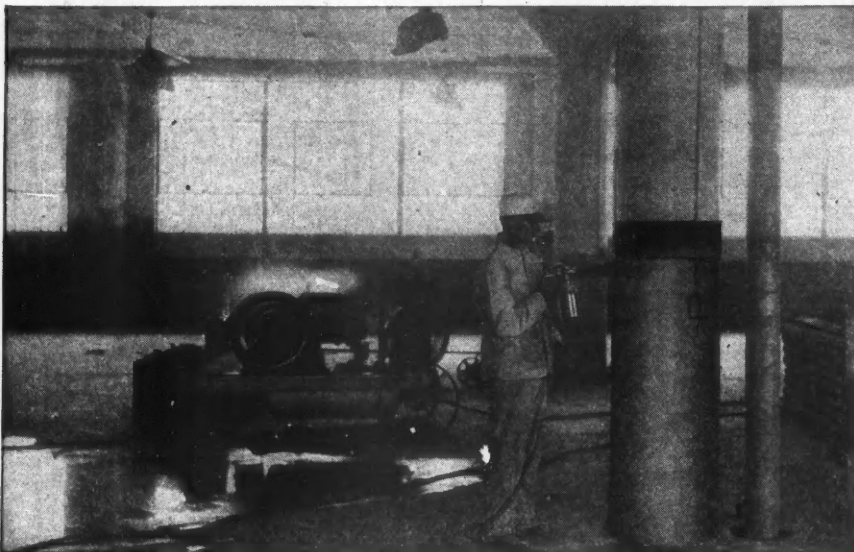
[Painting the dado—here the operator is using the DeVilbiss spray gun with Type [KN Pressure Feed Cup attached, which is advantageous on many kinds of work]
