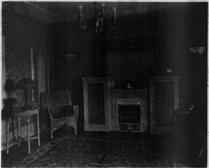
A Good Example of the Candle Type of Fixture. The convenience outlet in the baseboard is the most satisfactory way to light the portable lamp.
