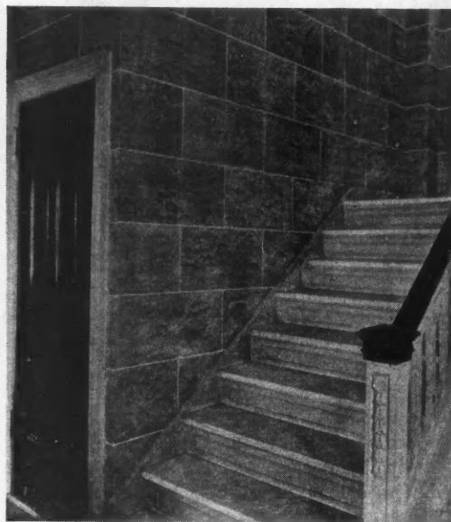
A view in the Halls and Stairway in the Clarendon Apartments, Riverside Drive and 86th Street, New York City, Chas. E. Birge, architect, William Randolph Hearst, owner, is shown above. Work installed by Vogel and Hase. Morene was applied over old painted surfaces roughly stippled, then flattened with a large pallet knife. When partly set, it was lined off with sunken joints.
