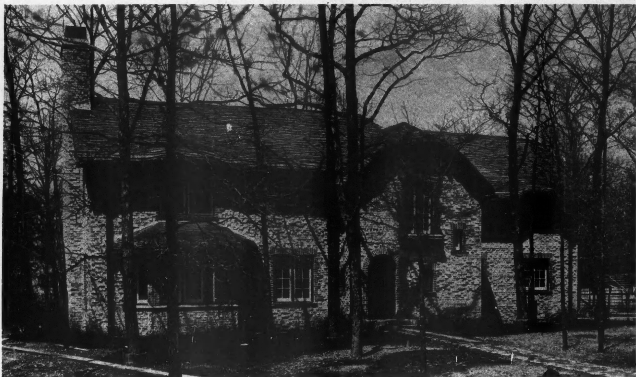
It Is Not Necessary to Go Abroad for Picturesqueness. Here is a home of common brick built in an exclusive Chicago suburb which possesses every element that makes for picturesqueness and genuine interior comfort. The Staggered brick wall was specified by Chatten & Nammond, of Chicago, the architects.
