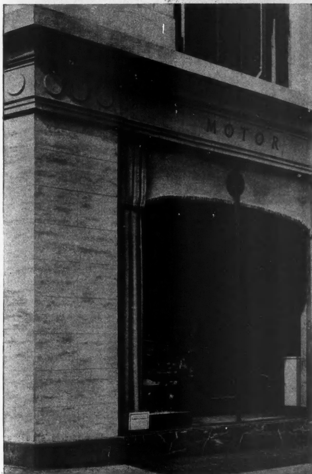
A Light First Coat, a Heavy Second Coat, a Blowing on of Sand, a Lining Off with Sunken Joints, and This Handsome Corner Resulted.
