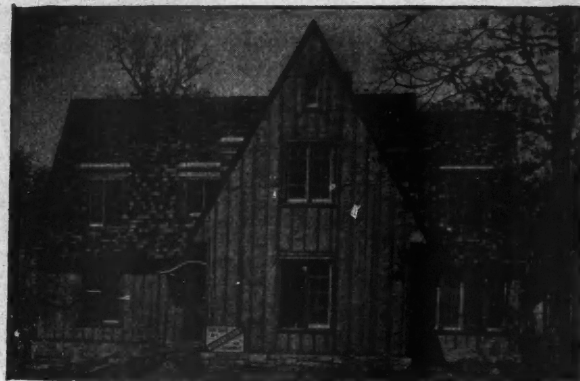
Houses near Chicago, showing the "underclothing" of Cabot's Quilt, with furring strips over the Quilt, on which the outside finish is laid. Roof also insulated. Leon E. Stanhope, Architect, Chicago
