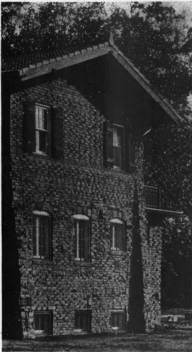
Not Hard to Understand the Rustic Appeal of this House with Its Staggered Brick Giving Fine Play of Light and Shadow.
