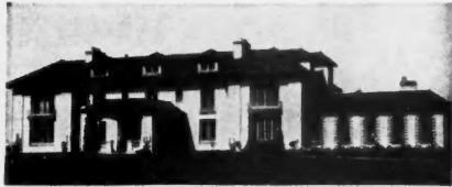
RESIDENCE SENATOR GEO. S. NIXON, RENO, NEVADA. EDWARDS METAL SPANISH TILE USED ON THIS BUILDING
