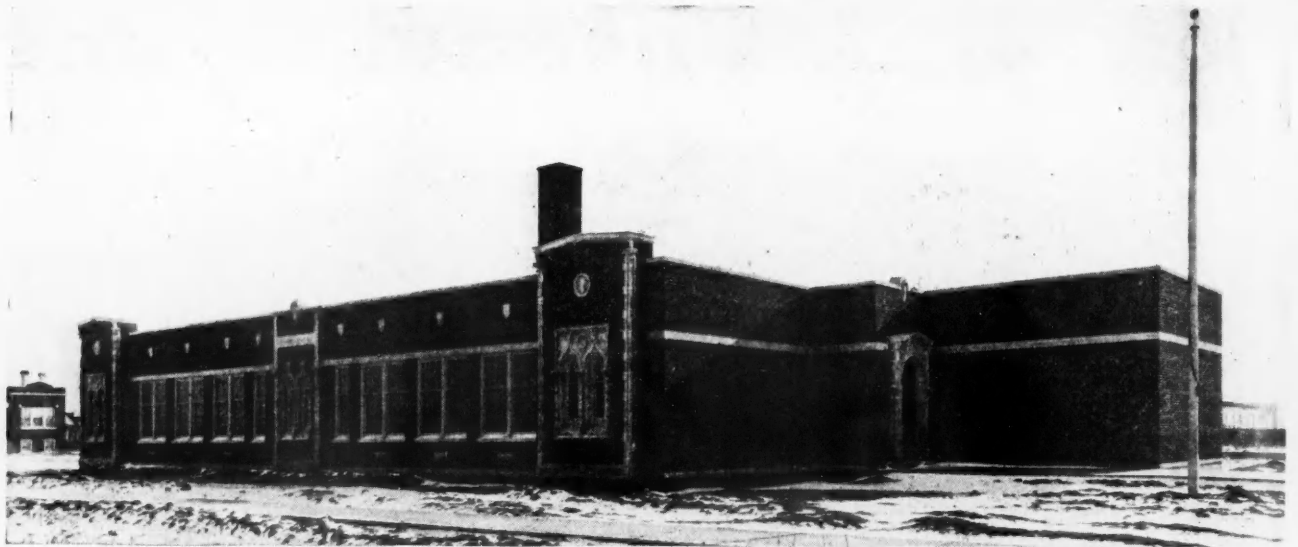
The Komensky Grade School, Berwyn, Ill., Is a Good Example of the Modern Trend of Schoolhouse Construction. It is of Romanesque architecture. The exterior is of warm colored rough texture shale brick with Bedford cut stone trimmings. It contains six classrooms and the boiler room and the coal room are on the ground floor—no basement.
