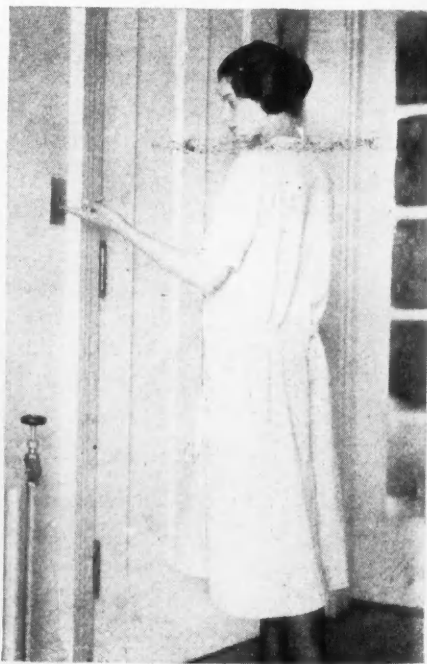
Convenience Outlets Make It Possible to Have the Reading Lamp at the Head of the Bed, and to Use the Various Appliances Shown. Note the outlet beside the bureau; its height makes it easy to use. And in the illustration at the right observe that the location of the switch is important; this one is behind the door, and therefore most unhandy.
