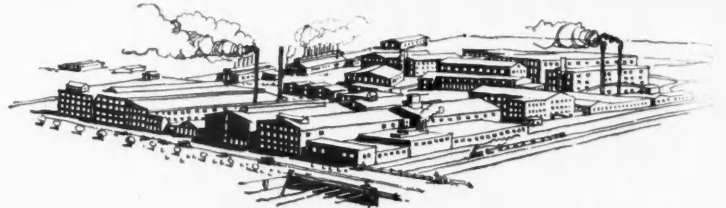
Plant No. 15—Philadelphia, Pa. Began making floor coverings nearly a hundred years ago as Thos. Potter Sons & Co., Inc. Its products have been widely known and used for several generations. Today is producing tremendous quantities of plain and inlaid linoleums, printed linoleums, Floortex (felt base floor covering), and oilcloth.
