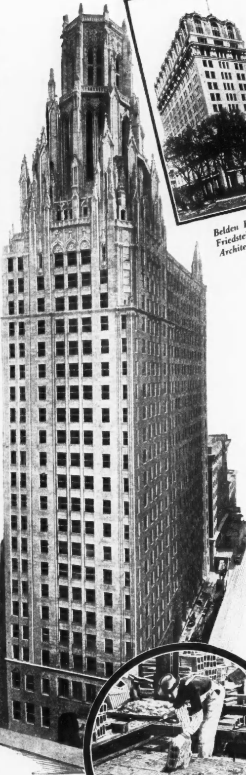
Temple Bldg., Chicago, Holabird & Roche, Chi. Architects
