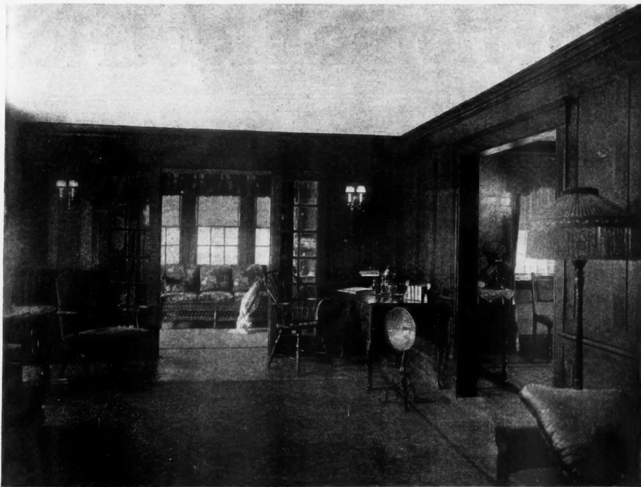
In This Living Room Illumination Is Furnished Entirely from Side-Wall Brackets and Portable Lamps. There Is No Central Ceiling Fixture Used.
