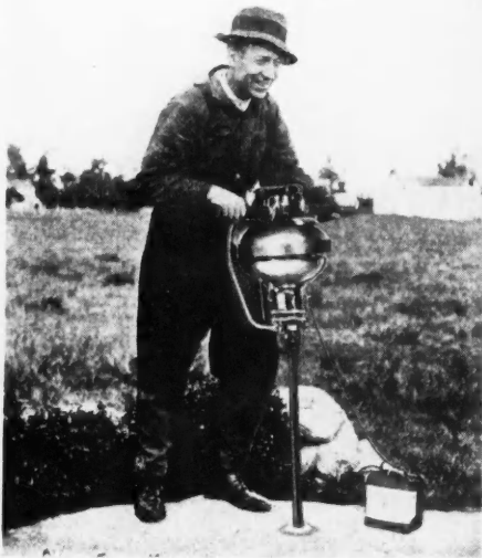
Upper Right Illustration Shows Gasoline Hammer Drill Used for Ramming Back Fill. Lower Left Shows Complete Drilling Unit Operating.
