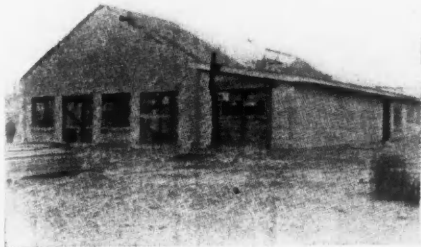
View showing ACME INTERLOCKING TILE being used by New Jersey State Prison Department in Construction of this building.
