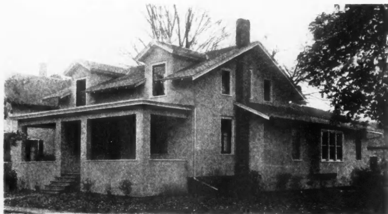
House Finished with Magnesite Stucco. Magnesite Is a Nonconductor of Heat and Cold; Keeps House Warm in Winter, Cool in Summer.
