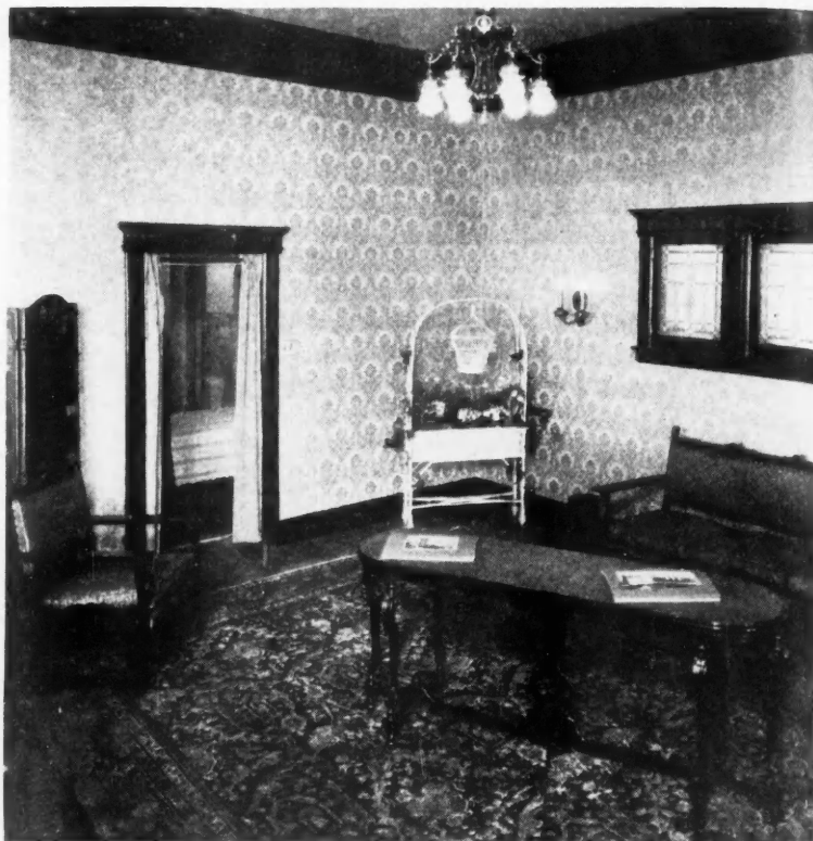
This Living Room Had the Walls Finished in Special Practice Plaster and Then Sized and Covered with a Fabric Finished in Oil Colors Made Especially for Use on Walls.
