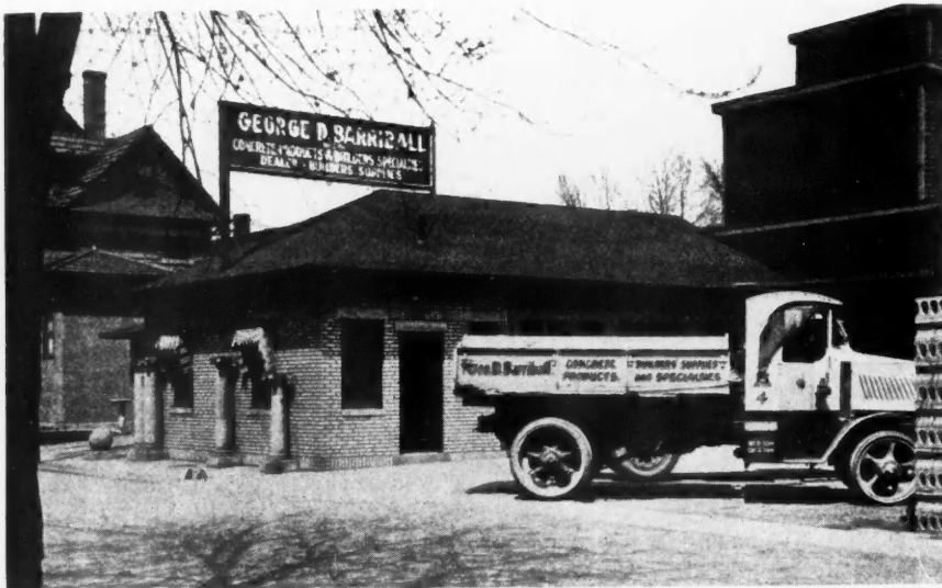
Gentlemen, Meet George Barriball's Concrete Products Yard, Cleveland. Mr. Barriball is noted as the neatest manufacturer in the business.
