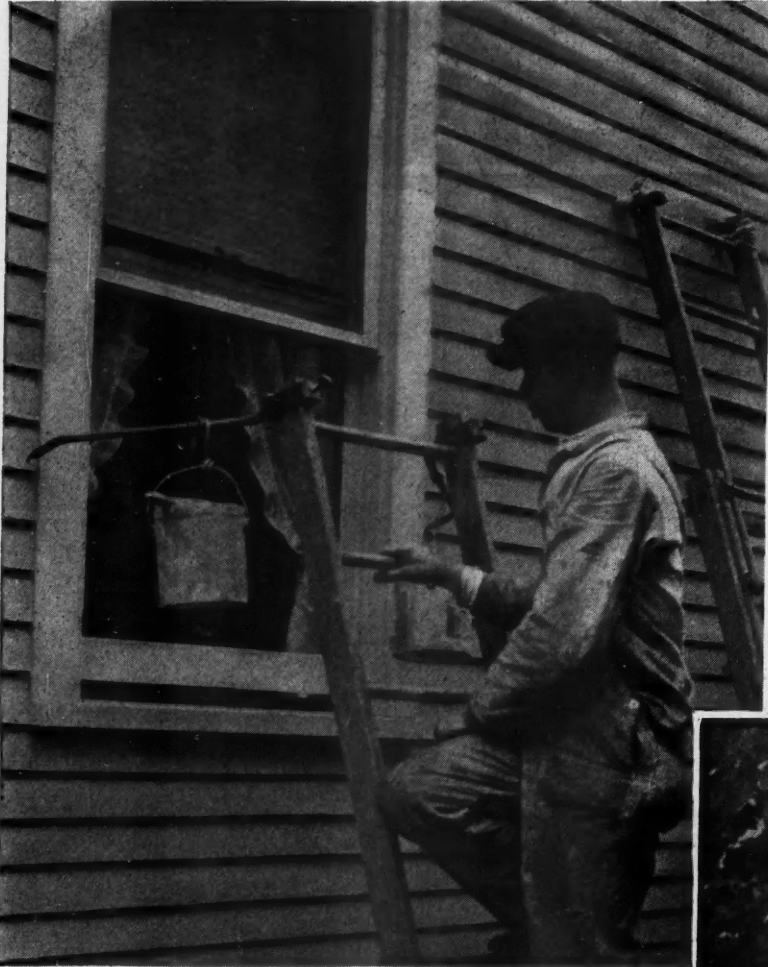
The New Safety Arm or Bracket Holds the Ladder Safely and Securely, Gives Good Working Space and Radius, and Insures a Good, Careful Job.
