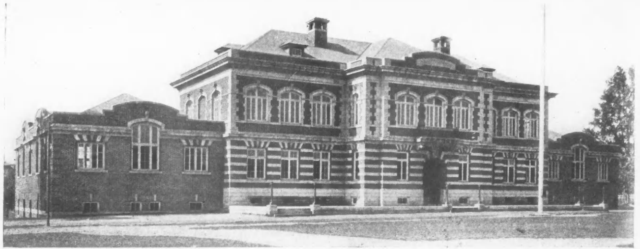
The Recreational Building of the Kingsessing Playground, Philadelphia, Philip H. Johnson, Architect. It has two stories and a basement with body of brick and cornices of terra cotta. Base is of granite as are also the copings.
