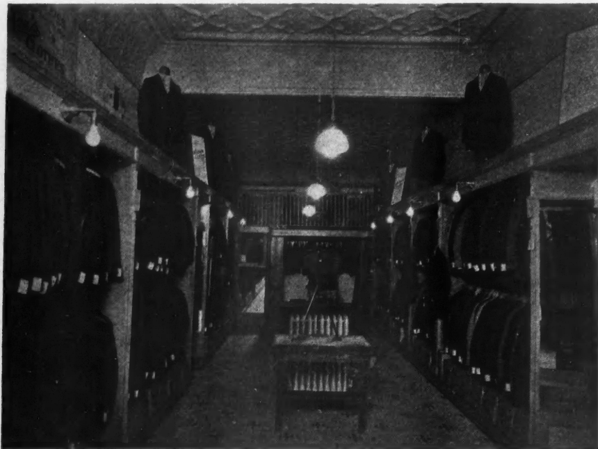
Fig. 3. The Single Row of Units in the Long Narrow Room as Pictured Here Is Generally Satisfactory. This employs a glass encircling globe and provides ample illumination, with the side brackets playing an important part in centering attention on the displays.
