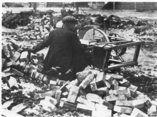
He Cleans the Mortar Off Bricks After a Fire, Salvaging an Average of 5,000 Bricks a Day.
