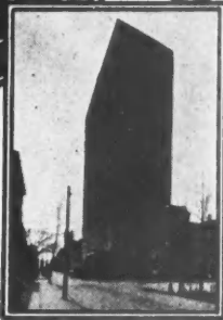
Rittenhouse Square Apartment House, Phila., Pa. Architects McIlvain & Roberts, Phila., Pa. Gen. Contractors, Metzger, Fisher and White, Phila., Pa.
