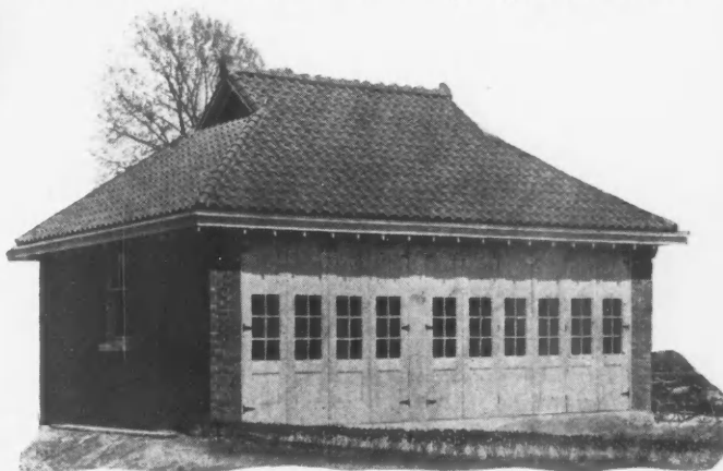
A Pleasing Design, Three-Car Capacity. Brick walls and tile roof make a very durable, substantial structure. This garage was built to match a residence.
