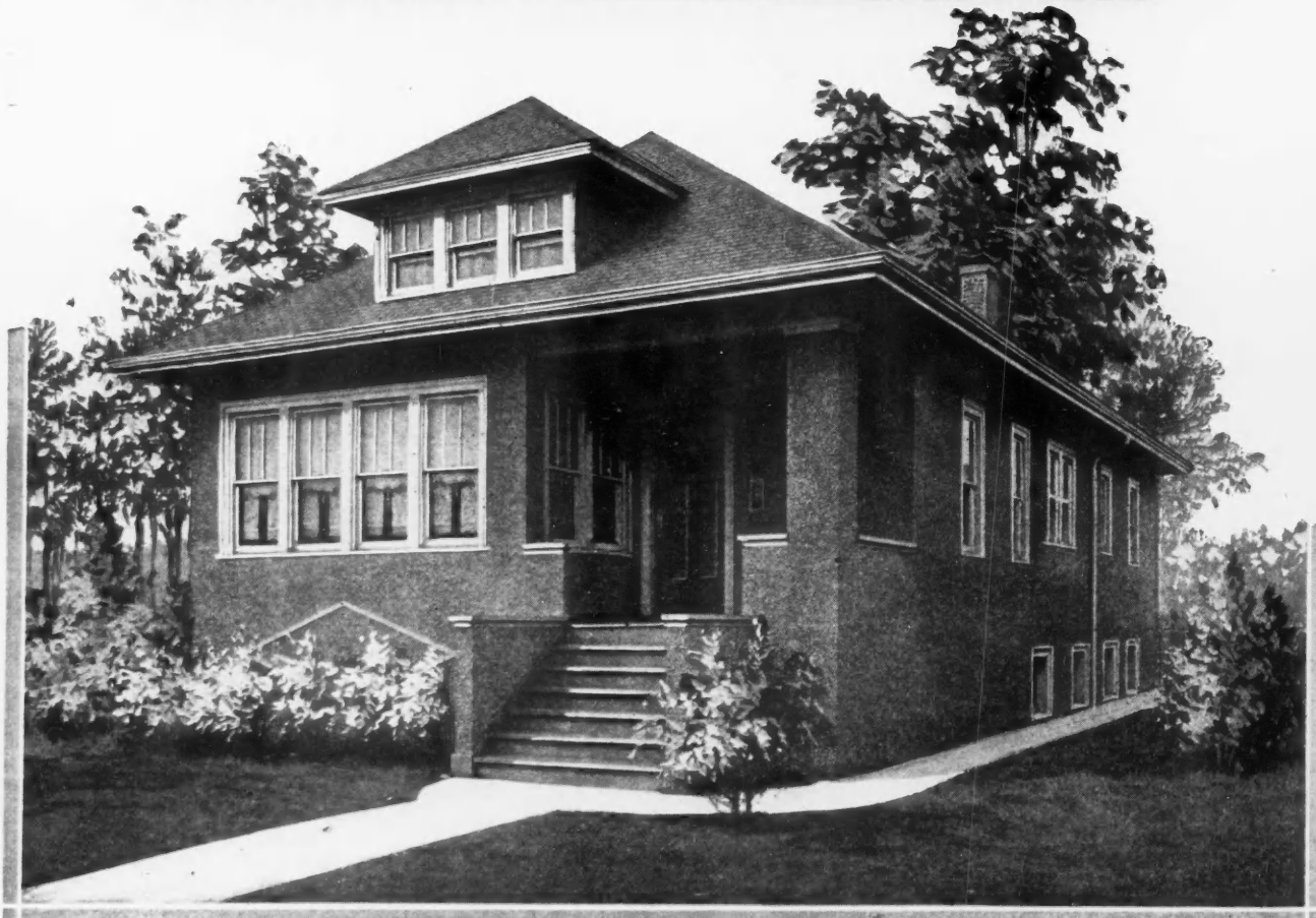
ATTRACTIVE AND ECONOMICAL STUCCO HOME. This residence is especially designed for home-seekers preferring a stucco house that is cozy and compact. It has a conservative and substantial appearance. The rooms are all large and comfortable and the interior arrangement is very pleasing and convenient. One particularly desirable feature that will appeal to the housewife is the breakfast room located directly between the kitchen and dining room. From the porch one enters a vestibule, half of which is converted into a coat closet. Directly ahead is the dining room. The breakfast room and kitchen are also on this side of the house. The living room joins the vestibule by cased opening directly to the left. It is very modern with a fireplace, seat and built-in book cases. The two bedrooms and bath occupy the rest of this side of the house.
