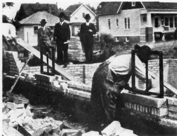
Fig. 1. Steel Windows Being Installed in Brick Veneer. Windows may be built in either before or after veneer is put up.
