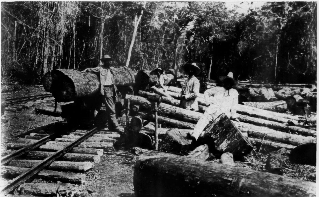
A Few of the Larger Logging Companies Have Installed Modern Methods and Handle Their Mahogany Logs from Forest to Tidewater on a Narrow Gauge Railway. This photo is of the operations in Campecho, center of the Mexican mahogany industry.
