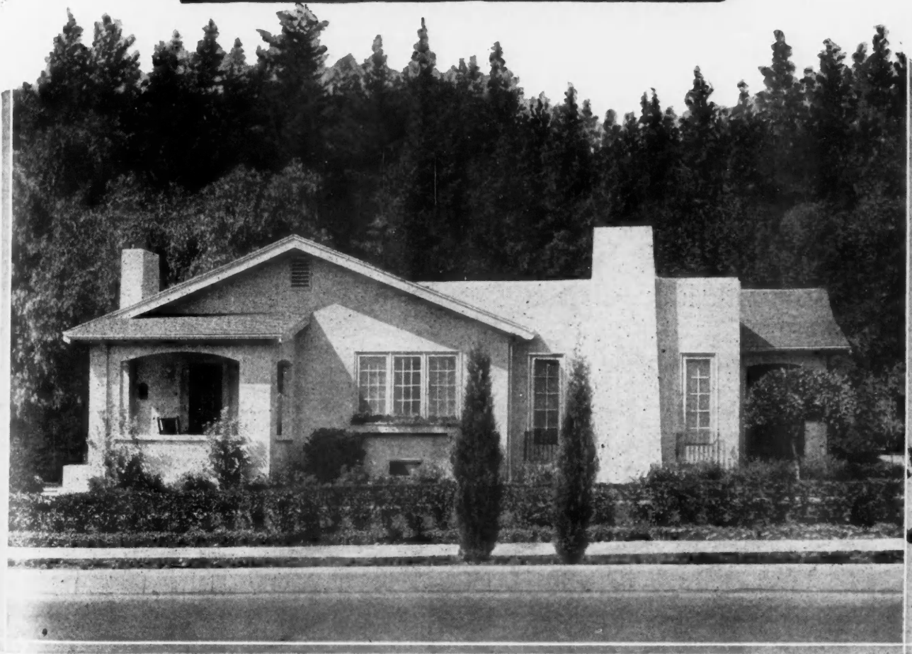
ATTRACTIVE DUPLEX BUNGALOW. For those who seek additional income from their property and prefer the western style of architecture this double-house with four rooms and bath in each home will particularly appeal. Both sides of the house are planned along the lines of an apartment. The exterior is of stucco and the exposed parts of roof shingles. A pleasing effect has been worked in with the stucco finish and flat roof. The two porches indicate the front entrances. The living room is entered from the porch in both homes. In addition there is a dining room, bed room, kitchen and bath in each flat. In the left one a wall bed opening into the living room has been provided, making two bedrooms in this apartment. The building is 56 feet 6 inches wide and 36 feet deep. The rooms are all of comfortable and convenient size and are well lighted, ventilated and heated.
