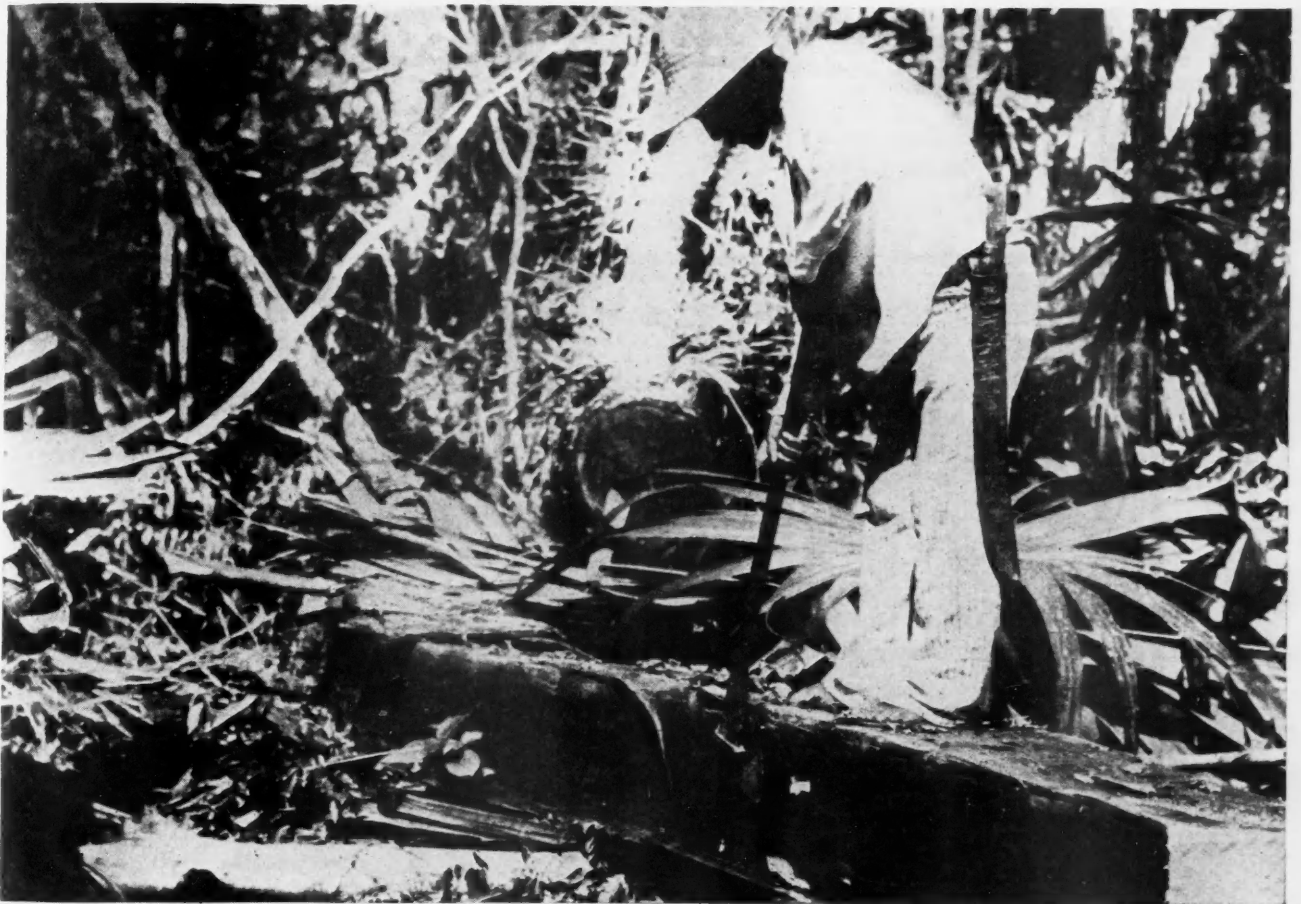
These Peon Workmen, Laboring for Next to Nothing and Under Most Trying Conditions, Become Highly Expert in the Use of Their Long Axes. They square the mahogany timber to exact size and with surprising accuracy.
