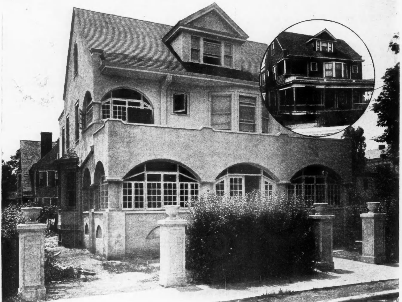
Hard to Believe Such a Change Is Possible. The house in the circle is the same house before it was "overcoated" with stucco. It is located in Brooklyn.
