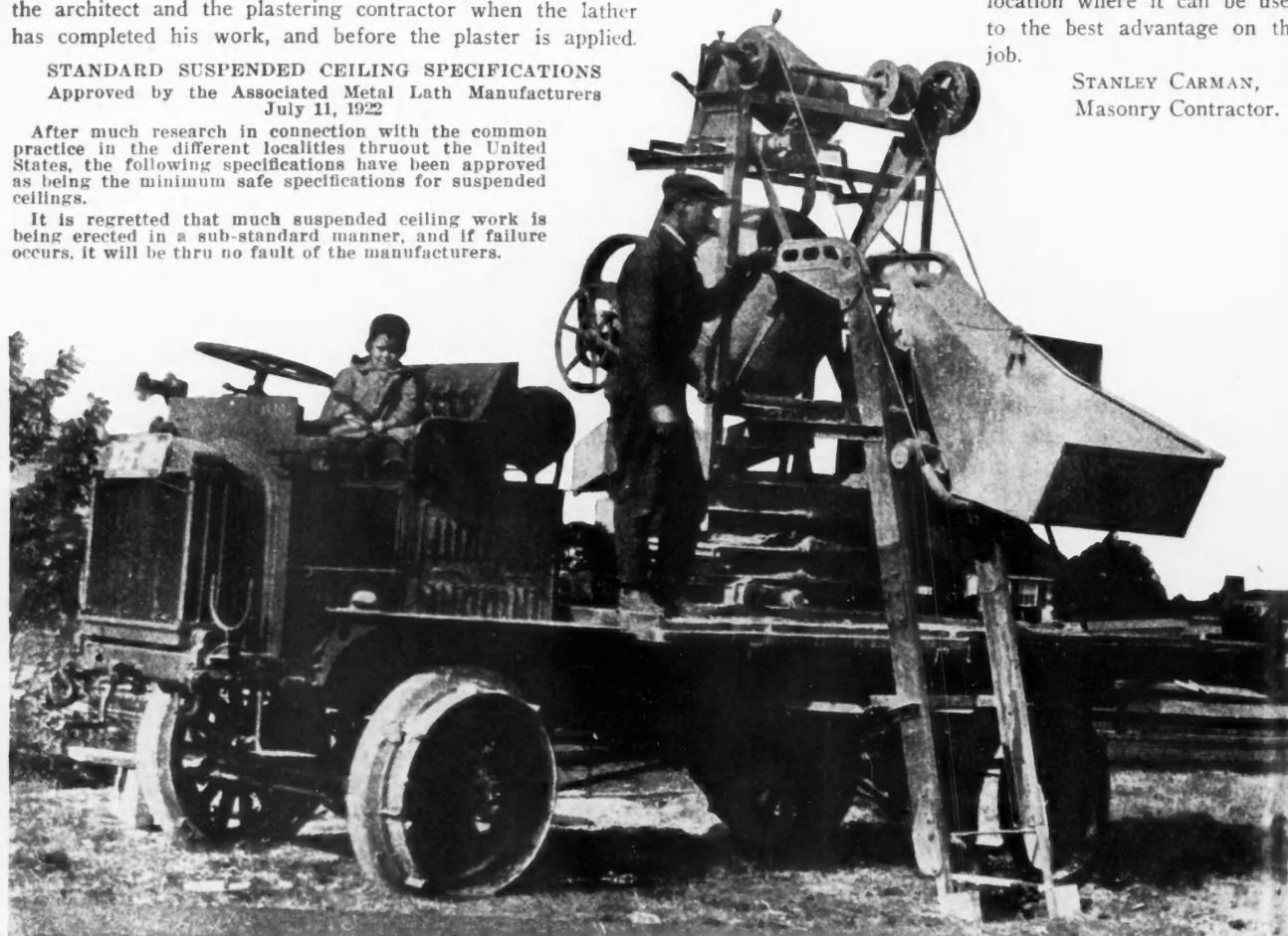
The Concrete Mixer Is Mounted on an Auto Truck. It facilitates moving the mixer for all that is necessary is crank the truck and drive away to the next job. Mr. Carman has put 10-inch steel flanges on the front wheels of the truck and 12-inch flanges on the rear wheels which enables the truck to go over soft ground.
