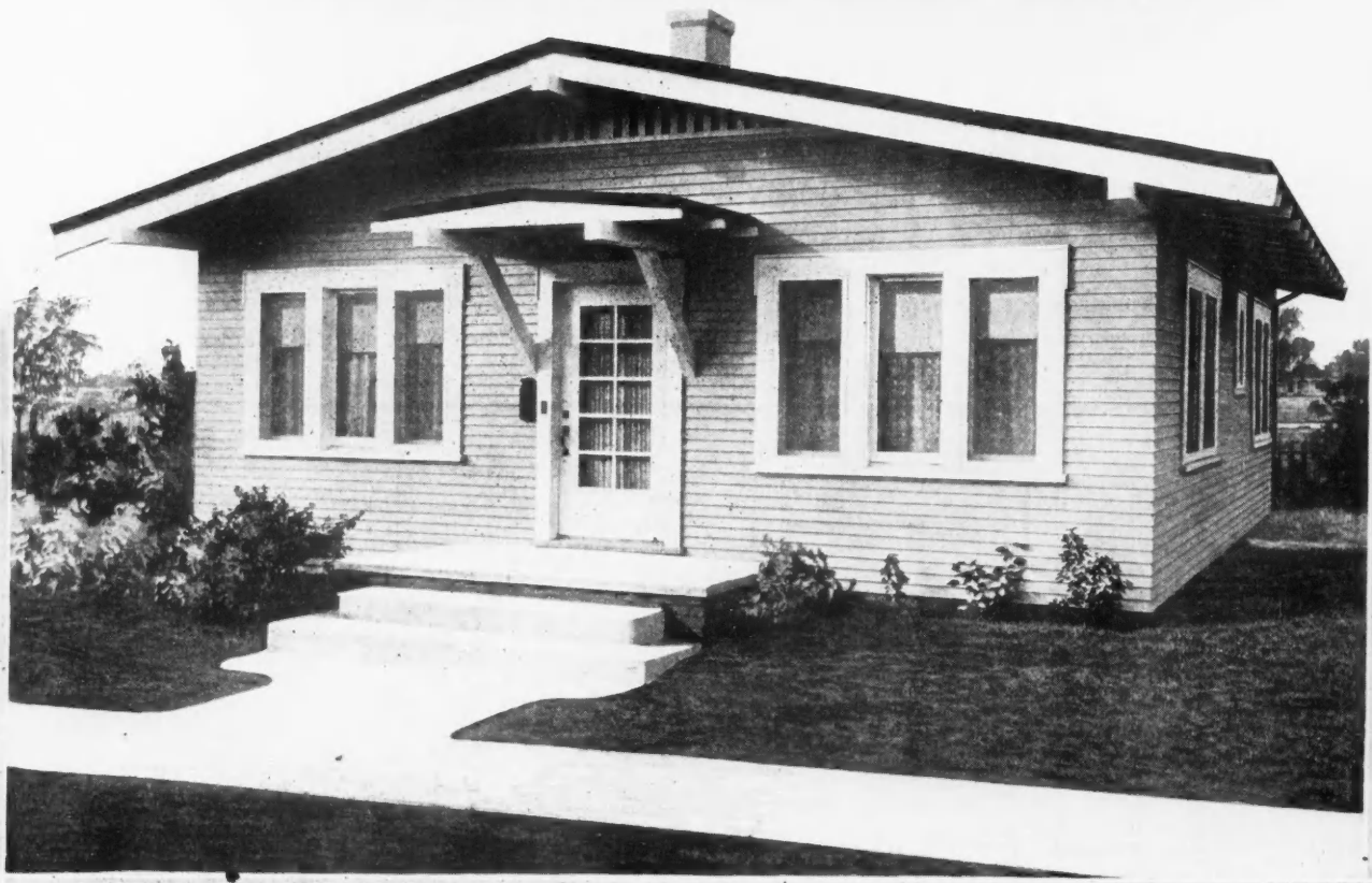
A COZY BUNGALOW FOR A SMALL FAMILY. The fact that this 5-room home is set close to the ground, built up but one story, finished with narrow clapboard sidewalls and heavy eaves supported by extended beams, is an assurance of its bungalow nativity. The designer has sought a departure from the customary by adopting some very attractive colonial features. Note the front entrance, the platform with the colonial hood over the front door. The front windows are built in well, giving an abundance of light to both the living room and front bedroom. The living room is entered from the front door. Directly back of the living room is the dining room. The kitchen is also at the rear.
