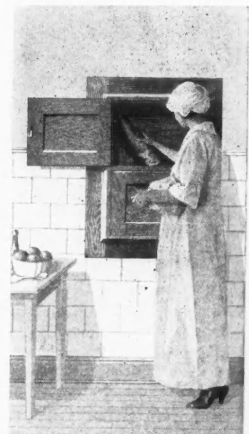
Built-in Receivers Solve the Delivery Problem for Housekeepers.
