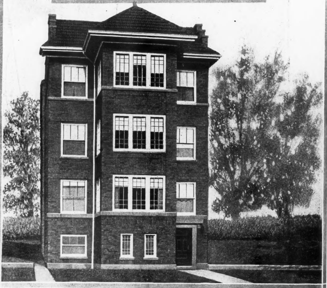
MODERN THREE-APARTMENT BUILDING. The sun parlor, which has come to be one of the most important features of the modern apartment, is prominent in this building. It is further enhanced by an ornamental hip roof of green tile which is also used for the main roof. Among the popular developments in apartment construction in the last few years is the living room extending the full width of the house as shown in the floor plan here. Each apartment contains five rooms, of which two are bedrooms conveniently located on one side of the apartment, with bath adjacent. This building is constructed on a narrow lot, being 28 feet wide by 56 feet long.
