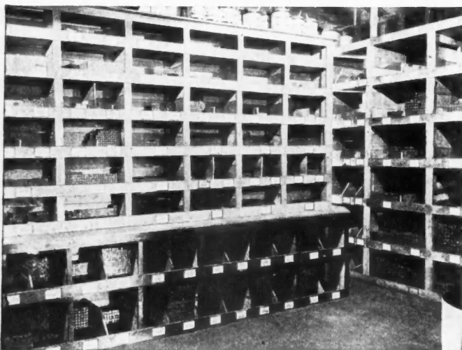
Orderly Arrangement of the Cadillac Building Construction Stock Room Saved Time and Stopped Losses.
