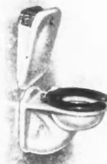
Wall Tank Opened to Reach Flushing Apparatus.
