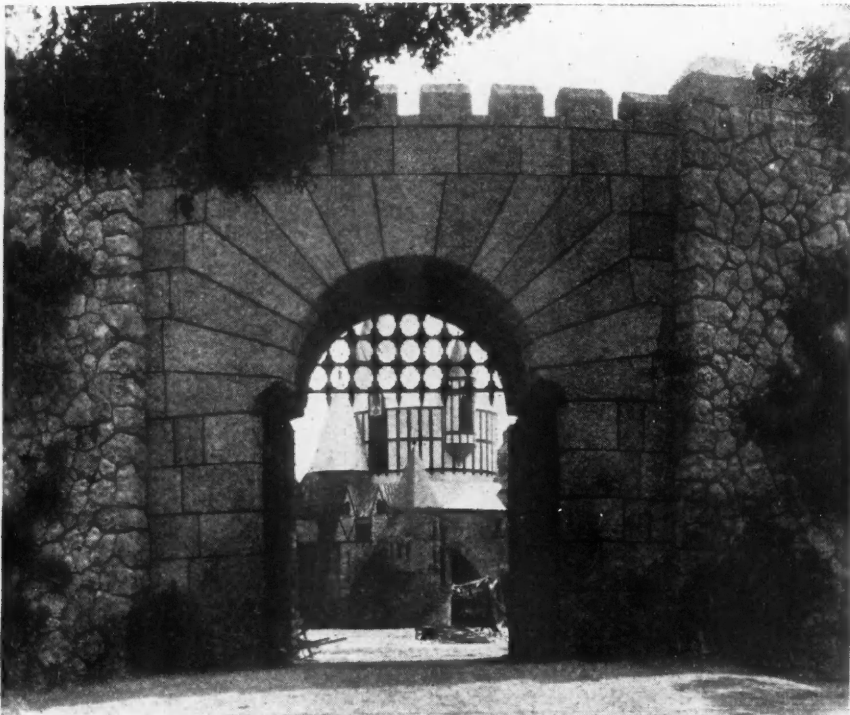
Massive Wall and Gateway Built to Imitate Stone Perfectly Is One of the Interesting Construction Features of the "Robin Hood" Scenery.
