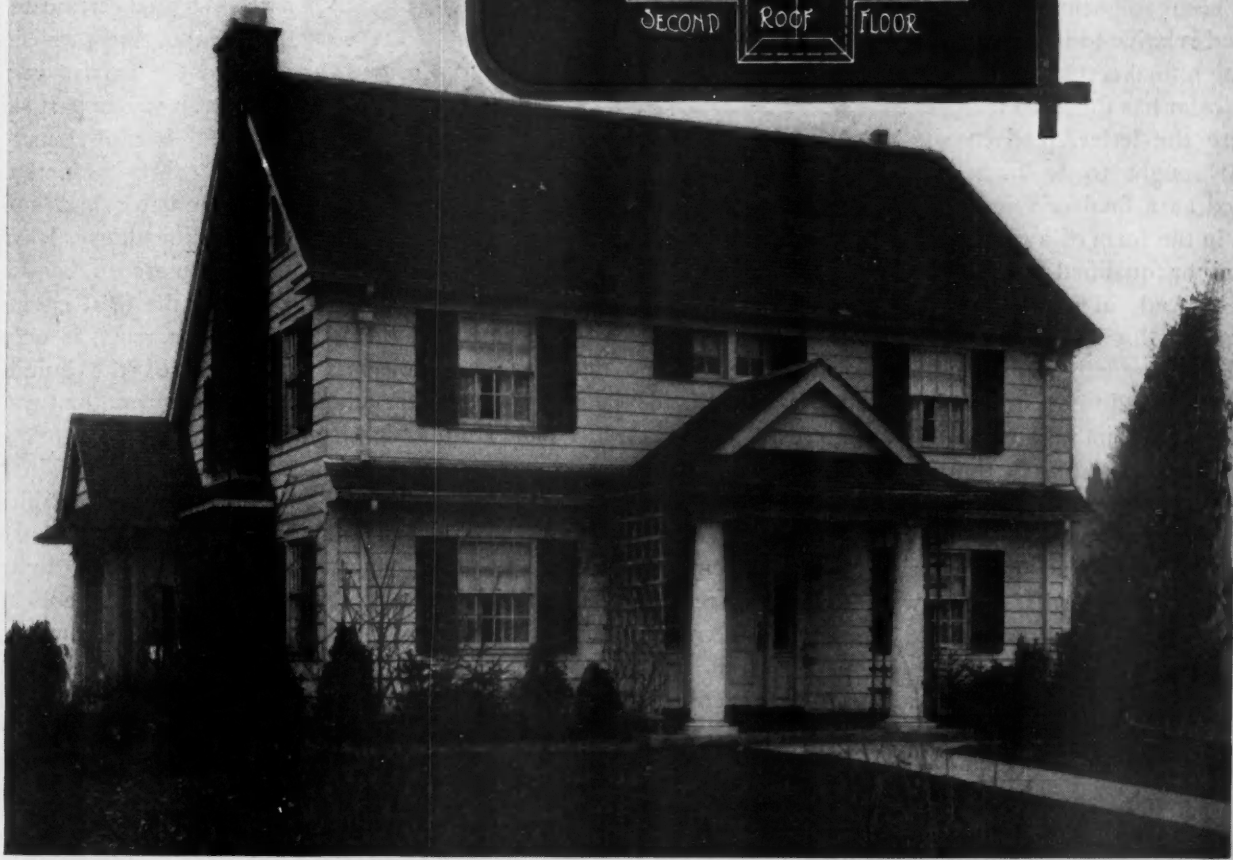
SPACIOUS COLONIAL HOUSE OF SEVEN ROOMS. Expressing as it so eloquently does hospitality and substantial comfort, this house will continue to hold its appeal in the years to come just as it has done for the last century. There is something irresistible about the white clapboard siding, green shutters, small pane windows and delightful entrance. In this case the front door has been shielded by the addition of a small roof supported by large white columns and embellished still further by lattice sides. On the first floor are the three main rooms, living room, dining room and kitchen and a sun porch in the rear. The rooms are all designed with comfort as the main object. Upstairs are three bedrooms, the side bedroom being larger than the other two and connected directly with the bathroom. A small alcove is built at the end of the hall. Size of house, 36 by 26 feet.
