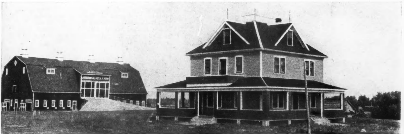
Attractive Farm Building Group Recently Erected by A. F. Allshire, Canadian Builder, Manitoba, Canada. The House Is 30 by 34 Feet, With Modern Conveniences, and the Barn Is 56 by 96 Feet.
