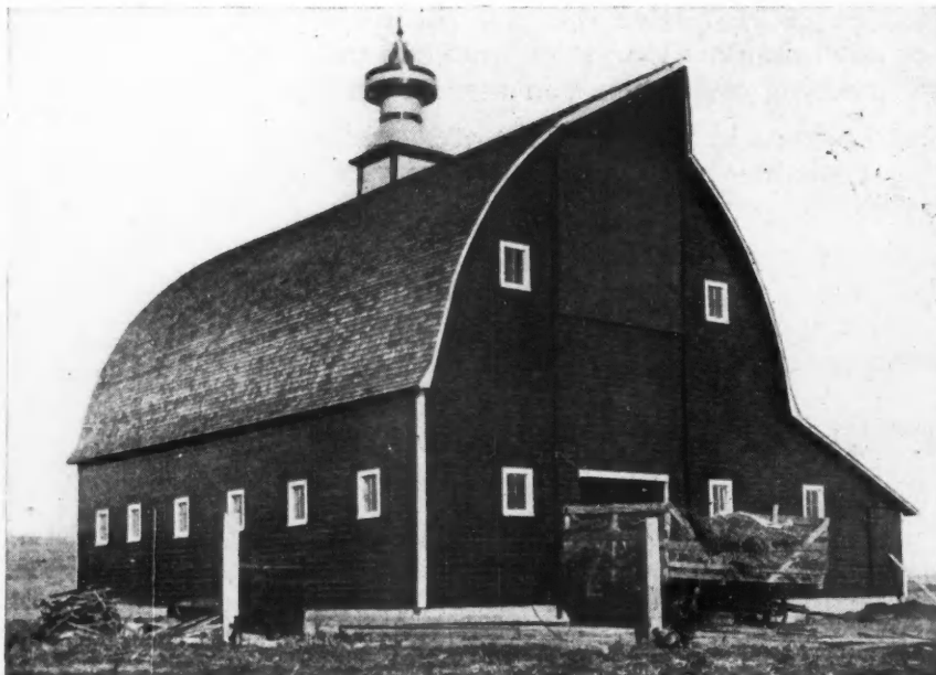
Out in Poole, Neb., W. M. Eggleston, Contractor and Builder, Writes They Are Strong for Gothic Roofs, Even on Hog Houses. He Wants Some Brother Builders to Send Some Pictures if they Have Any.
