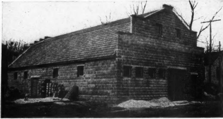
New Plant of Milltown Concrete Co., Milltown, Ind. This Was Built of Blocks Made by the Company and the Entire Building Was Erected by Three Men.
