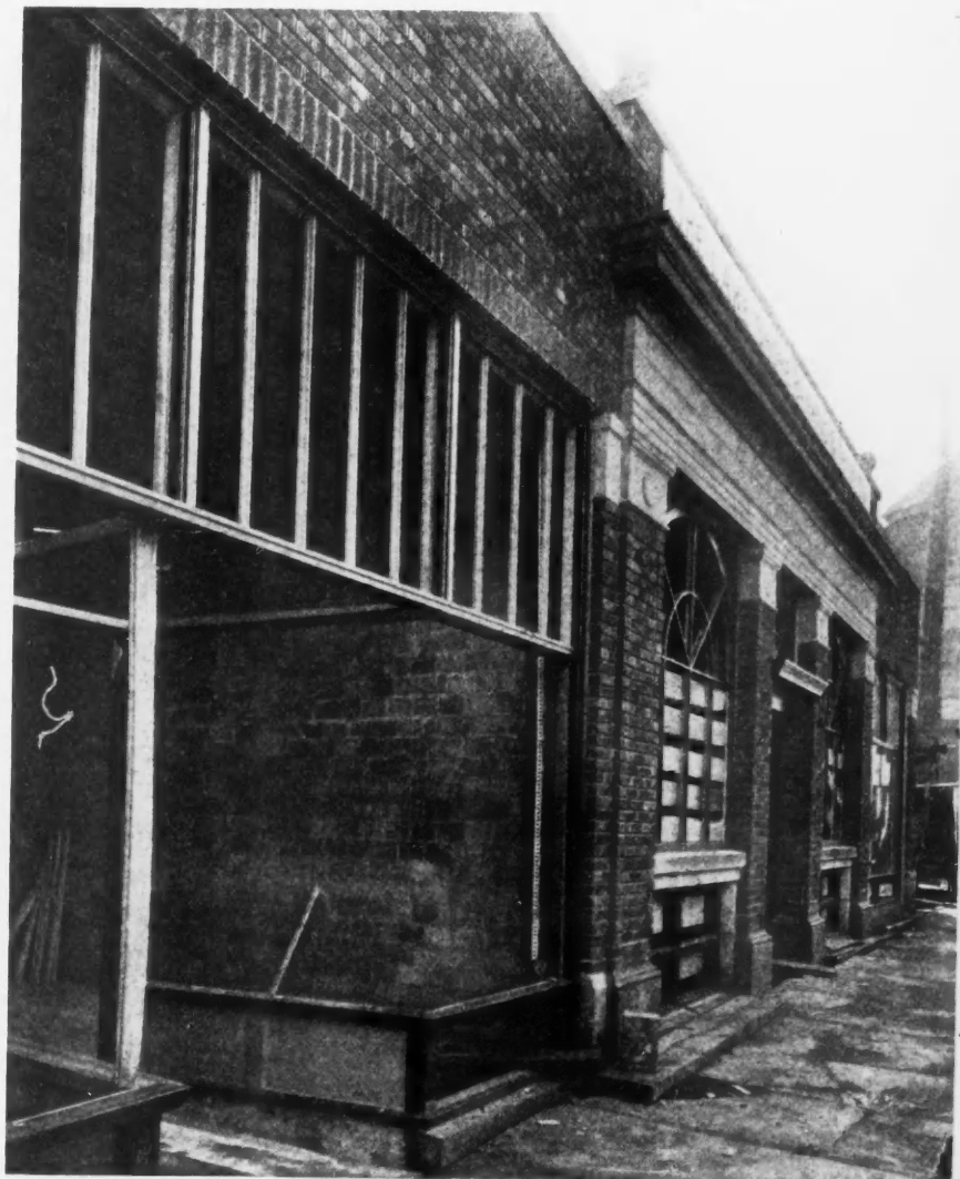
New Store and Bank Building in Cleveland, Ohio, Constructed of Concrete Tile with Brick Veneer. This Building Is 84 by 68 Feet 2½ Inches. Architect, E. R. Russell.
