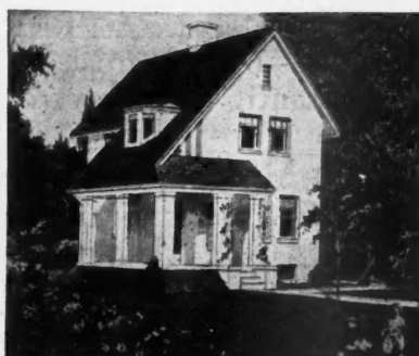
Two-Story Residence No. 1184
