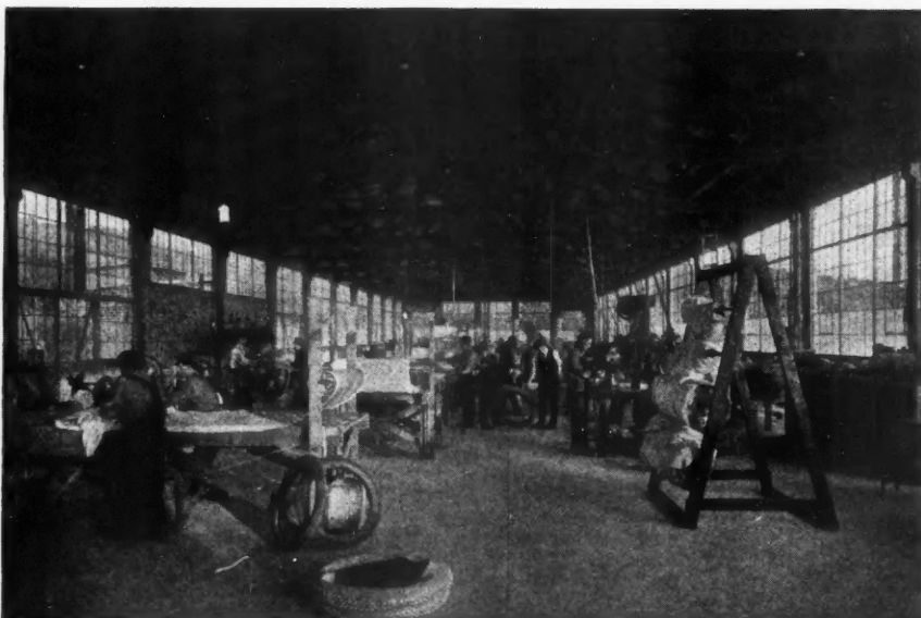
There is Little Need of Artificial Lighting in This Workshop. The Sunshine Pours in from Both Sides and Provides a Soothing Efficient Light for the Workmen.
