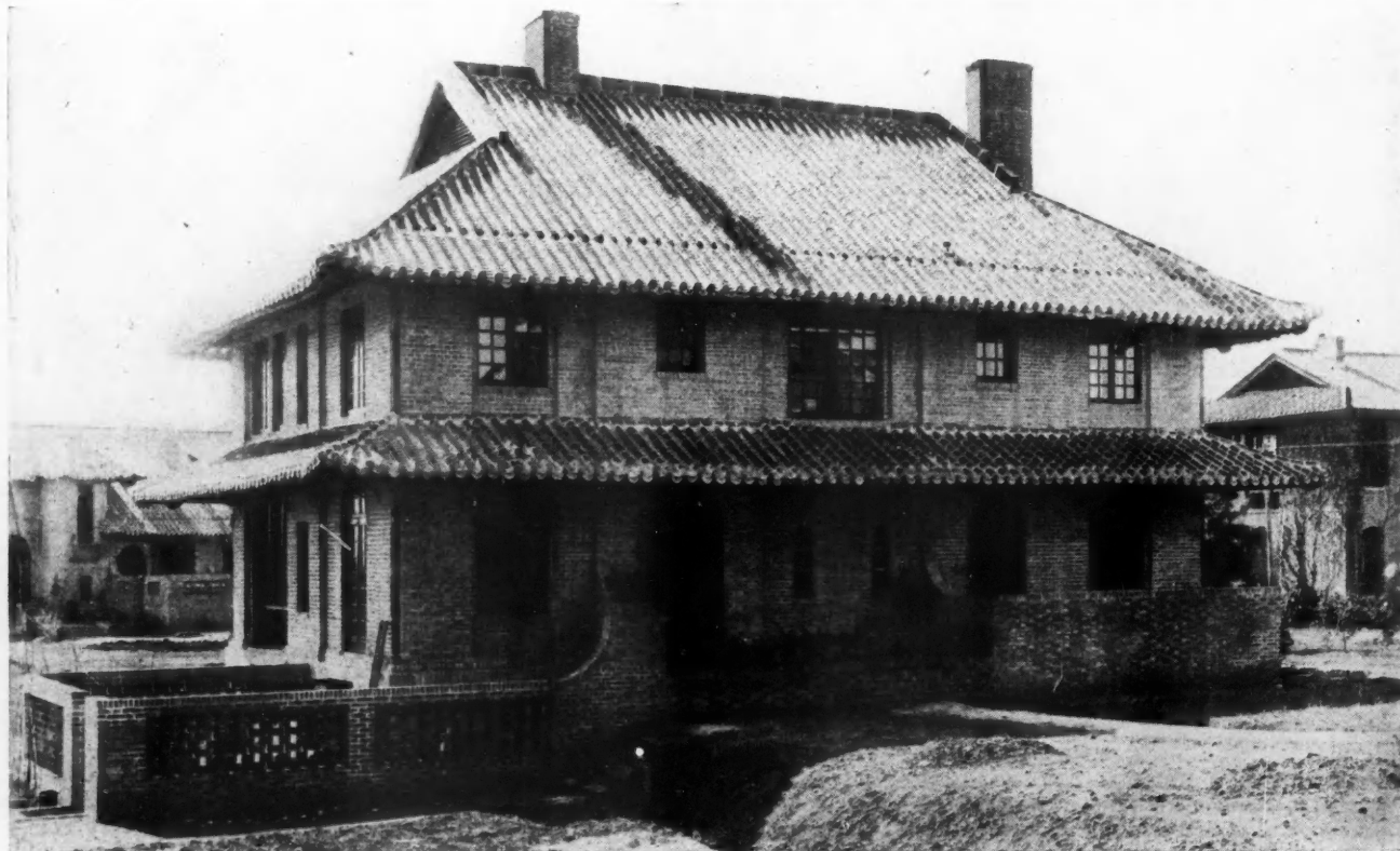
Professor's Home, One of the Buildings of the Canton Christian College, Canton, China. Only the Roof Lines and the Heavy Tile Roofs Show the Chinese Building Style, the Balance Being Typically American Brick Construction.
