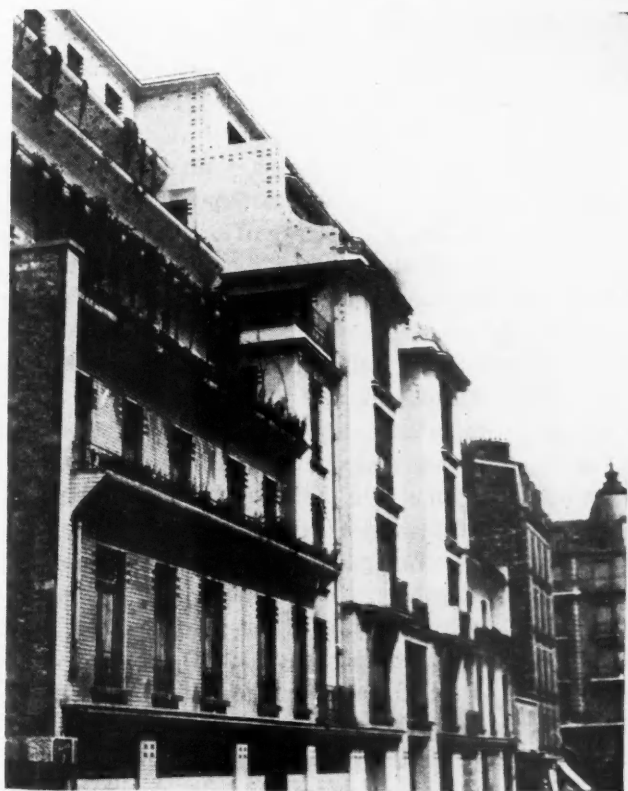
Front of Apartment Building Showing How Each Floor Recedes Giving the First Floor Apartment Ten Rooms and the Top One Four.
