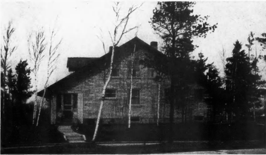
Fig. 11. Attractive Bungalow at Morgan Park, Minn., One of Several Hundred Houses Constructed of Single Wall Concrete Block as Described in the Accompanying Article.
