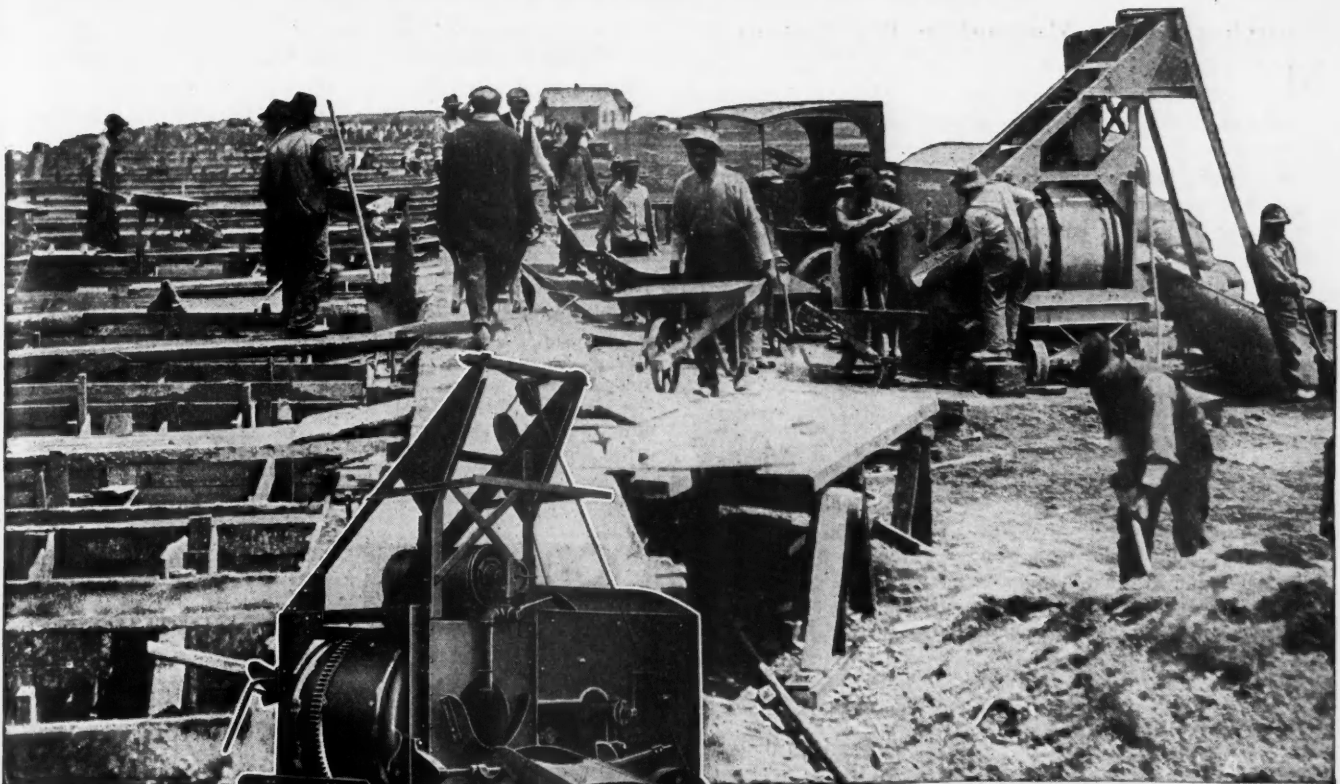
To the left is a No. 10 Lansing Mixer with power side loader, water tank and gasoline motor power. The automatic water tank is of the enclosed pressure type, with 20-gallon capacity.
