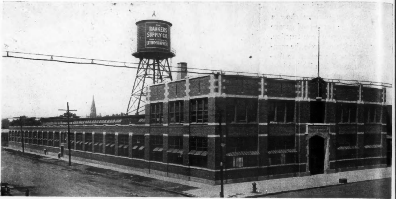
Recently Completed Factory of Bankers Supply Company, Chicago, Designed by Shankland & Pingrey, Chicago, Architects and Engineers. It Demonstrates the Effective Use of the Window Wall or Steel Sash in a Monitor Roof Type Daylight Factory.
