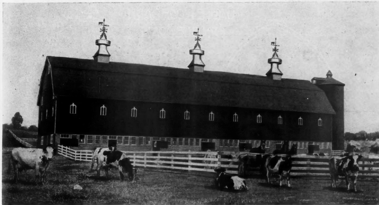
Familiar Gambrel Roof Barn. The Gambrel Roof Is Used Extensively in All Parts of the Country and Has Many Advantages, the Most Important Being Its Strength. Details of Gambrel Roof Are Shown on the Next Page in Blueprinted Form.
