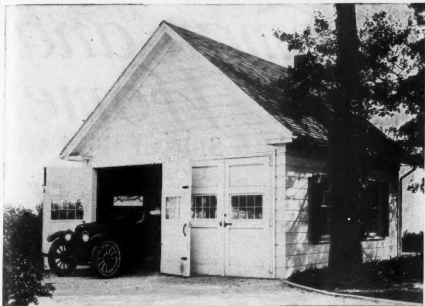
Fine Farm Garage with Two-Car Capacity and Double Hinged Doors. It Is Built to Harmonize with Colonial House. Note Side Windows and Shutters.
