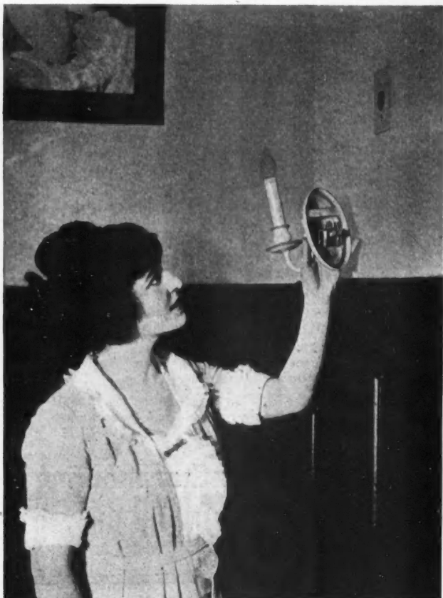
Wall Bracket About to Be Installed in New Wall Outlet Placed at Intervals Around the House. These Small Outlets Permit the Fixtures to Be Moved at Will Without Wall Damage and Extra Expense.
