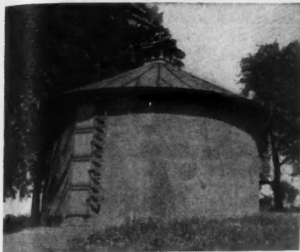
Circular Farm Ice House Built with Steel Silo Forms. Such Ice Houses Are Economical and Almost Indispensable on the Modern Farm, and Should Furnish Silo Contractors with a Considerable Volume of Business.
