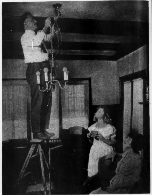
Same Flexible Outlet Designed for Ceiling Fixtures. The Fixtures Are Attached by Means of Two Prongs Which Provide the Contact.
