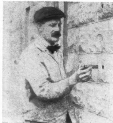
Inserting the Expansion Shell. This Little Device Is Very Valuable to Builders for Fastening Accessories of All Kinds on Walls.
