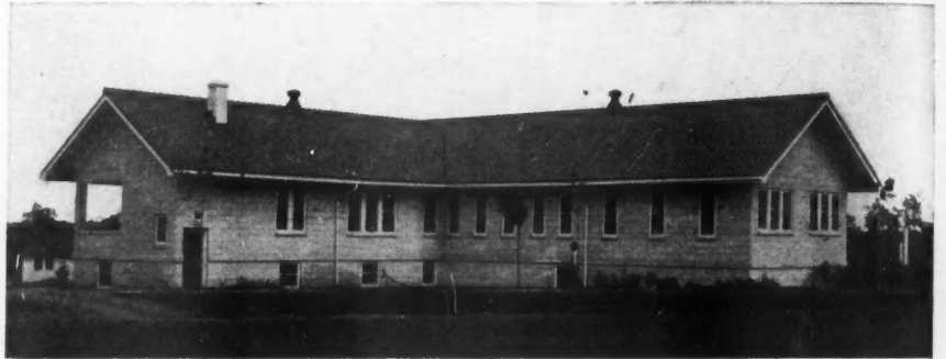
View Showing Right and Rear Wings of the Farm Boarding House at Mooseheart Farm.
