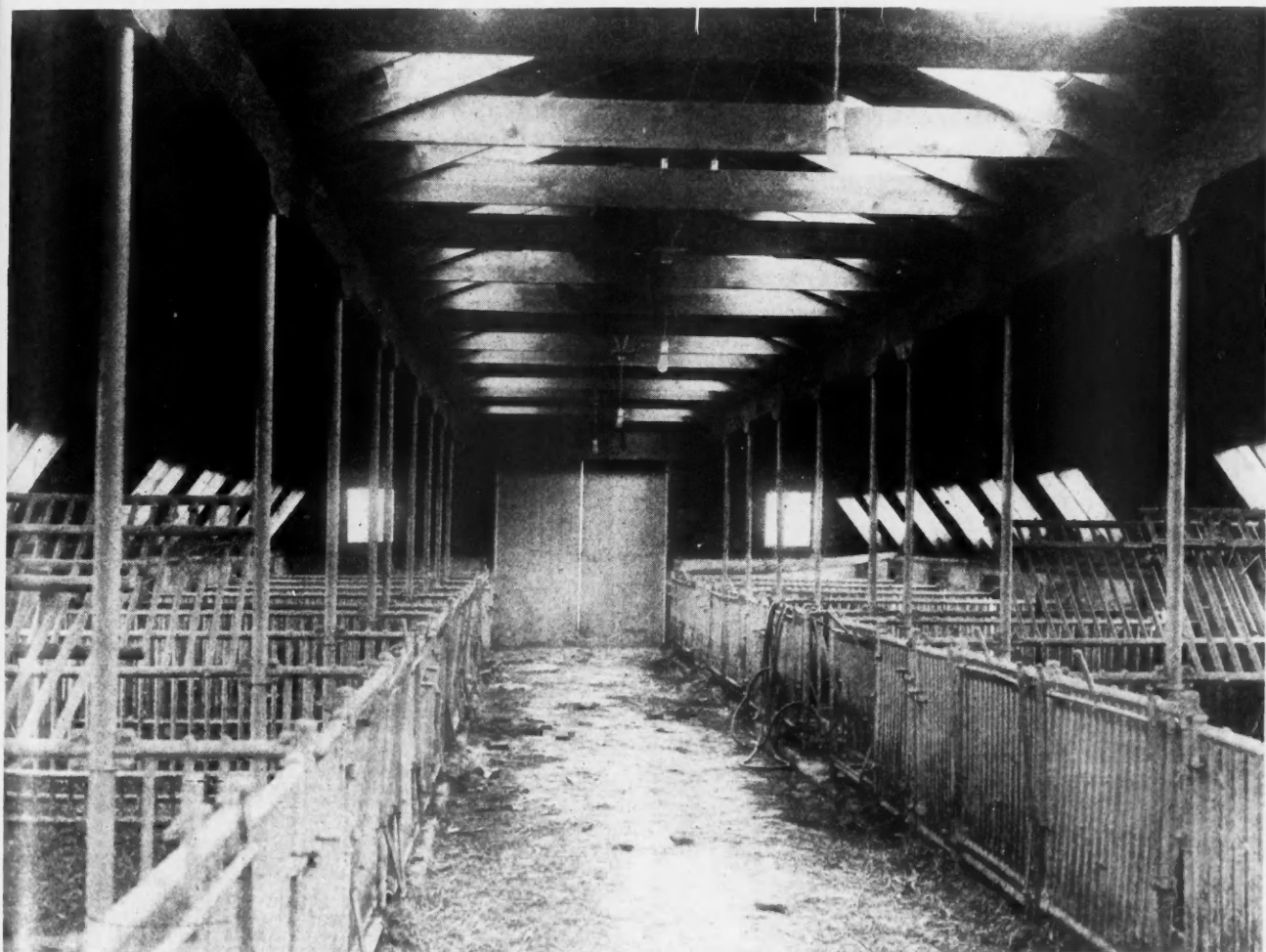
M ODERN "HOG PARLOR" ON JUST-A-MERE STOCK FARM. Owned by M. T. Anderson, breeder of Big Type Duroc Jersey swine at La Porte City, Iowa. The hog house is 28 by 80 feet, hollow tile construction with gambrel roof and special roof windows. The lower picture of the interior shows the wonderful lighting effect produced by the windows at 3:30 P. M. when this picture was taken. There are 48 windows in all, and 20 modern steel pens 7\frac{1}{2} by 9 feet. The main alley is 8\frac{1}{2} feet wide while the smaller alleys leading to the feed yards are 3 feet wide.
