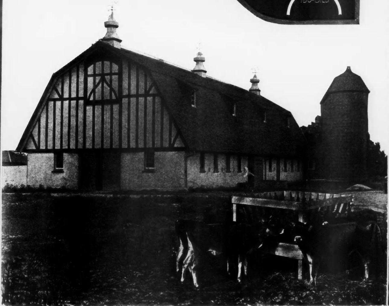
EXCELLENT TYPE OF GAMBREL ROOF BARN OF ENGLISH HALF TIMBER DESIGN. The walls are hollow tile, stuccoed on the exterior with timber effect above the first floor. Immediately adjacent are two large glazed hollow tile silos 16 feet in diameter connected with the feed mixing room. From this room, carrier track leads to all of the stalls which are arranged facing in on a large feed alley. There are 39 stalls of modern design with steel stanchions, drinking cups, and sanitary mangers. Carrier tracks running along the litter alleys take care of the litter carriers to the manure pit. Fresh air inlets and foul air vents have been installed to provide proper ventilation as well as roof ventilators. The large hay mow is well lighted by roof windows on each side. Size, 36 by 96 feet.
