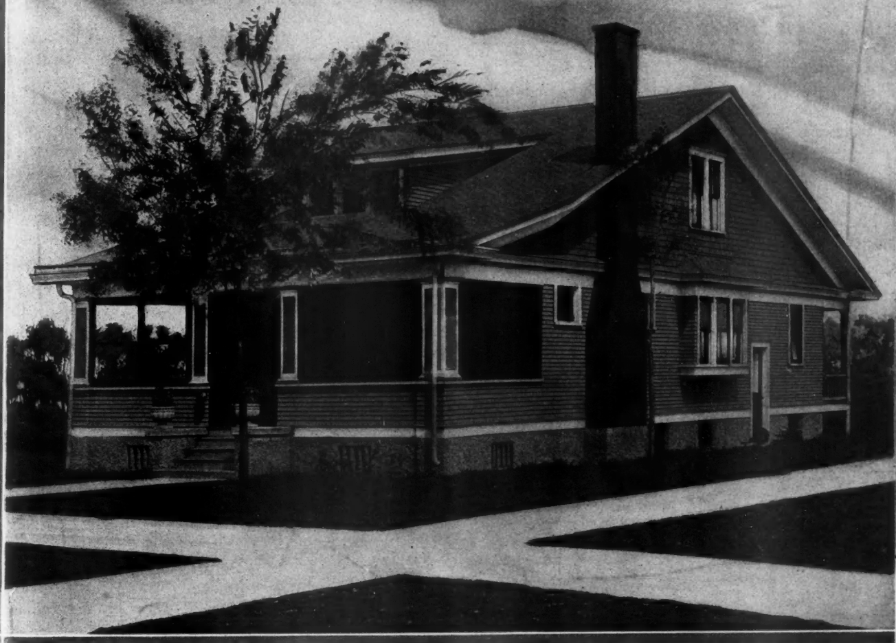
COZY STORY-AND-A-HALF HOUSE OF ATTRACTIVE DESIGN. This charming little frame structure with its broad front porch and concrete foundation stuccoed above the building line is bound to appeal to many people with family. The low gable roof gives the house an appearance of rambling comfort altho the building is not large, being 30 by 40 feet. The porch is screened in and covered by an extension of the main roof. On the first floor are four rooms: Living room, 16 by 13 feet, with open fireplace and wall bookcases; dining room with bay window; kitchen, 12 by 14 feet; one bedroom, and a washroom which can be used very conveniently on laundry day. This house would also suit very advantageously the needs of a farm home. Upstairs there are two bedrooms, bath, and a storage room.
