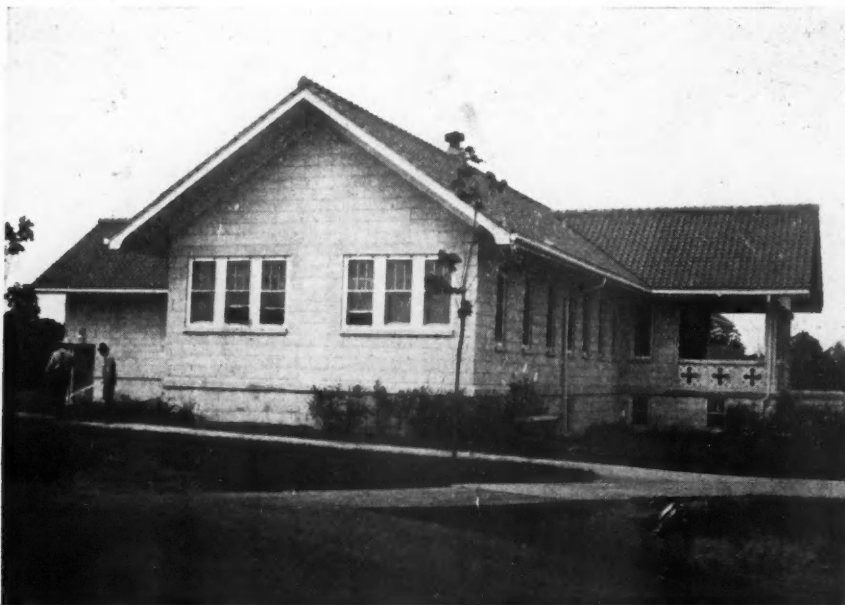
Side Elevation of the "Airship Type" Boarding House, Showing the Left Wing of the Building. The Abundance of Light and Air in the Sleeping Rooms, as Provided by the Many Windows, Is a Dominating Feature of the Plan.
