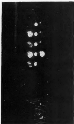
Fig. 1. Typical Lamp Annunciator Signal Such as Is Found in Any Hotel or Private Office Building. The Lights Are Red and White.
