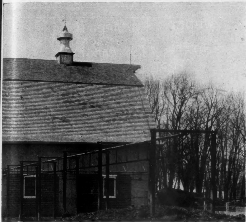
From the Litter Alley to the Manure Pile Via Rapid Transit. Carrier Systems Like the One Shown Here Are Being Installed in Modern Dairy Barns to Relieve the Boys and Hired Help of Much of the Burdensome Work Which Has Made Farm Work Unpopular.
