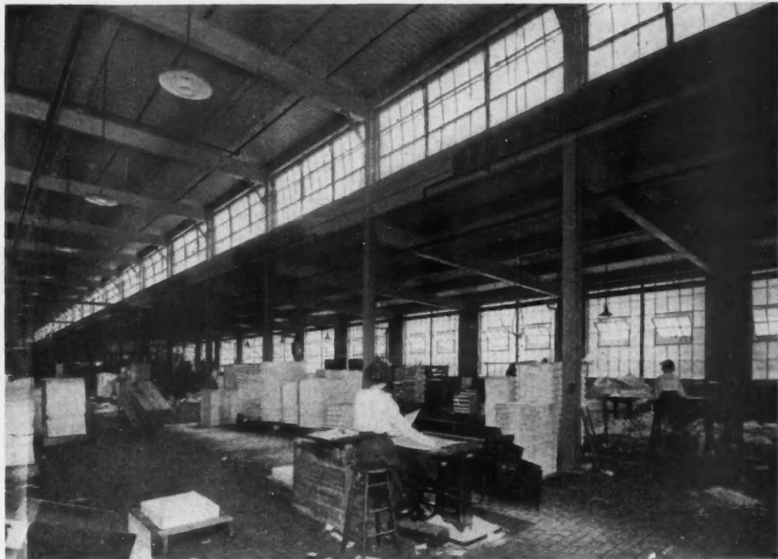
Interior of Bankers Supply Company's New Factory, Showing How Lighting Facilities Have Been Improved by Use of Steel Sash with Ventilators. The Floor Is Paved with Special Wood Blocks.
