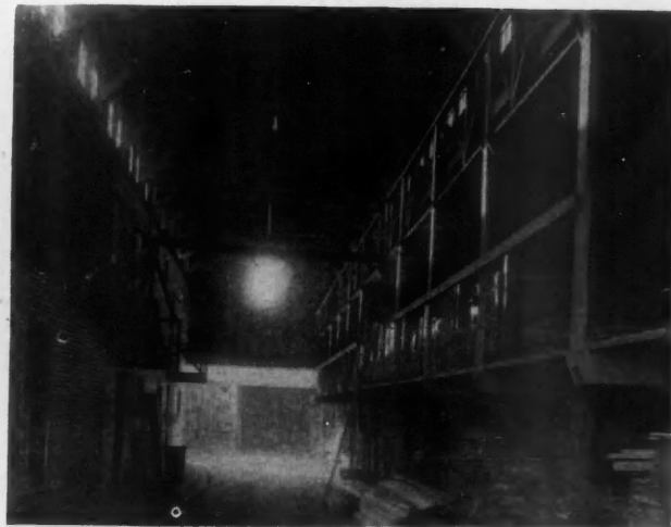
Shed No. 3. Note the Arrangement of Bins for Storage of Lumber. All Drives Are Concrete, Inside and Outside the Sheds, to Prevent Delay in Deliveries Frequently Caused by Muddy Driveways. Bad Weather Means Little in the Work of This Concern. Trucks Drive In and Out All Year Without Layoffs.
