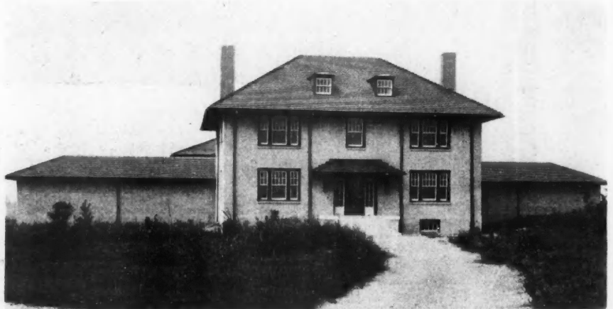
Front View of Administration Building. One of the Five New Buildings Which Have Been Erected in League Island Park. It Is Gray Brick with Roof of Red Tile. The Low Wings Are Sheds for Tools and Wagons.
