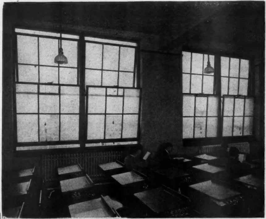
Plenty of Daylight Is Essential for Two Reasons—Light and Ventilation. Special Windows and Hardware of the Type Shown Here Have Been Instrumental in Keeping the Eyes of the Children Strong and Their Bodies Healthy.
