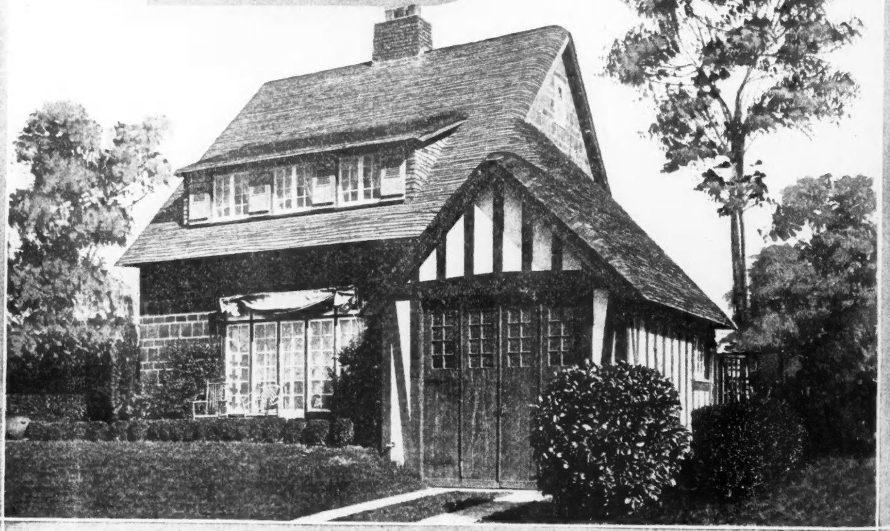
CHARMING HOME OF UNIQUE DESIGN. There are several features about this pleasing little home that help to make it distinctive and different. There is the hollow tile exterior, thatched roof, and built-in garage with its tall doors and half timber effect walls of stucco. The casement windows and French doors are also very attractive—in this home they are metal, similar to those shown in detail on the opposite page. The entrance to the house is on the left side. It opens into a reception room which is located between the living and dining rooms. The living room is large, well-lighted, with an open fireplace in the inside wall. A small den adjoins it. The kitchen is very completely equipped. Upstairs are four comfortable, cheerful bedrooms with ample closet room. The garage is 12 feet 6 inches by 20 feet. The house is 36 by 32 feet.
