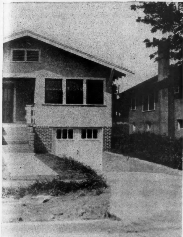
Little Excavation Was Required to Make This Drive. The Owner Has a Garage in the Basement, an Excellent Shelter for His Car in the Cold Months. These Built-in Garages Add to Driving Comfort.
