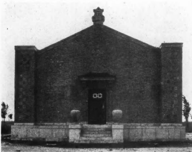
Rear View of Bandstand. Note Entrance. This Stand Is of the Semi-Open Type and 35 Feet in Diameter. The Rear Wall Is Brick with Stone Trimmings. A Stone Lyre Surmounts the Structure.
