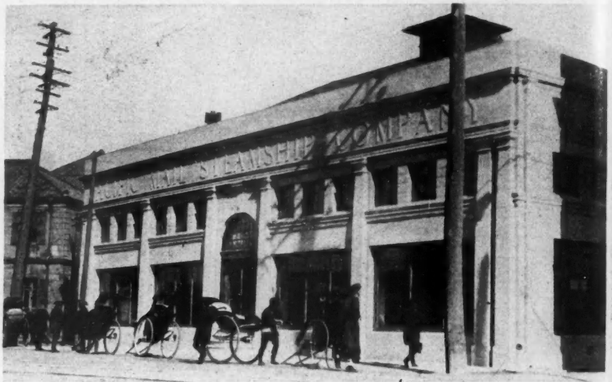
Reinforced Concrete Office Building of the Pacific Mail Steamship Co. at Shanghai, China: Were It Not for the Rickshaws, This Picture Might Have Been Taken in an American or European City.
