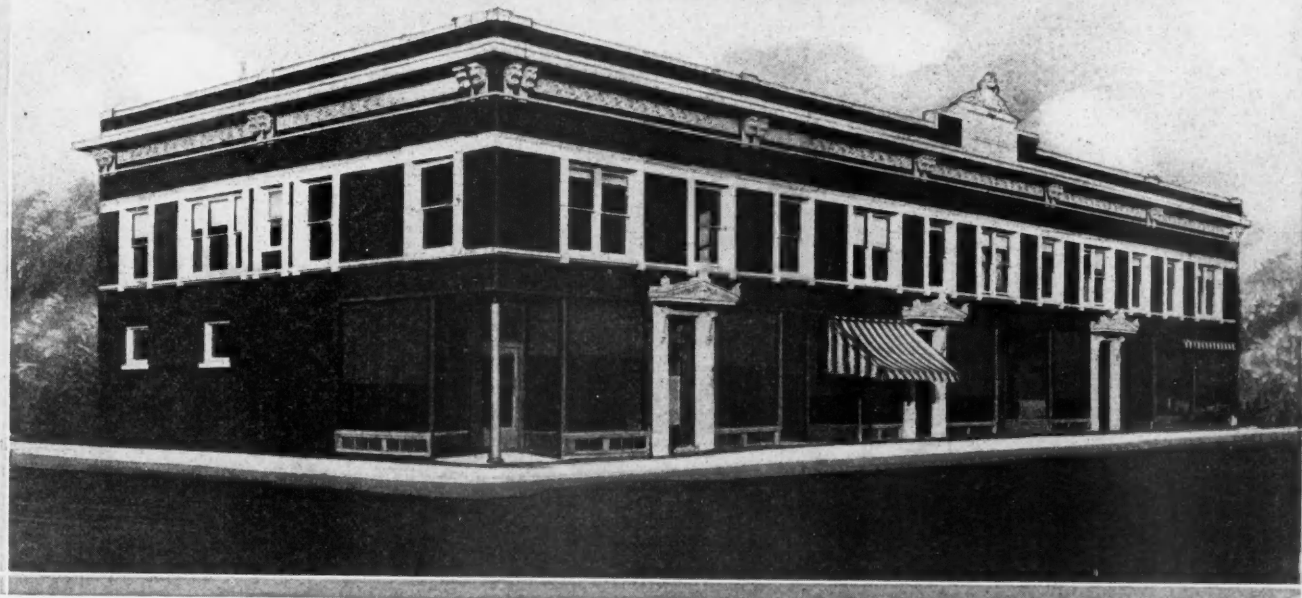
E FFICIENT CORNER LOT STORE AND APARTMENT BUILDING. This exemplifies an excellent handling of the corner lot building problem to gain maximum results. On a site 42 by 120 feet, the contractor has erected a building containing seven stores on the first floor and six modern apartments upstairs. The income feature of such a layout is apparent. The building is of brick with attractive terra cotta trim, all store fronts of the latest types. The corner store is the largest, 16 by 53 feet, the others being 41 feet deep and ranging from 11 to 17 feet in width. The apartments contain three, four, and five rooms. Plenty of window space is provided along the front and side walls and courts in the rear of the building. The floors of the stores are rubber tile, details of which are shown on the opposite page.
