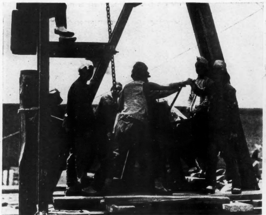
Primitive Building Methods Are Still in Use in Many Parts of the Orient. This Picture Shows Natives Operating a Hand Power Pile Driver.
