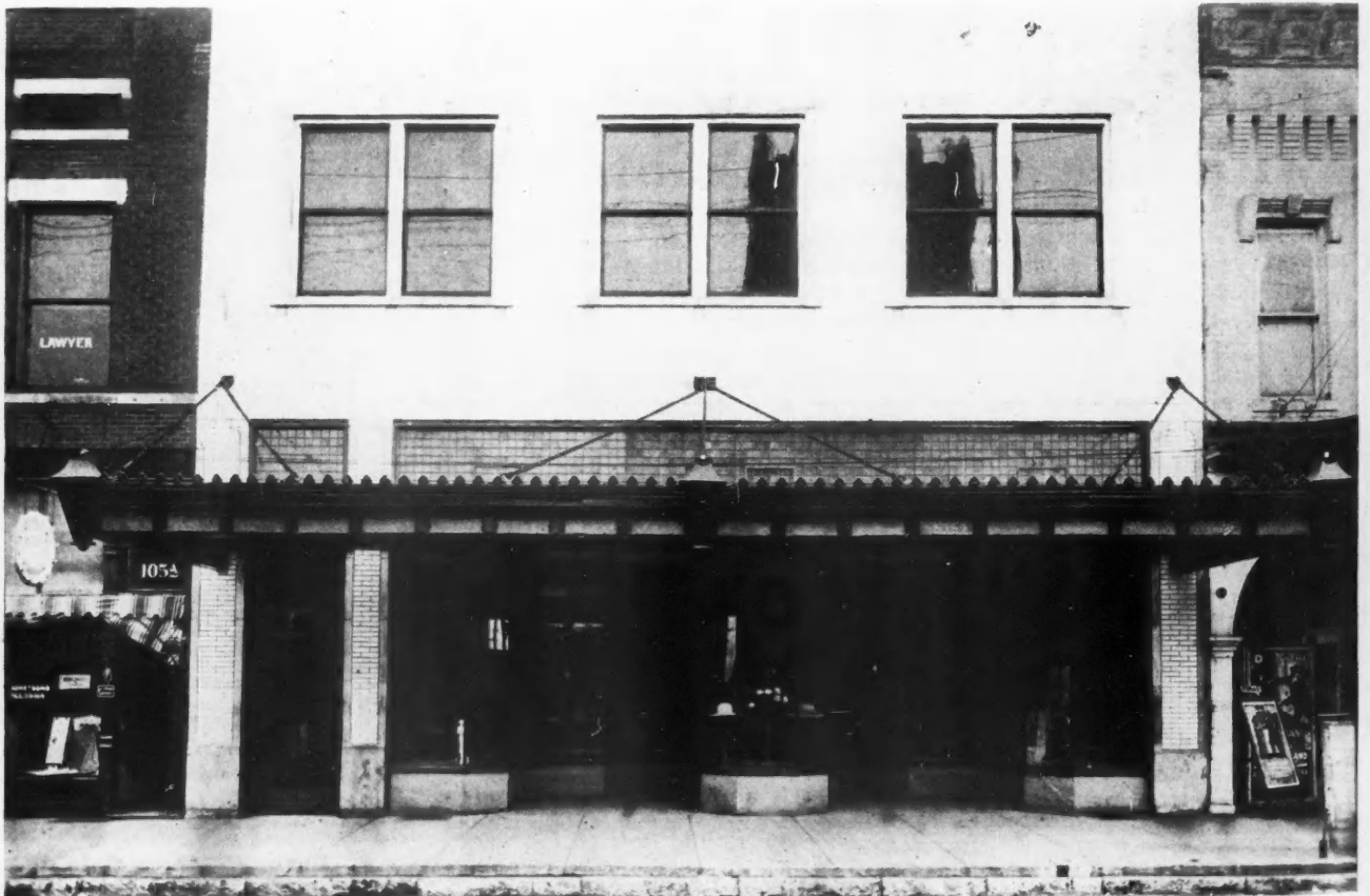
The Type of Canopied Store Front That Is Installed in Many Modern Retail Establishments. The Broad Entrance Narrows to the Door, Giving a Large Amount of Window Display Space.
