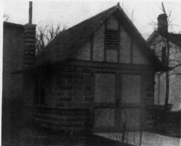
Pleasing Effects Are Obtained by the Use of Concrete Blocks with a Variety of Faces. Plain Face and Rock Face, with Stucco and a Belt Course at the Sill Line, Make This Garage Attractive in Exterior Appearance.
