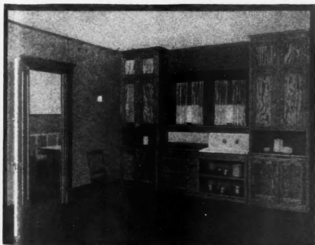
A Built-In Kitchen Cabinet Makes the Kitchen Work Easy. Note How Windows Have Been Placed Over the Sink, with the Cases for Dishes Within Arm's Reach. A Glimpse of the Breakfast Nook Also Is Given.
