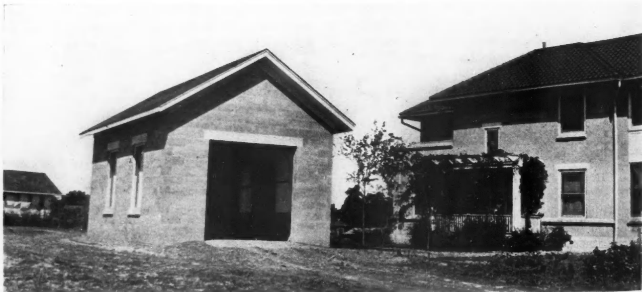
A Single Car Garage of Smooth, Granite Face Concrete Blocks. The Garage Is Unfinished, But Will Have a Roof of Concrete Tile. The Walls and Roof Correspondent to Those in the Adjoining Residence.
