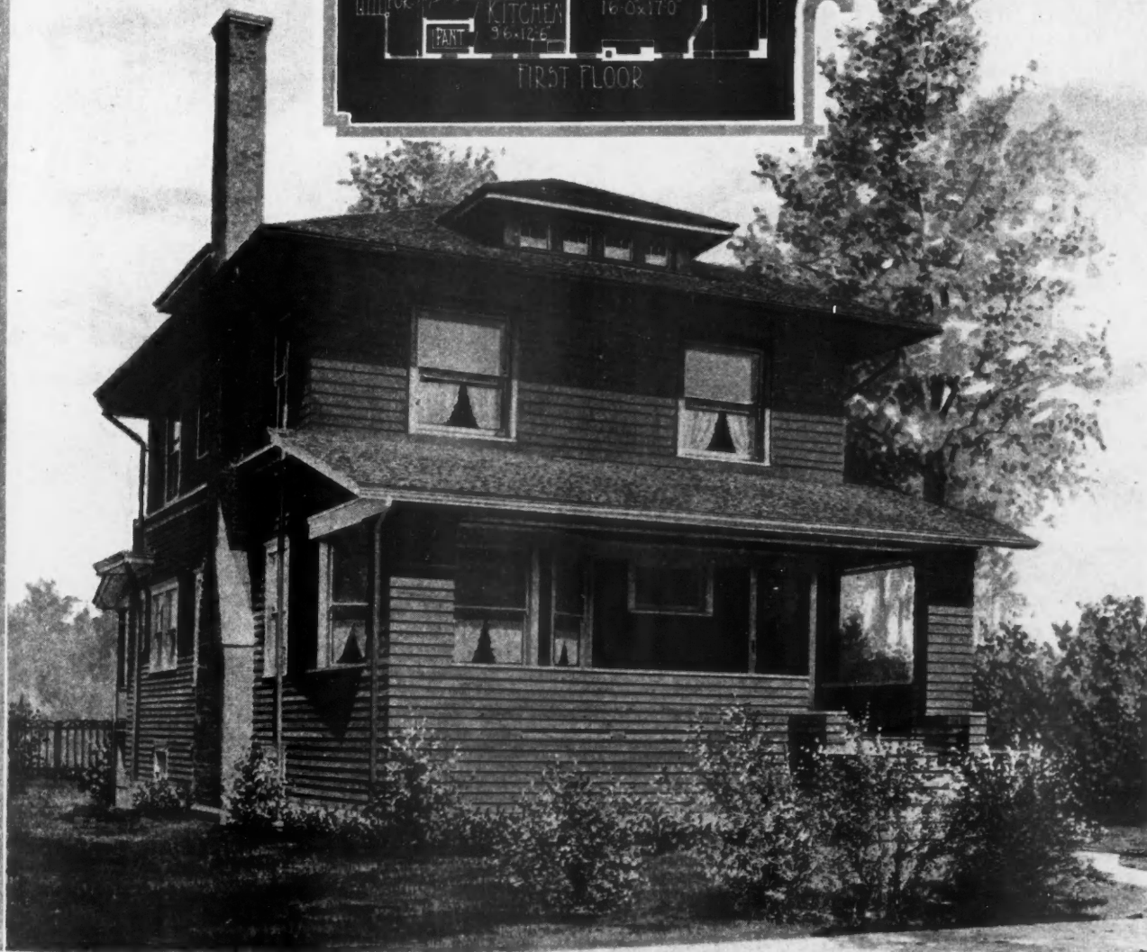
S EVEN-ROOM, HIP-ROOF FRAME HOUSE. This is the type of house that always is in demand. It is only 26 x 30 feet in dimensions, but it contains seven good rooms, living and dining rooms and kitchen on the first floor, and three bedrooms, den and bathroom on the second. The 10-foot porch, extending across the front of the house; the hip roof with dormer in the front and the lapped siding give the house a good exterior appearance. The floor plan shows how excellently and compactly the rooms have been arranged. Over the pantry extension at the rear of the house there is a balcony, 6 by 16 feet, which can be enclosed for a sleeping porch.
