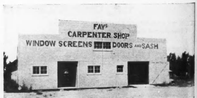
Arthur H. Fay's Carpenter Shop, Kimberly, Idaho.
