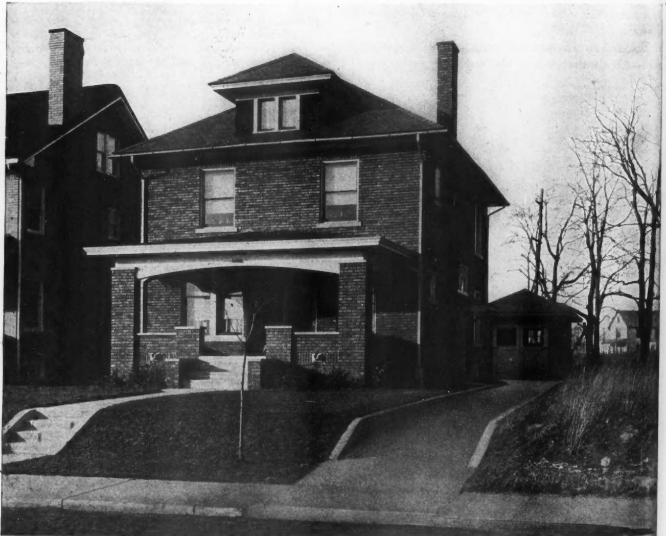
SEVEN-ROOM BRICK HOUSE. Here is a design for a home of rough face brick that will find many admirers among prospective home builders. Its dimensions are 30 by 40 feet, and it has a most attractive porch. The garage, shown at the rear, is of the same materials and same architectural design.
