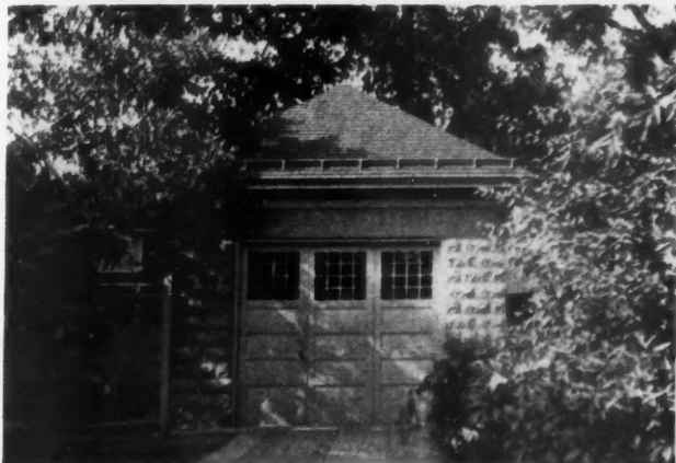
Rock Face Concrete Block Garage. Attractive Doors Add Greatly to the Appearance of This Garage.
