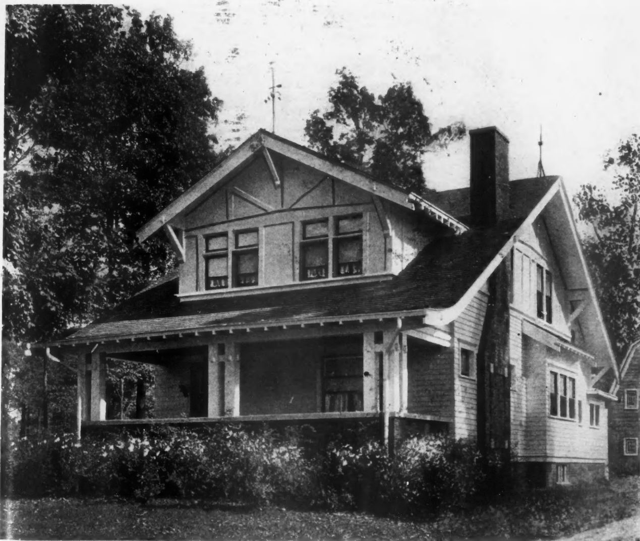
AN IDEAL HOME FOR THE AVERAGE FAMILY. This seven-room house of the bungalow type of architecture contains seven rooms with all the modern features that are good in home construction. The house is of frame construction, and is 26 by 45 feet, suitable for a narrow lot. The broad porch and large living room make this a comfortable home in both summer and winter.
