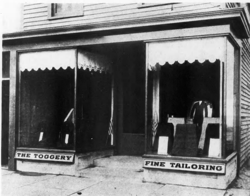
A Frame Business Building That Has Been Modernized by the Installation of a Standard Store Front. The Front Has Greatly Increased the Value of This Building for Business Purposes.
