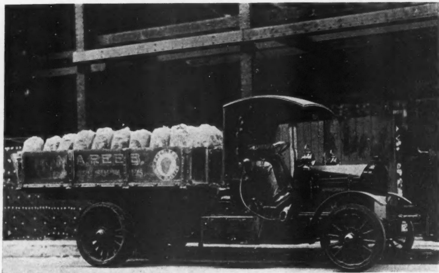
Heavy Materials Require a Staunch Piece of Delivery Equipment. Here Is the "Pierce-Arrow" Truck Used by M. A. Reeb to Handle Heavy Loads of Cement.
