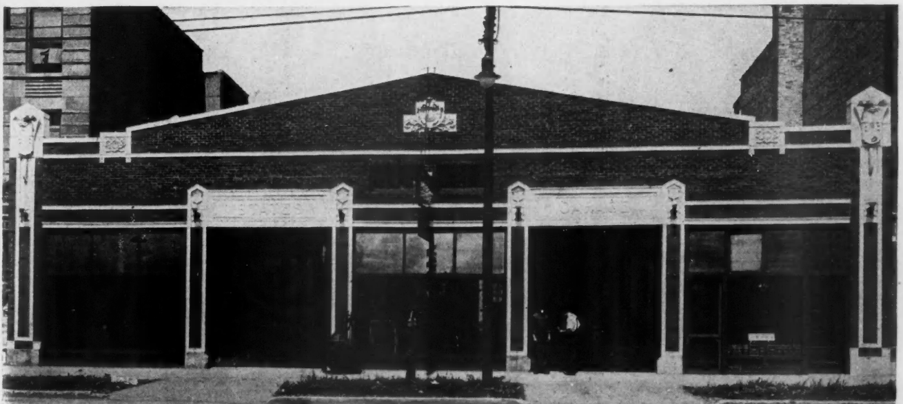
Perspective of a Public Garage, of Concrete, Face Brick and Terra Cotta. The Building Is 66 by 120 Feet in Dimensions and Provides Storage Space for a Number of Cars. An Office, Display Room for Accessories and a Stock Room Are Located at the Front of the Building.
