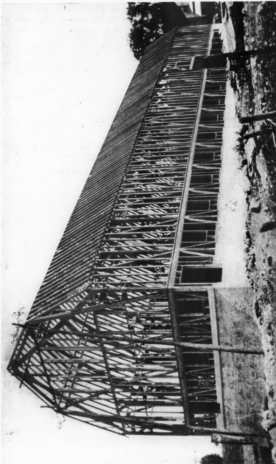
The Combination Dairy and Horse Barn, Erected at West Cornwall, Vt., by D. W. Ames, of Brattleboro, Vt., a Member of the American Builder Family. This Structure is 42 by 165 Feet, of Plank Frame Construction, Set on a Concrete Foundation. This Photograph Was Taken During the Course of Construction and Is an Excellent Example of This Method of Barn Framing. There Are Stalls for 64 Cows and Pens for Their Calves, a Bull Pen, Two Sheep Pens, 20 by 40 Feet, a Horse Stable and Vehicle Storage Space on the Mow Floor, and a Mow That Will Hold 225 Tons of Hay. About 115,000 Feet of Lumber Were Used in the Structure. A View of the Barn After It Was Finished and Floor Plans of the Building Furnished by Mr. Ames Are Shown on the Following Page.
