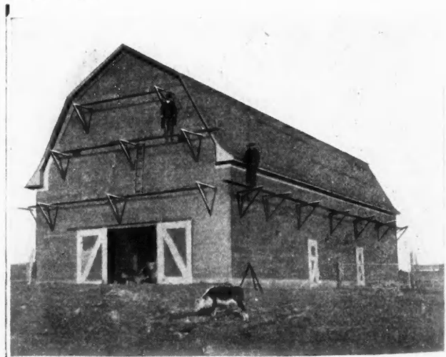
Reliable Brackets Installed on Barn.
