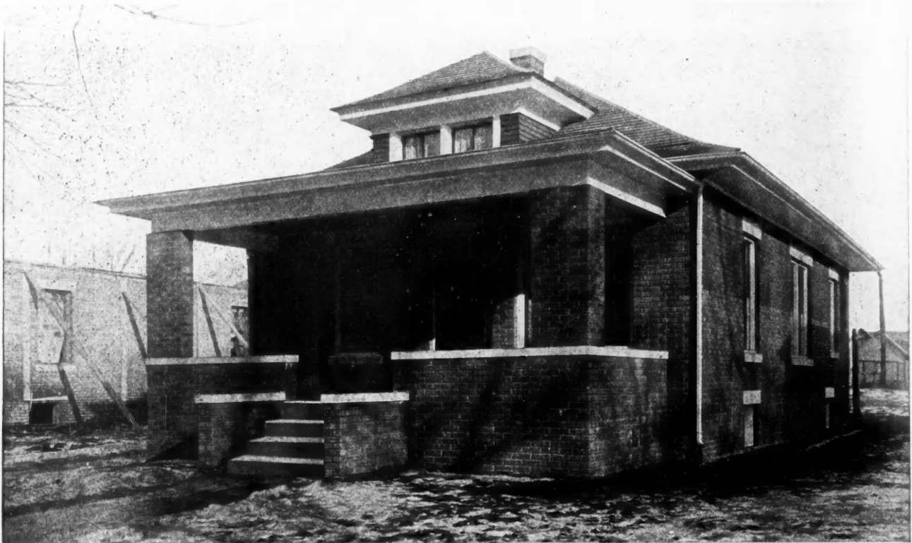
Photo A. A Six-Room Brick Veneer and Tile Bungalow, Which Sells Readily for $3,600.00. Contractor Schindelbek Says He Can Handle Two Such Houses with No More Attention to Detail Than One House Formerly Required.
