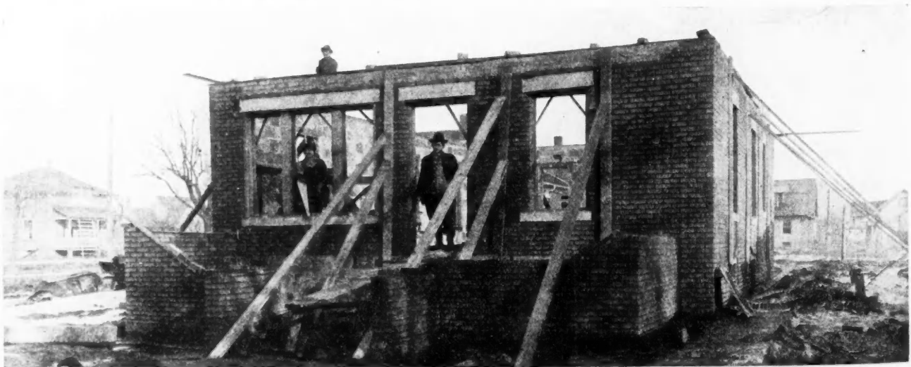
Photo B. Contractor Schindelbek in the Doorway of One of His Brick and Tile Cottages at Aurora. The Braces Are to Keep the Walls in Alignment, as This Job Was Done in Zero Weather.
