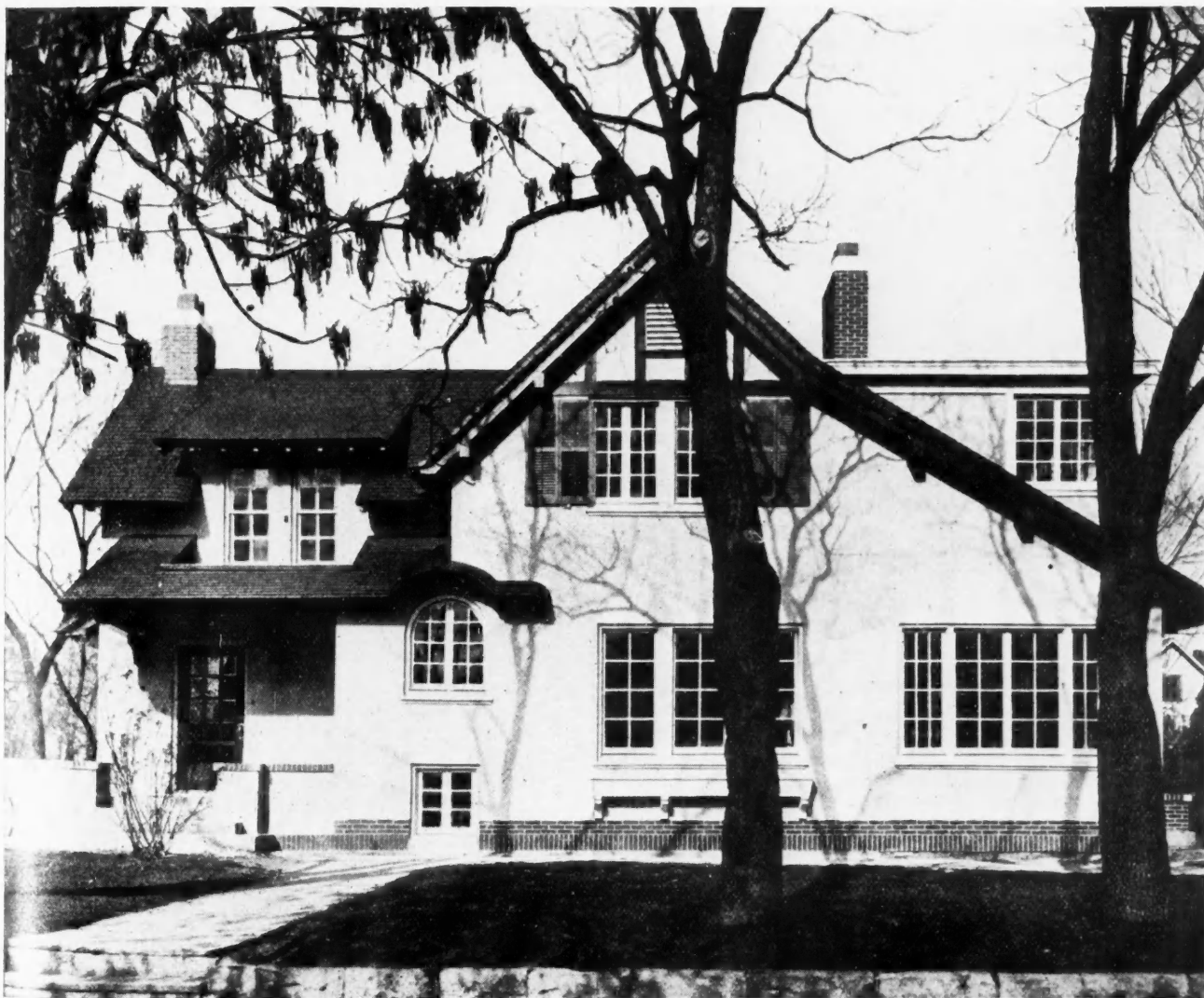
Plate D. Mr. Whiteside's House After Remodeling. Did You Ever See a More Attractive, Up-to-Date Looking Job. Overcoated with Cement Plaster on Metal Lath. Root & Siemens, of Kansas City, Architects.
