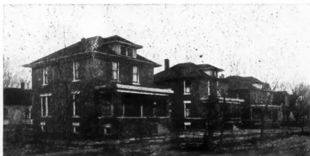
Type of Houses First Erected by Contractor Schindelbek and Selling at About $4,000.00. The Bungalow Type Adopted Later Sells More Readily and at a Better Margin of Profit.
