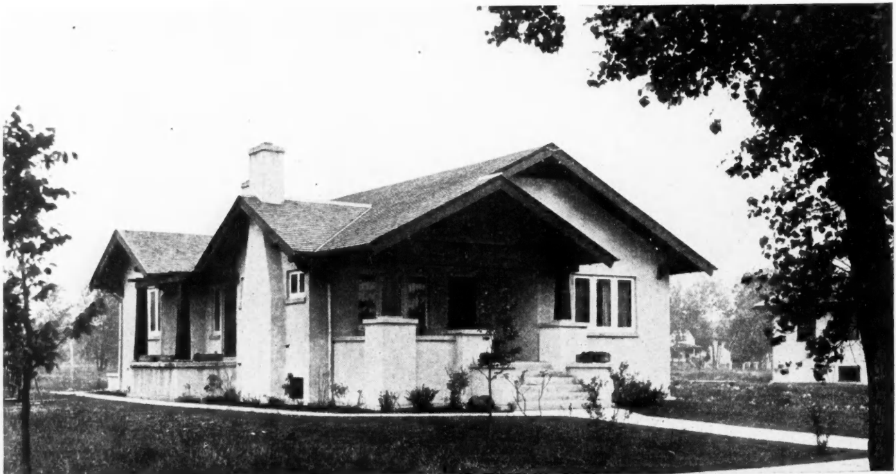
A Plastered Tile Bungalow of Strictly Modern Design, Containing 5 Rooms and Bath. We Will be Glad to Give Any Further Information Desired Concerning this Design or Can Furnish Blueprinted Working Plans and Typewritten Specifications for Only $8.00 Per Set. In Writing Please Mention Design No. 6886.
