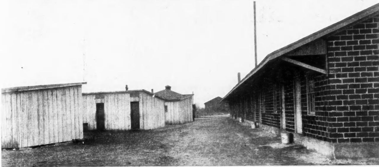
Fig. 1. The New Negro Shacks of Tile on the Right which Replace those on the Left at the Bethlehem Steel Company Plant at Sparrow's Point, Md.
