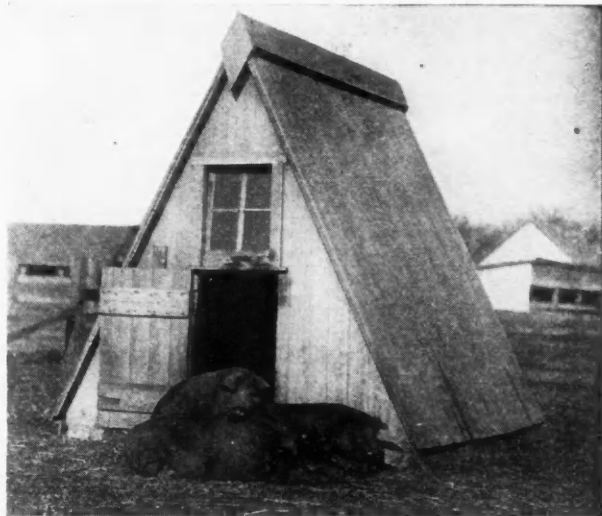
"A" Shaped Hog House or Portable Cot of the Sort that Every Farmer Likes and Usually Wants Ten or a Dozen of.
