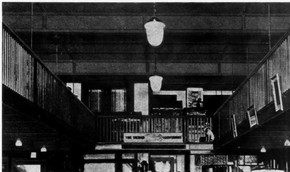
This is a photograph showing the Beaver Board ceiling which was flooded. In the Store of Mel Moorhead, McDonald, Pa.
