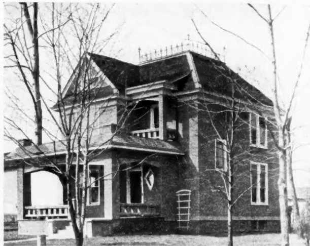
Plate F. Peru Residence Modernized by Cement Plaster Overcoating.
