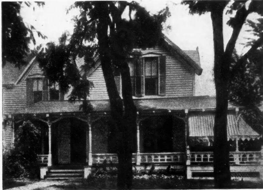
Plate C. Old-Time Residence of Mr. A. Whiteside, Hutchinson, Kansas. Compare this Photograph Carefully with the One Below, Showing the Same House Remodeled.
