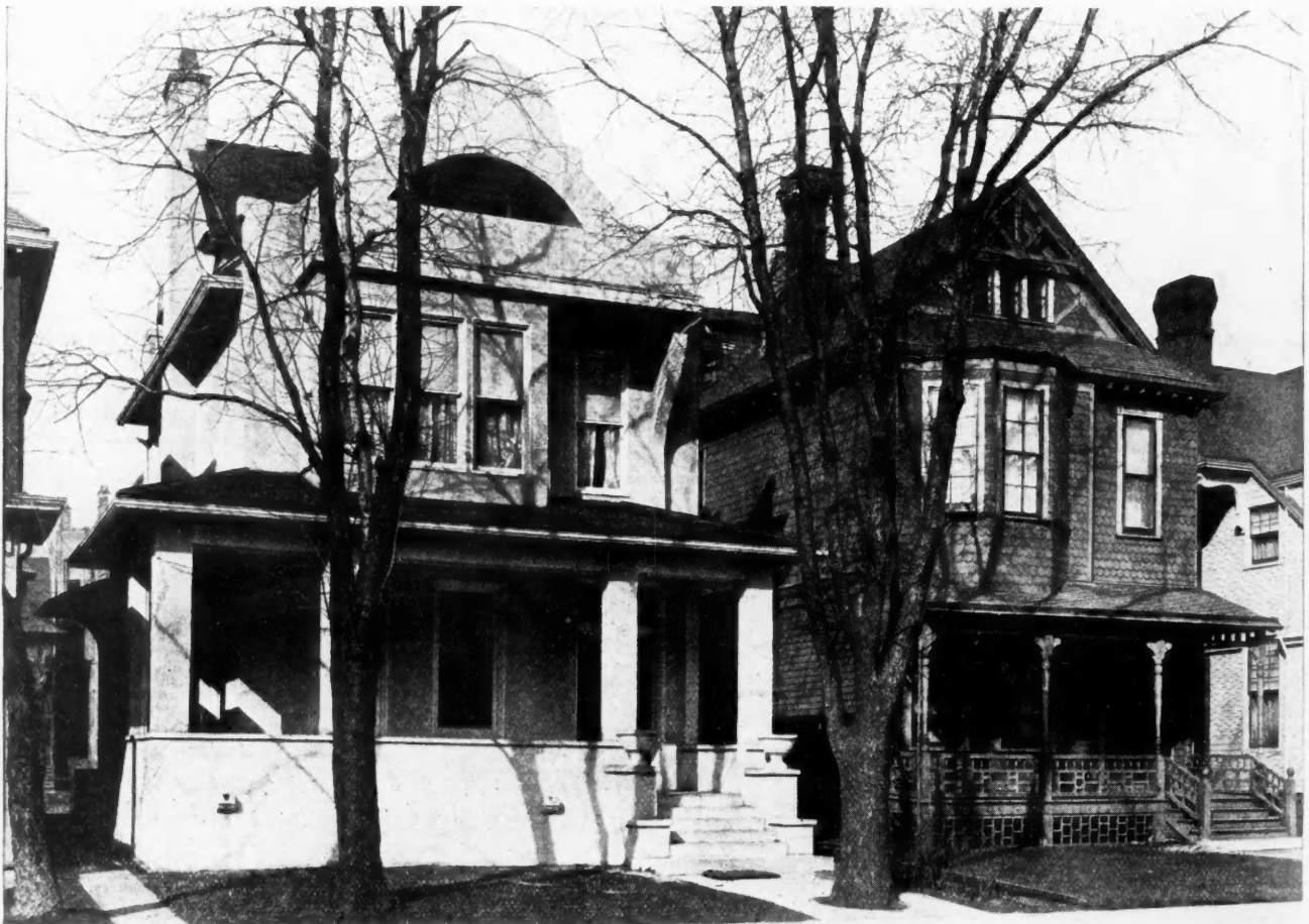
Plate A. Originally Twin Houses, Frame Construction with Shingled Siding. This House to the Left Has Been Modernized by Overcoating with Cement Plaster on Metal Lath.
