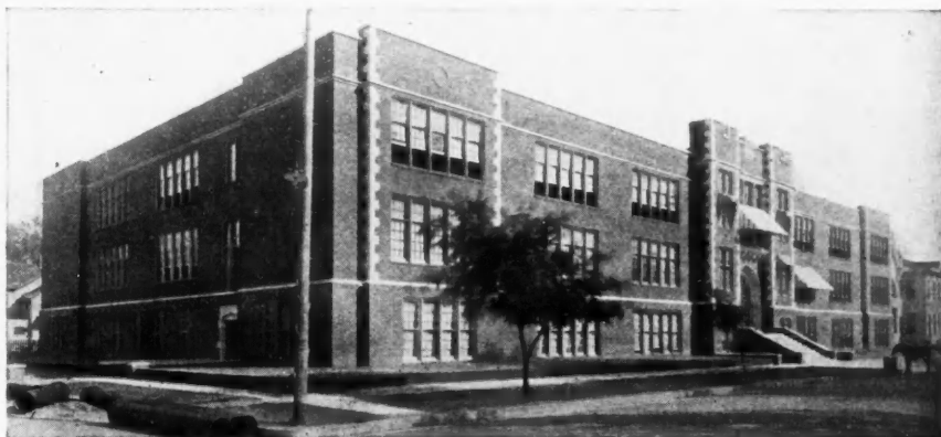
Plate B. Wichita, Kansas, High School Plastered Thruout on Metal Lath. Reason, Fire Protection.
