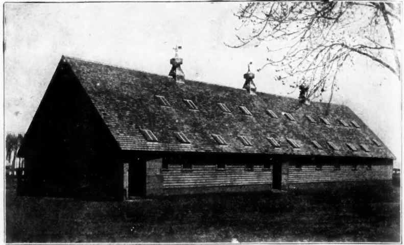
Hog House of W. I. Isgreg, Kekamah, Neb. It's for Prize Winners and Has Chief Sunshine Roof Windows.
