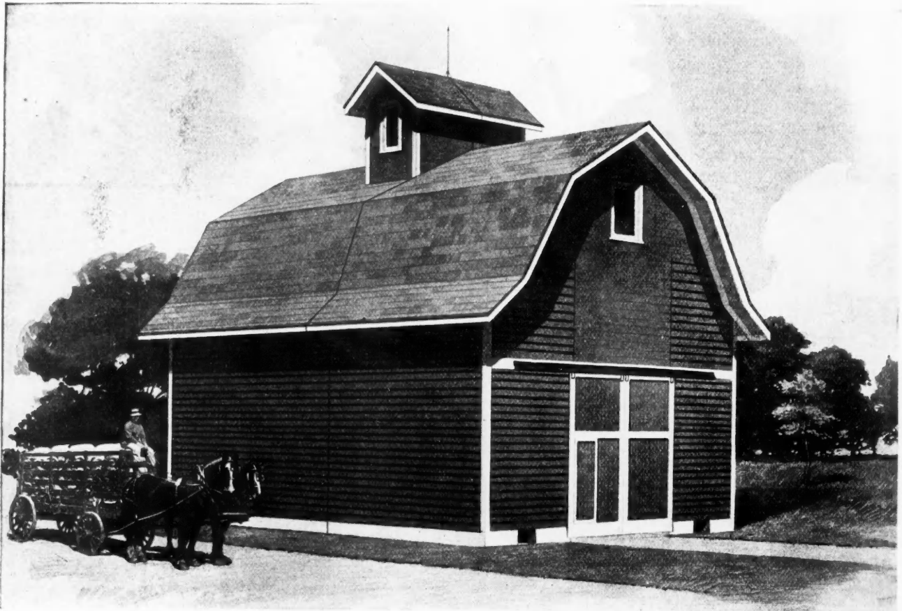
The Type of Two-Story Corn Crib and Granary Which Is Being So Successfully Used on the Average Farm. Equipment Includes Cup Elevator for Putting in Grain and Drag Chain for Taking It Out. Design No. A391.
