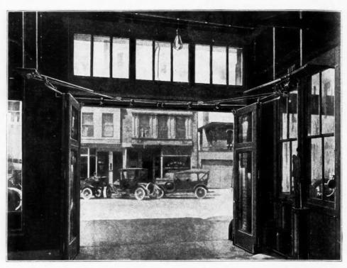
View Looking Out Thru Public Garage Doors Equipped with the R-W Stewart Electric Door Opener,
