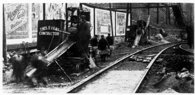
Two Ideal Cincinnatus Tractor Paving Mixers at work on Colerain Ave., Cincinnati, Ohio, since May, 1915. These mixers were adopted because of their compact construction and because they prevented the tying up of the trolley service on that busy thorough-
