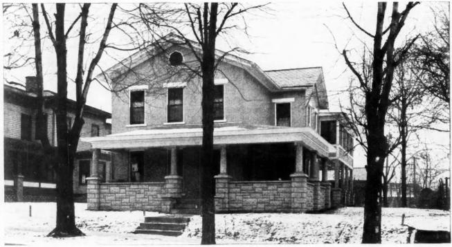
Formerly Unattractive House Improved in Value and Appearance by Concrete Block Porch Built Around Two Sides of Structure. The Total Cost of Remodeling Was Only \$570.00.
