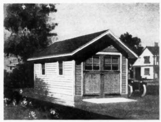
Simple Frame Garage Listed as Design No. G160. The Floor and Foundation Are of Concrete.
