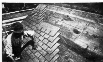
Laying Rex Strip Shingles in Milwaukee, Wis. Two Men Laid 14 Squares of "Strips" on a Straight Roof in Eight Hours.
