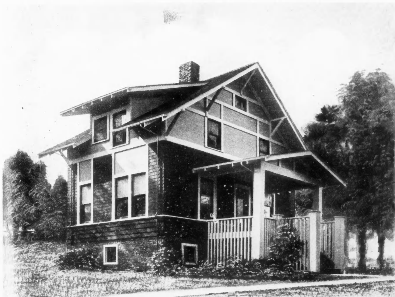
Modern two-story, six-room house. Size 32 by 22 feet. We can furnish complete set of blueprinted working plans and typewritten specifications for only $7.00 per set. Blueprints consist of basement plan; roof plan; first and second floor plans; front, rear, two side elevations; wall sections; and all necessary interior details. Specifications consist of twenty-two pages of typewritten matter. When ordering, ask for Design No. 6763.
