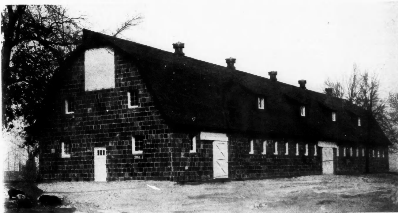
Structural Tile Barn, Size 36 by 162 feet, for Watertown State Hospital, Watertown, Ill. An Example of a Most Efficient and Economical Way of Building a Modern Barn. Designed by Illinois State Architect, James B. Dibelka.
