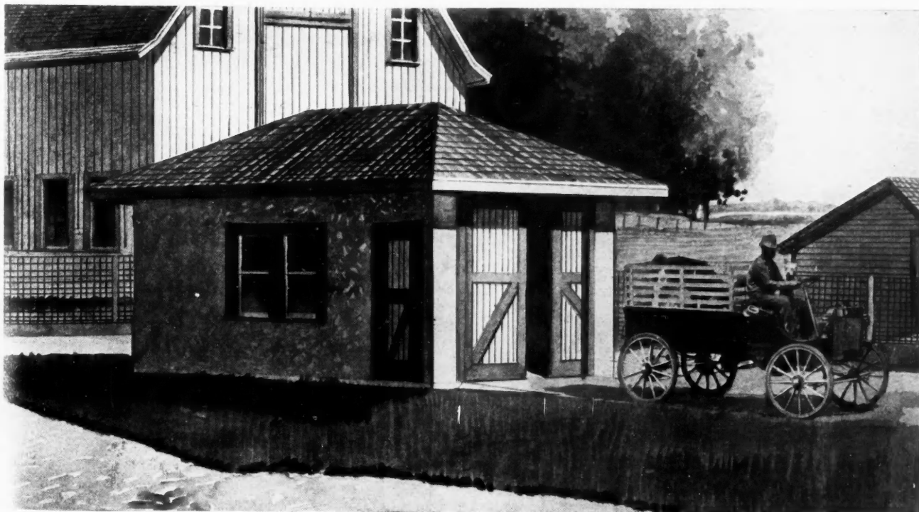
Photographic Architectural View of Garage and Power House, a Fire-Resisting Building of Metal Frame and Roof with Concrete Siding; Size 14 by 24 Feet. Big Enough for Work Bench and Gas Engine Outfit, in Addition to Garage Space. This is Design No. G 159.
