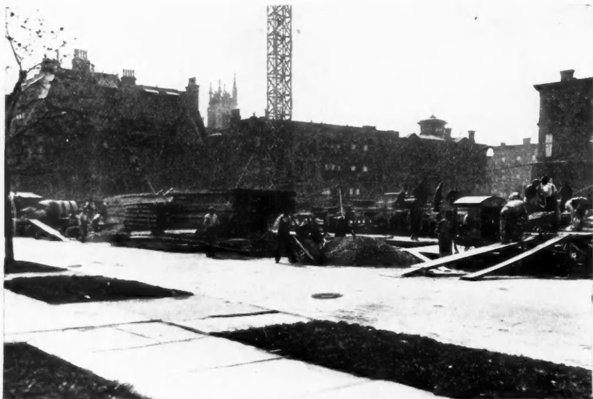
Standard Mixers in Use on Methodist Book Concern Building.
