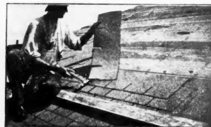
Laying Rex Strip Shingles in Milwaukee, Wis. Two Men Laid 14 Squares of "Strips" on a Straight Roof in Eight Hours.
