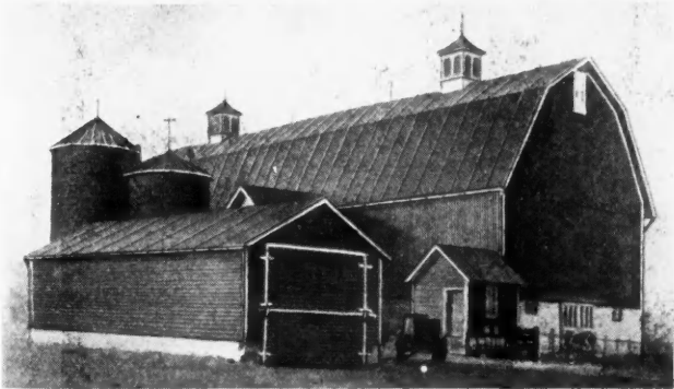
"You Need Have no Hesitation About Using Corrugated Iron for our Implement Shed," said the Builder. "Here is a Photo of an entire Group of Farm Buildings Constructed of It."
