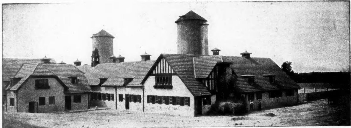
Notable Buildings on "Wabeek Farm" of James Couzens, Birmingham, Mich. Cement-Plastered Metal Lath Used for Silos, Fences, Partitions, Etc. Albert Kahn, Detroit, Mich., Architect; Ernest Wilby, Associate.
