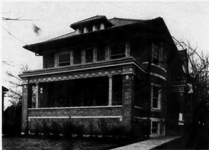
Beautiful and Expensive Brick Residence Trimmed with White Enameled Terra Cotta of Special Design.
