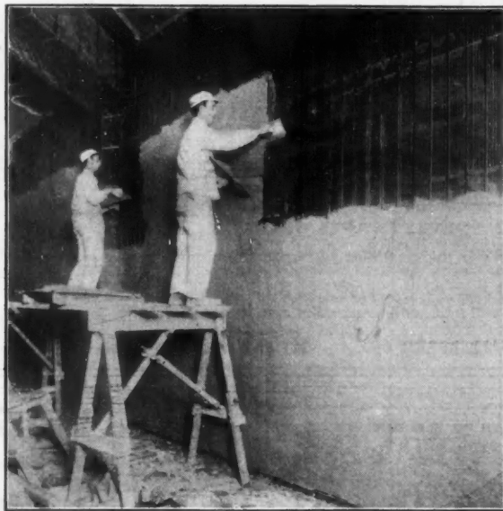
Plastering Hy-Rib Partition, 18 feet high
