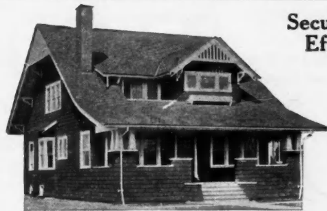
Home of J. J. Cleary, Charlotte Blvd., Rochester, N. Y. Architect, H. B. Nurse, Rochester, N. Y.
