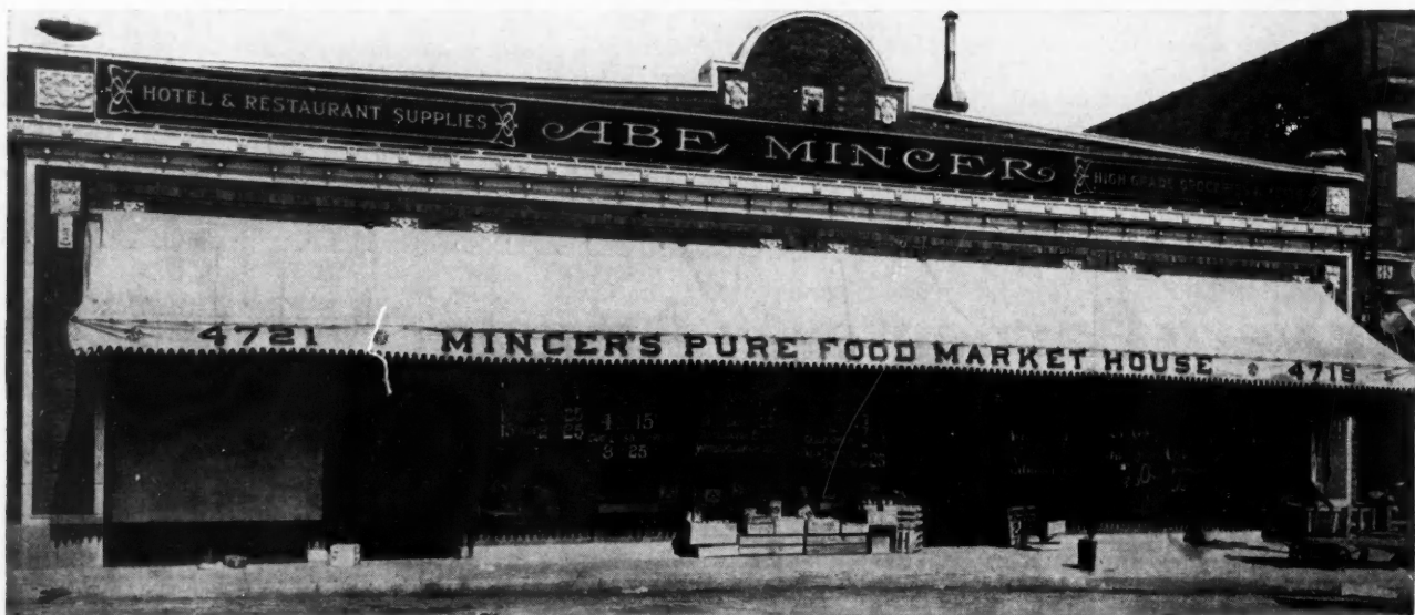
This Attractive Building Is Trimmed With Midland Stock Terra Cotta
