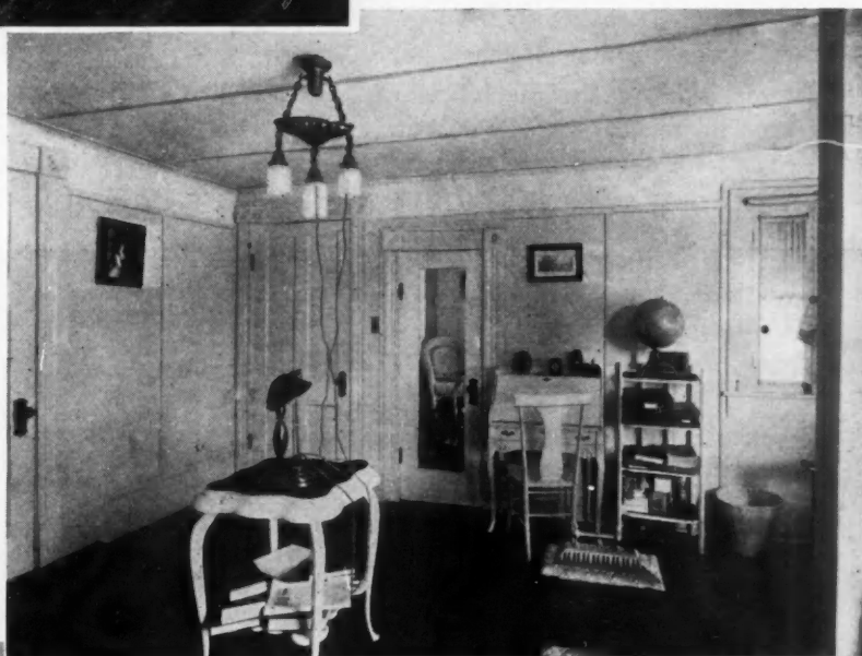
A Notable Example of "Beaver Board" Construction is the Residence of Mrs. Wolf, San Antonio, Tex. In Every Room Some Strikingly Beautiful and Different Effect Has Been Produced. This Bedroom is Finished in White Enamel with Panel Trim Very Inconspicuous.
