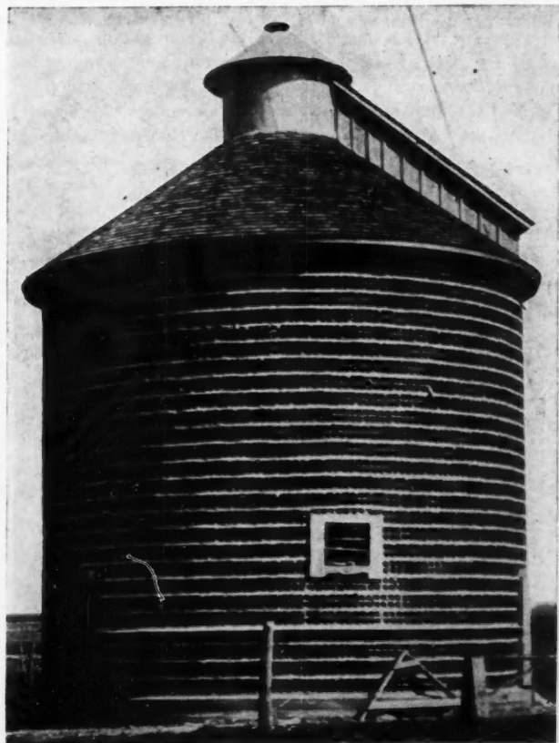
Near View of Tile Crib Showing Four-Hole construction of Each Tile. Holes Slant Upward to Exclude Driving Storms.
