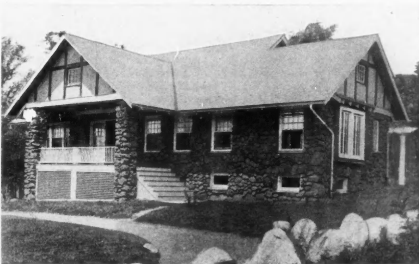
Fig. 1. Home of A. P. Richardson, Cragmere Park, N. J.—An extra attractive example of Cobblestone work.
