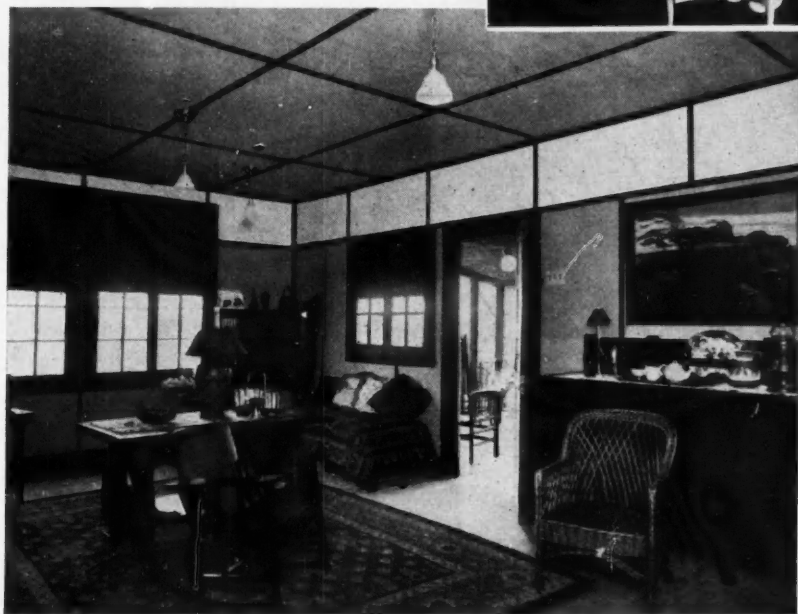
Living Room in Central New York Residence in Which No Lath and Plaster was Used, the Finish Throughout Being "Plastergon" Wall Board. Note Attractive Paneling Effect With Strong Contrast Between Dark Finished Battens and Light Spaces.
