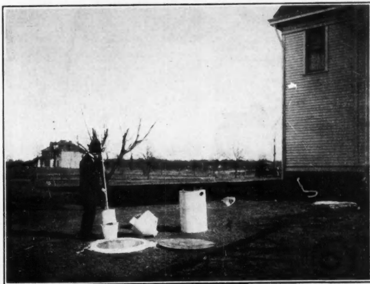
It is a Small Task at Long Intervals to Clean Out the Generator. Photo Shows Operation where "Jenne" Outside Pit Generator is Used.
