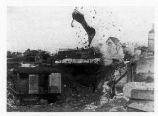
Blasting through 6 ft. of "Frost" for Rush Foundation Work
