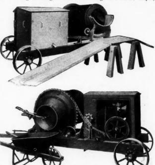
Northwestern Cone Batch Mixer, Intake Side (above) and Discharge Side (below)
