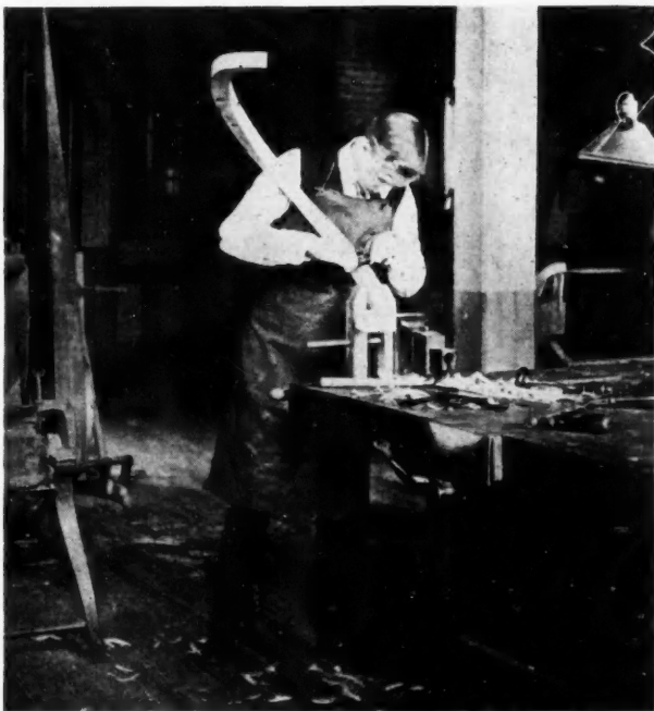
Working out Spiral Handrail for Colonial Stair
