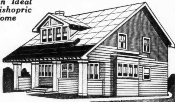
Ideal home showing Weather-boards over Bishopric Sheathing, lath side exposed, also Bishopric Roofing over Bishopric Sheathing. (smooth side of sheathing exposed)
