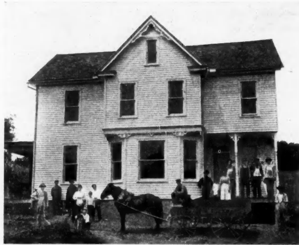
Contractor Barr, Clients and Men
