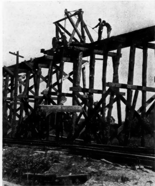
Portable Gasoline Engine Hoist, with Derrick Handling Timbers for Railway Trestle
