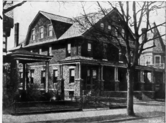
Residence of Mr. Patrick McCauley, Brooklyn, N. Y. Covered with J-M Asbestos Shingles A. J. McManus, Architect
