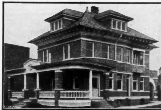
Asbestos "Century" Shingle Roof—Residence of Dr. Thomas H. Bowman, Harrisburg, Pa.; Harry B. Shoop, Harrisburg, Architect; James M. Bowman, Harrisburg, Contractor
