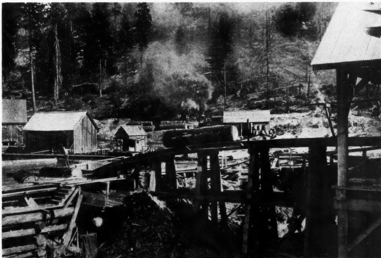
From Pond to Mill by Endless Conveyor—California Sugar Pine Region
