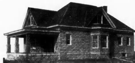
MODERN CONCRETE BLOCK BUNGALOW
