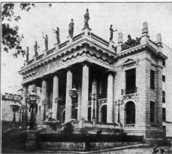
MEXICAN THEATRE JUAREZ, Guanajuato, Mexico. Rivas & Malo, Architects, Mexico City, Mexico.
