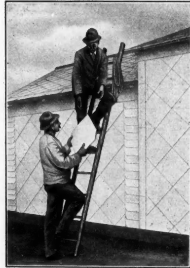
Asbestos "Century" Shingles as a Sheathing
