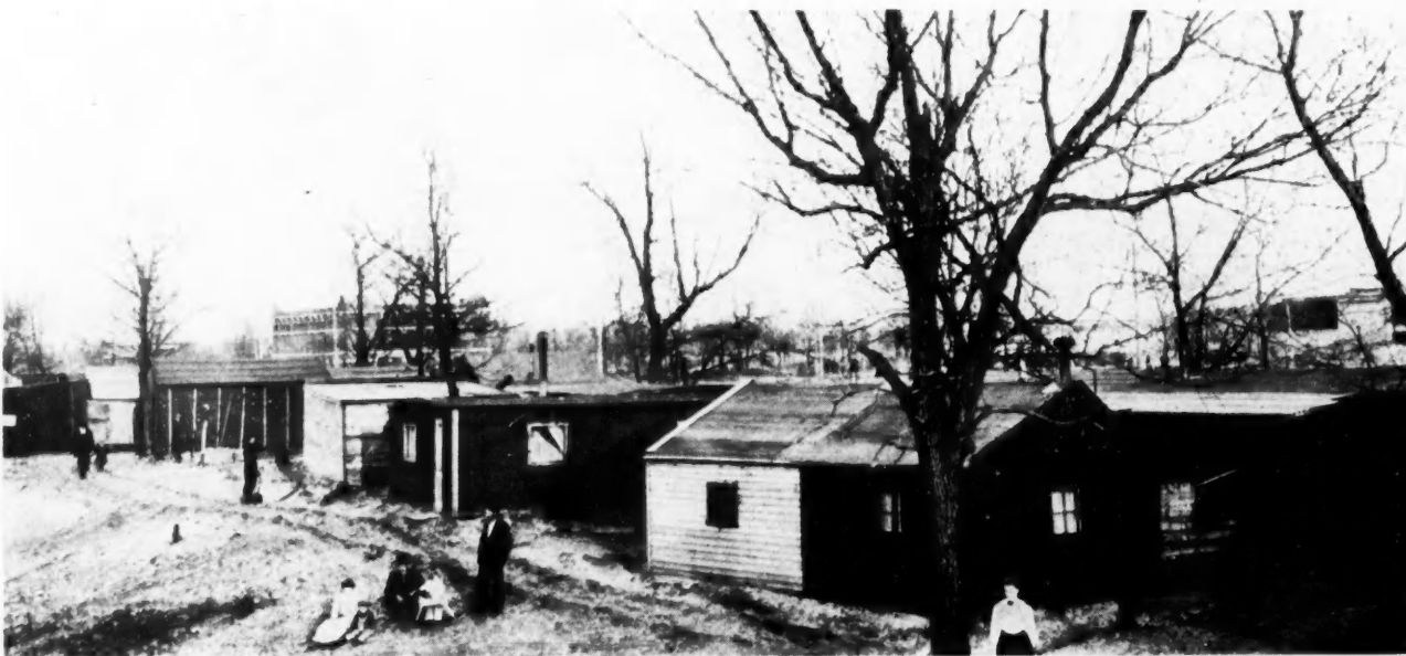
The Temporary Shacks Have Been Replaced by Modern Residences
