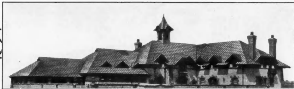
ASBESTOS "CENTURY" SHINGLE ROOF—ESTATE OF SENATOR T. M. DAVIS, NEWPORT, R. I.
