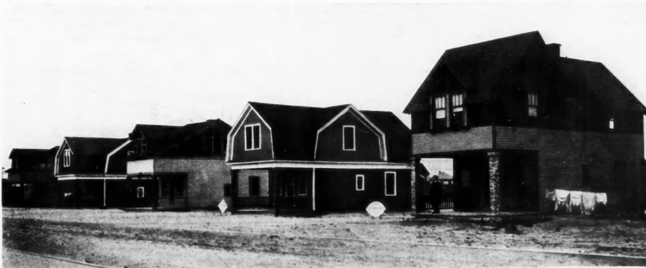
Group No. 3. A Comfortable Roomy Design—Variety of Roof Treatment Prevents Monotony
