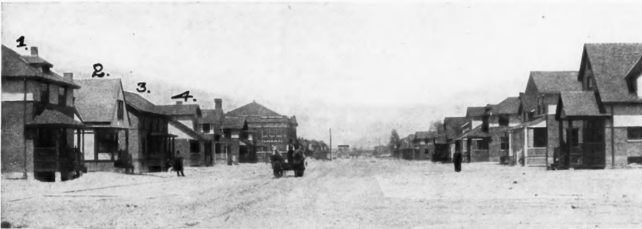
Group No. 1, Attractive and Substantial Six and Eight Room Houses, No Two Alike
