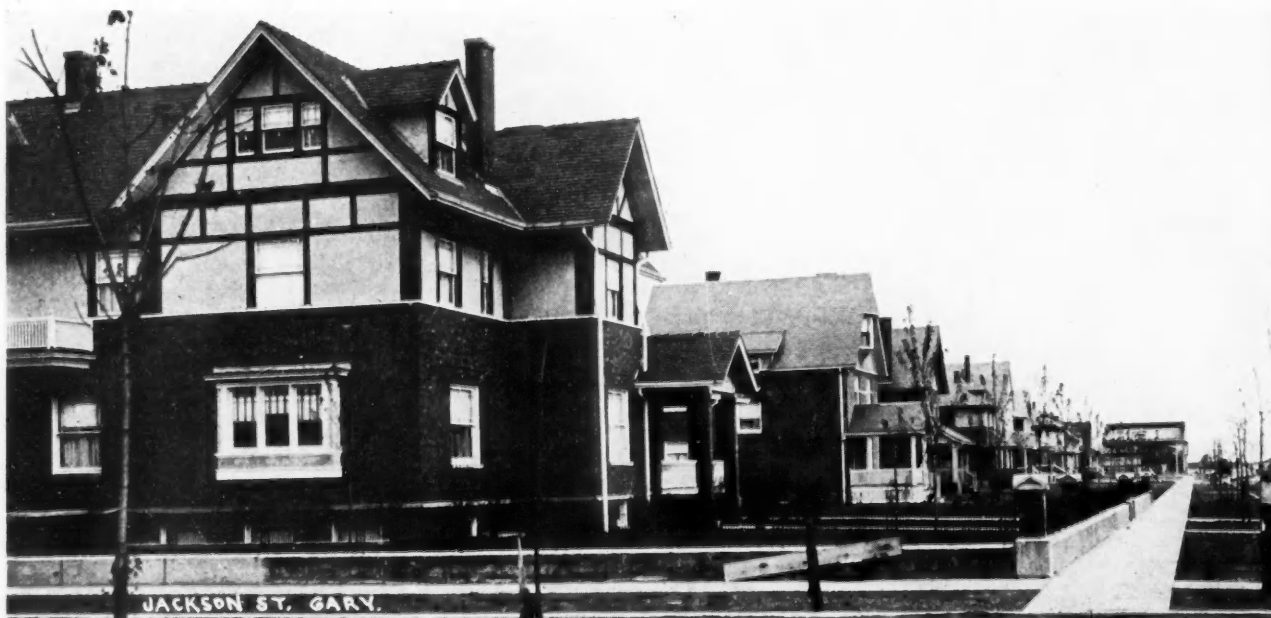
Brick, Cement Plaster, Timber and Tile Enter into the Exterior Construction of the Houses
