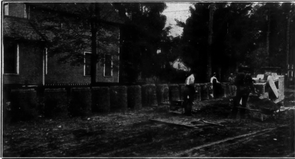
CUT OF COLTRIN NO. 6 MIXER WORKING ON REINFORCED SEWER PIPE
