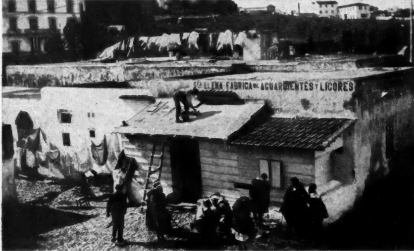
Laying a Concrete Roof
