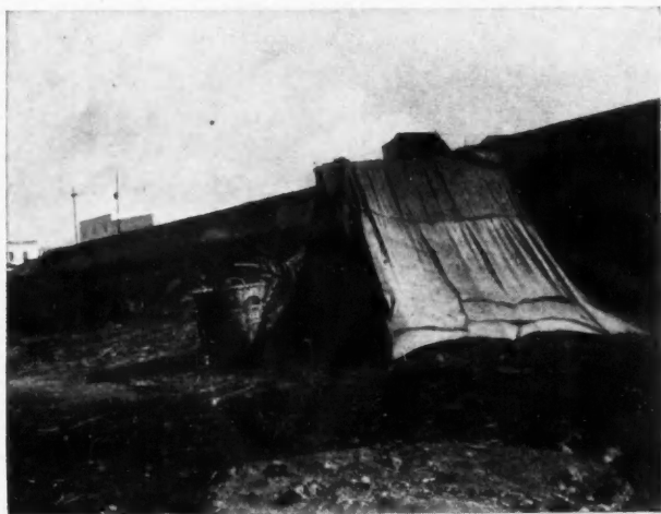
Plenty of Ventilation
