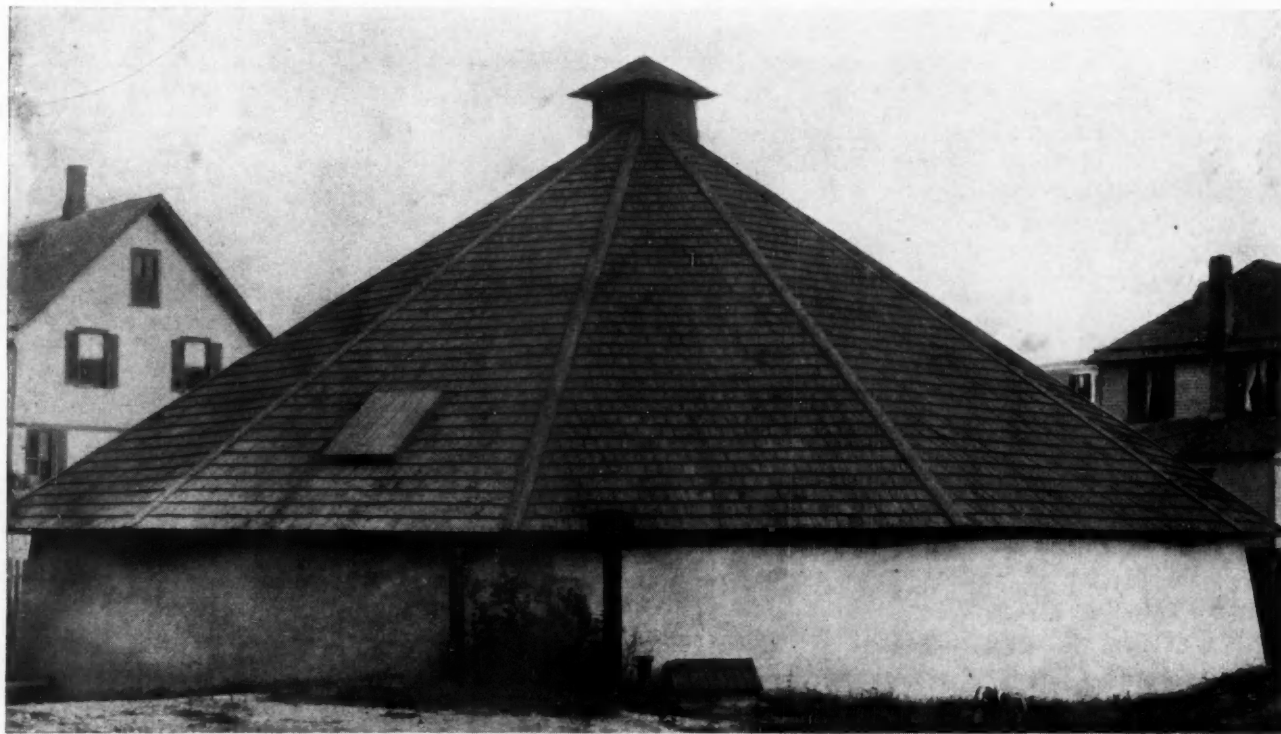
A Concrete Reservoir
