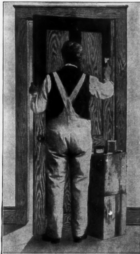
Removing with putty knife old finish softened with Solvo.
