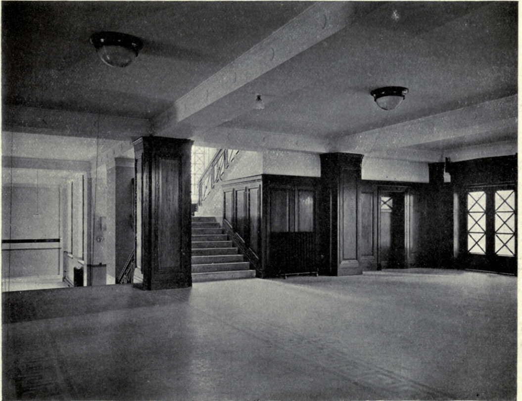
New Technical Institute, Cathays Park, Cardiff.
