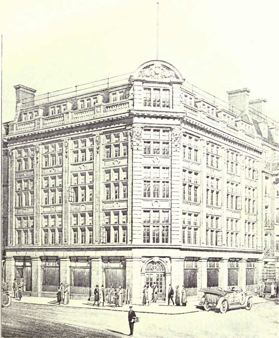
Business Premises, Gt. Portland Street, W.. H. O. CRESSWELL, Architect.
