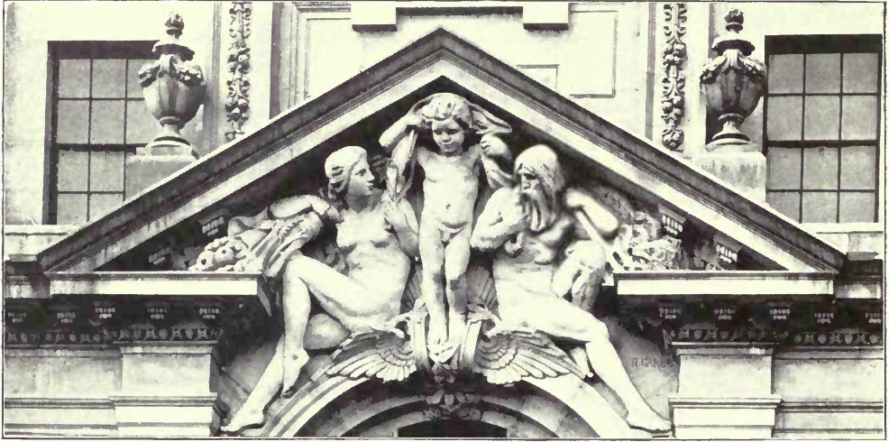
Detail to Entrance, Leibig House R. GARBE, Sculptor.
