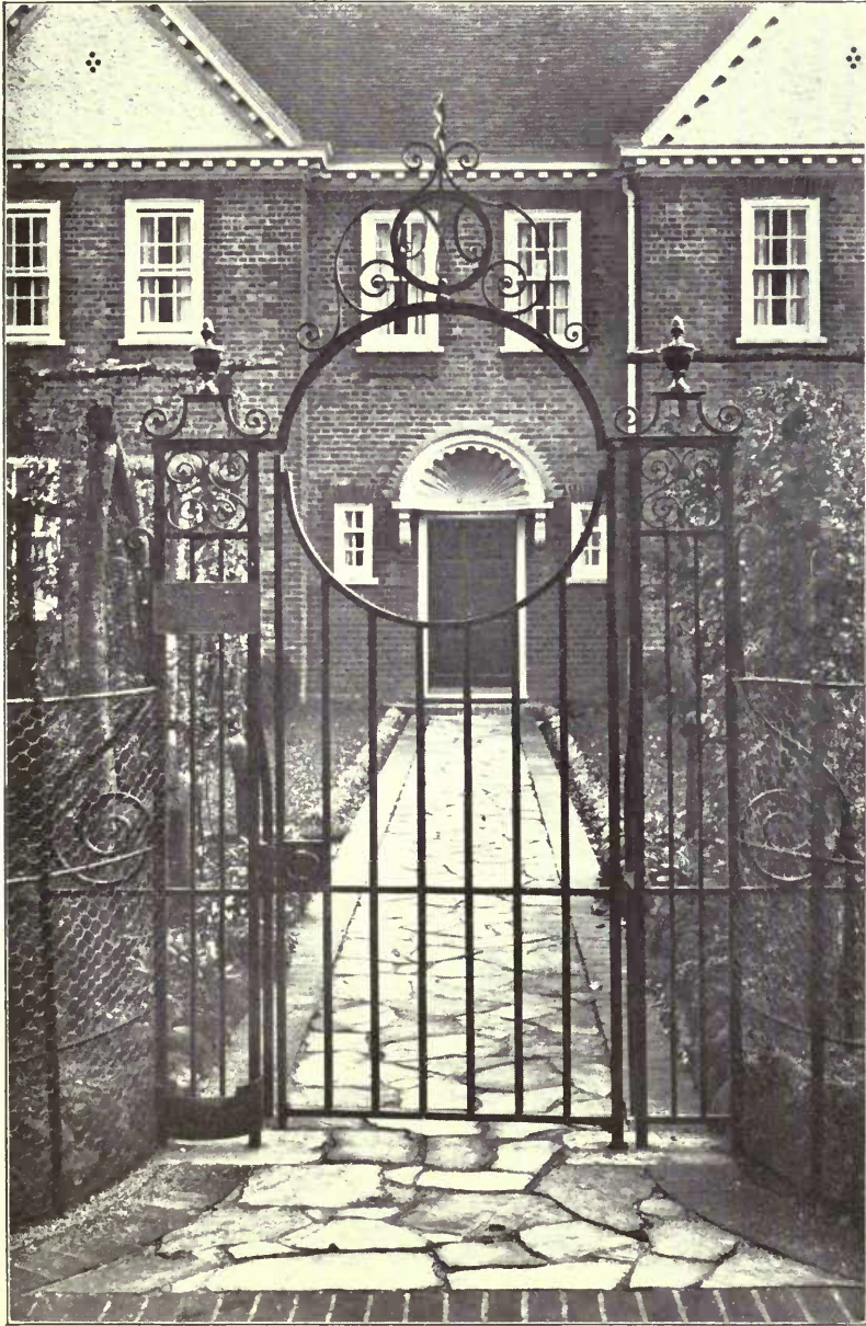
Queen Anne Cottage, Purley, Surrey, SYDNEY J. TATCHELL, Architect. Contractor: J. T. DEAKINS, 15, Blenheim Gardens, Wallington, Surrey.
