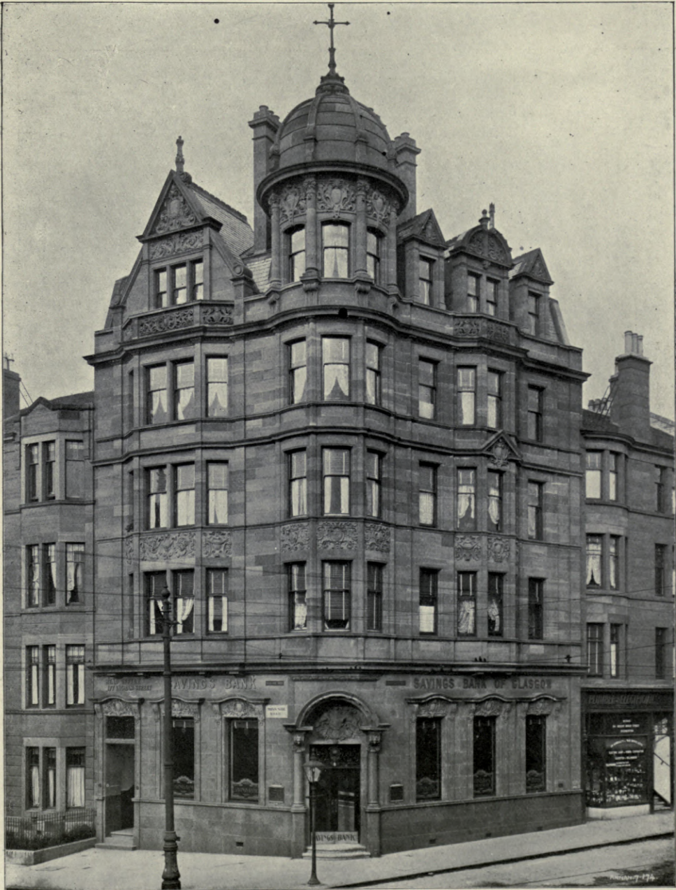
400. Glasgow Savings Bank, Shawlands Cross, NEIL C. DUFF, Architect. Mason Work; Geo. Barlas and Co., Ruthven Street, Glasgow.
