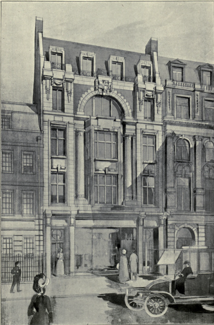
1714. No. 28 Margaret Street, W., JOHN BELCHER, A.R.A., Architect. Contractors: G. Godson and Sons, Pembroke Works, Kilburn Lane, W. Steelwork: G. Aston and Sons, Limited, 46 Eagle Wharf Road, N. Stone Carving: E. J. and A. T. Bradford, 62A Borough Road, S.E. (Tel. 2384 Hop.)
