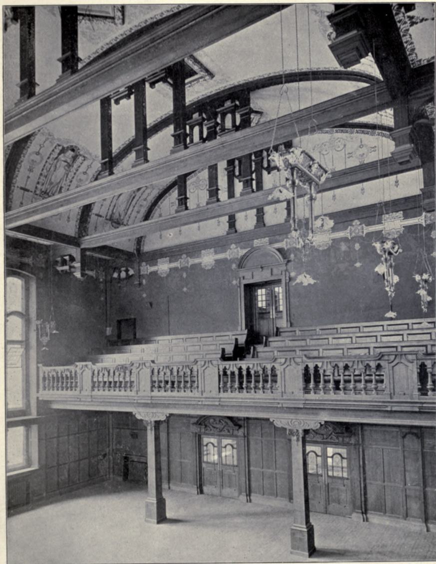
1455. Armstrong College, Great Hall, W. H. KNOWLES, Architect. Decoration, Handicraft Co., Vine Lane, Newcastle-on-Tyne.
