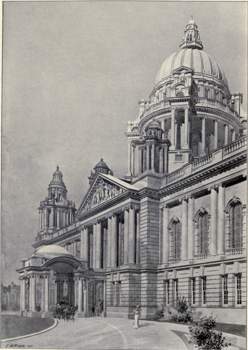
1512. The City Hall, Belfast, SIR BRUMWELL THOMAS, Architect. Contractors, H. and J. Martin, Ltd., Belfast. Heating, Ashwell and Nisbet, Ltd., 12 Great James' Street, Bedford Row, W.C.
