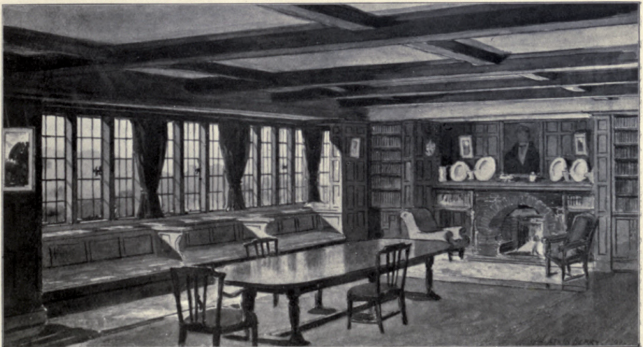
1635. Dining-room, House at Hailsham, W. H. ATKIN BERRY, Architect. Contractor, P. Hide, Hailsham.
