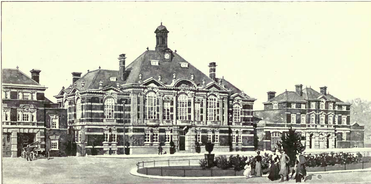
1611. Tottenham Municipal Buildings, A. S. TAYLOR AND A. R. JEMMETT, Architects. General Contractors: Walter Lawrence and Son, Waltham Cross and Tottenham. Devonshire Marble and Hopton-Wood Stone Staircases: H. T. Jenkins and Son, The Marble Works, Torquay. Electric Wiring and Telephones: Leo Sunderland and Co., 39 Victoria Street, S.W.
