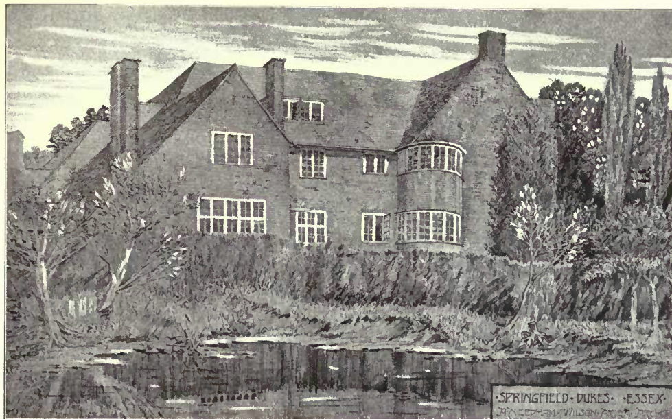
1586. Springfield Dukes, Essex , A. NEEDHAM WILSON, Architect. General Contractor: Frank Johnson, Chelmsford.
