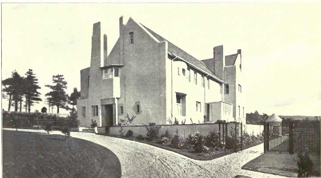
331. The Hill House, Helensburgh, HONEYMAN, KEPPIE AND MACKINTOSH, Architects.
