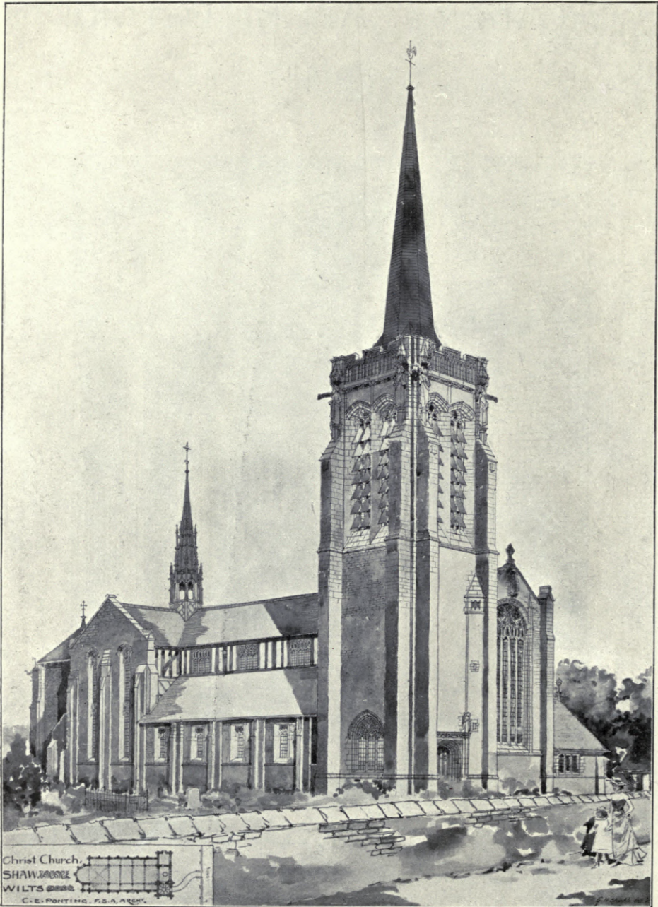
Christ Church, Shaw, Wilts., CHARLES E. PONTING, Architect. General Contractors: Hoskings Bros., Newbury, Berks.
