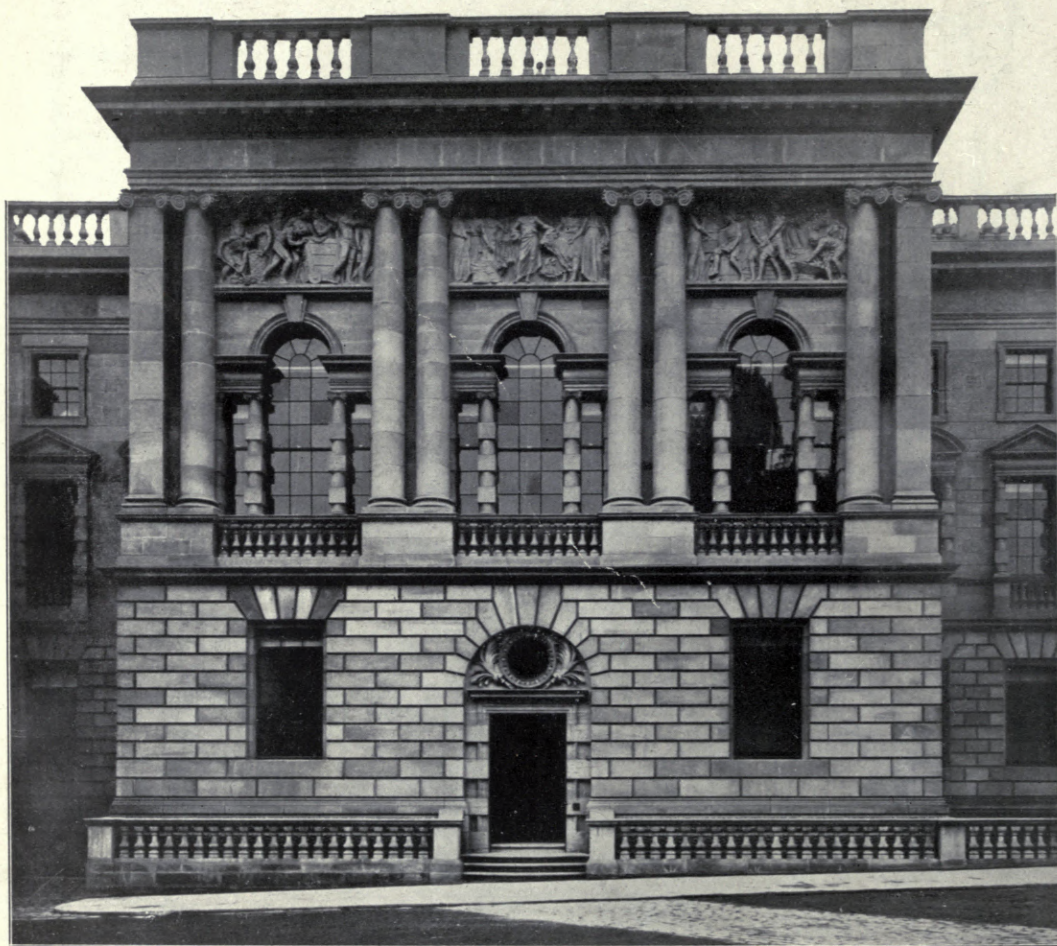
478. Midlothian County Buildings, Edinburgh , JAMES MACINTYRE HENRY, Architect. (For Plans, see Vol. 17, p. 84.)
