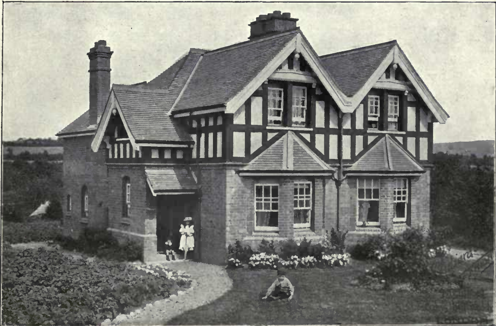
Cottages, "Southerton," Ottery St. Mary, Devon, T. E. LIDIARD JAMES, Architect.
