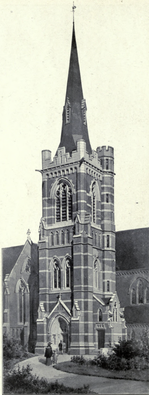
1478. Tower, Church of the Ascension, Balham Hill, T. E. LIDIARD JAMES, Architect.
